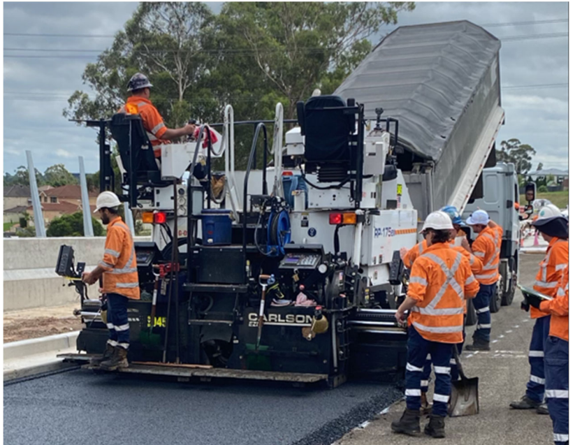
Laying permanent asphalt near the new pedestrian underpass.
