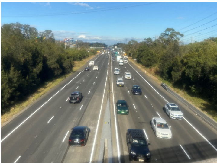
M4 speed restriction was lifted, returning to 100km/h in time for the holiday season.
