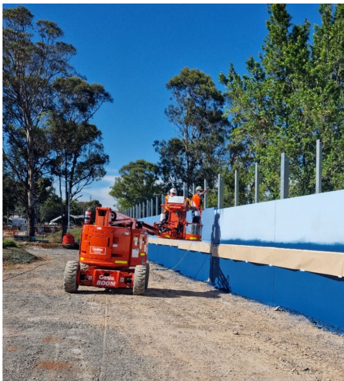
Painting underway at the noise wall near Lancelot Street.
