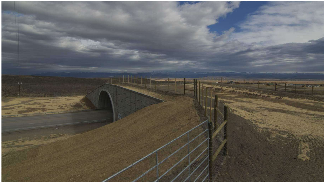
Wildlife bridge at Trappers Point, USA (photo: National Geographic)
