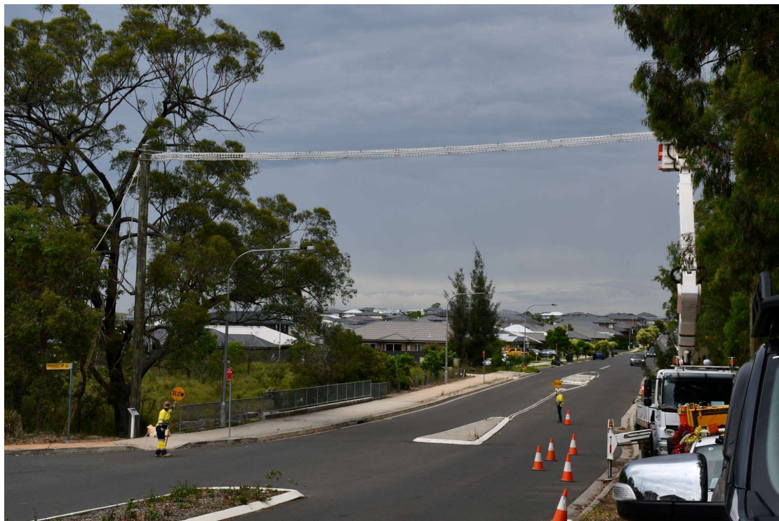
Wildlife ladder crossing erected in Glenmore Park
