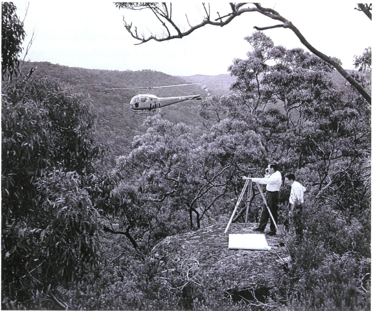
Preliminary road location work on the Sydney-Newcastle Freeway in the mid-1960s: surveyors at work in rugged terrain being aided by the DMR's first helicopter
