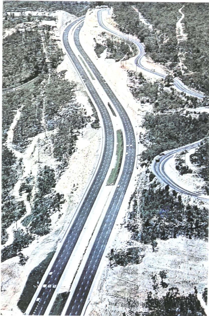
Curvilinear alignment of Sydney-Newcastle Freeway, with winding Pacific Highway on right
