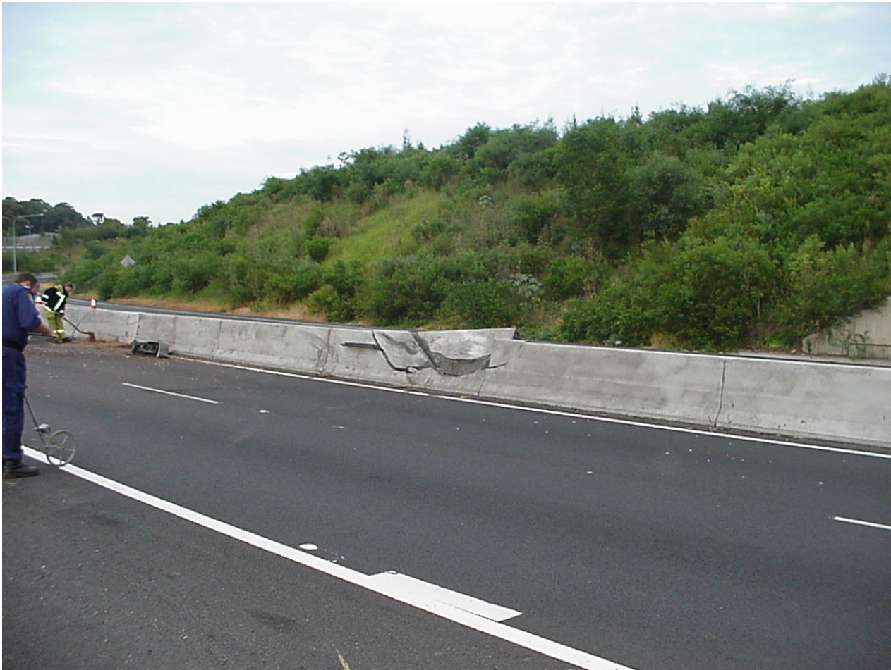
New Jersey barrier
