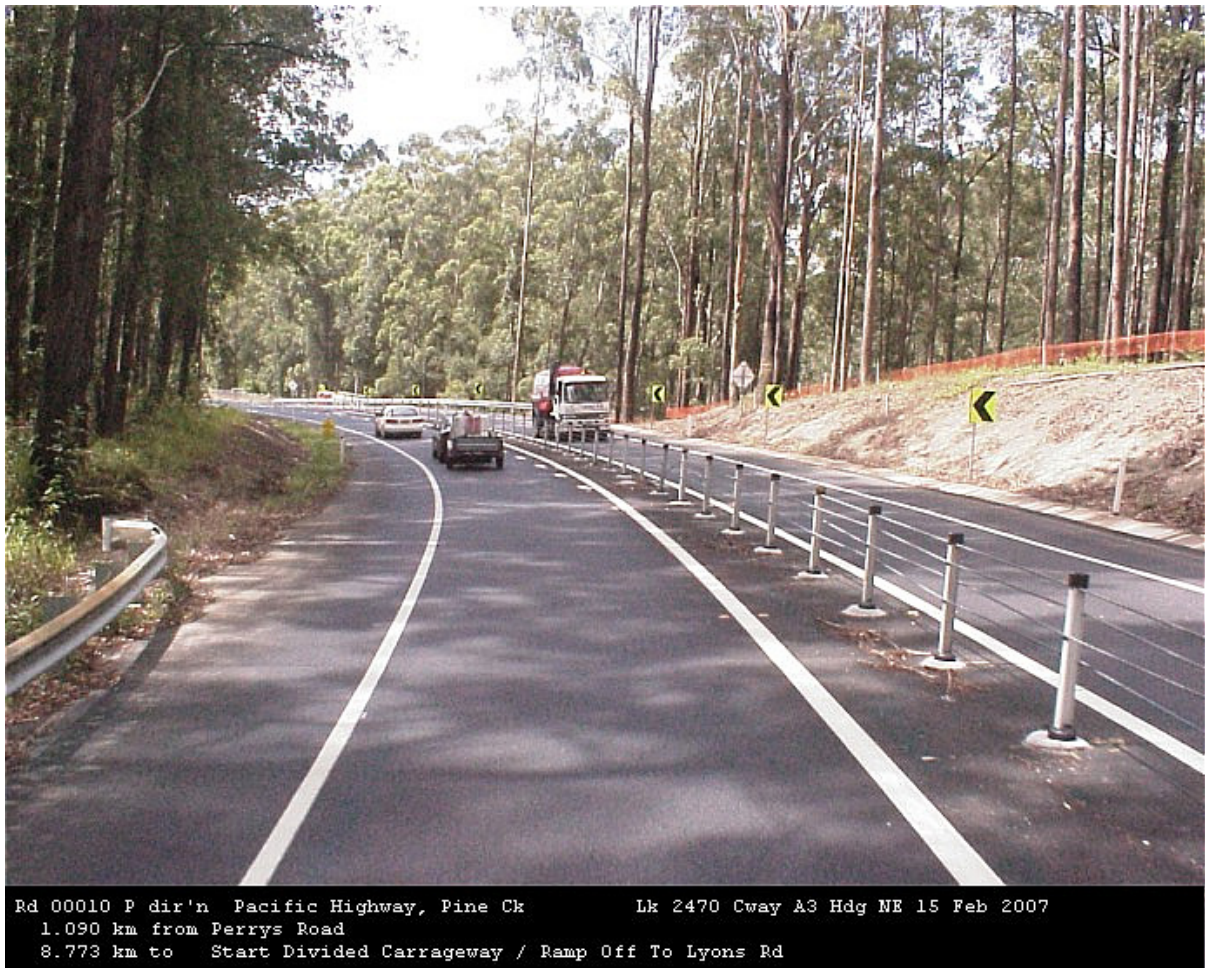
Wire rope median safety barrier on Pacific Highway
