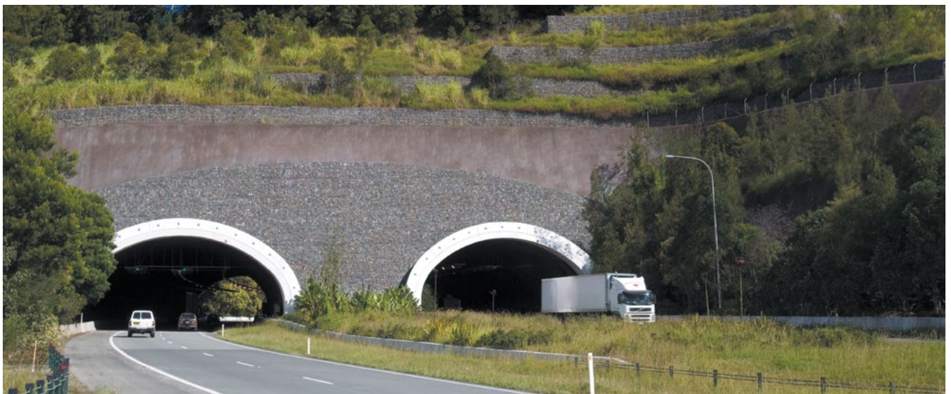
The Pacific Highway Cudgen Road tunnel allows the wooded ridge line and wildlife corridor to cross the road and extend down to the edge of the Tweed River. Native planting and seeding is provided to revegetate the edges of the portal. Use of gabion facing is suitable for the natural context.
