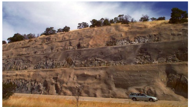
Shotcrete applications extend neatly to the edge of a change in the rock surface and coloured to match existing rock can look quite unobtrusive and visually acceptable. (Southern Freeway M1.)
