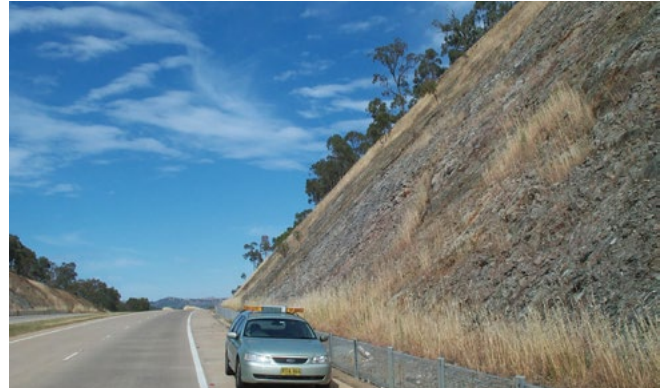
Untreated cutting on Hume Highway.
