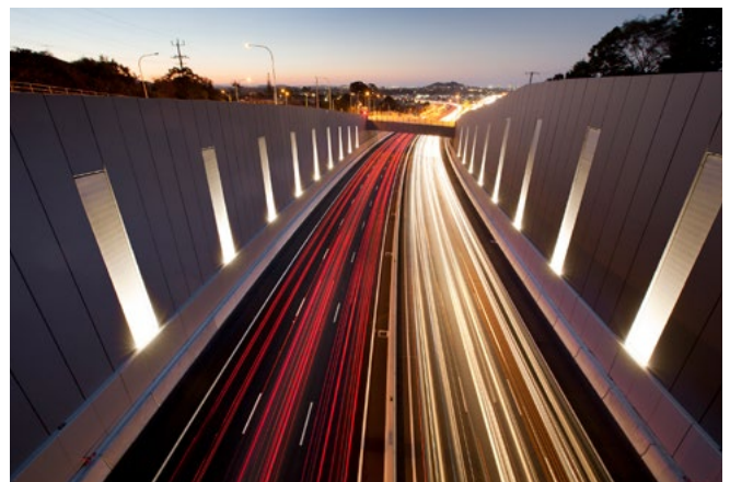
Concrete panel covering pile retaining wall and shotcrete on the Pacific Highway at Banora Point.
