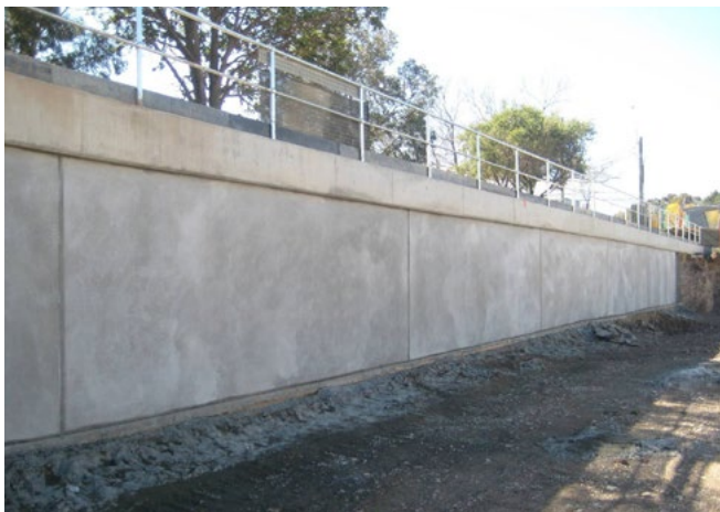
A formal element in the landscape can be more acceptable than a formless finish such as untreated shotcrete.
