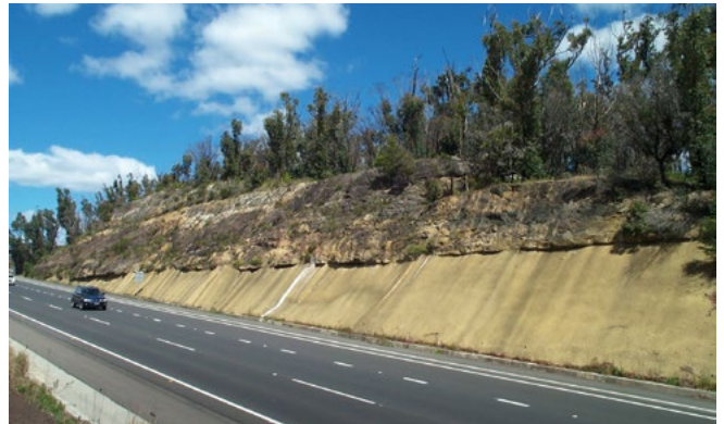
Shotcrete applications extend neatly to the edge of a change in the rock surface and coloured to match existing rock can look quite unobtrusive and visually acceptable. (Southern Freeway M1.)
