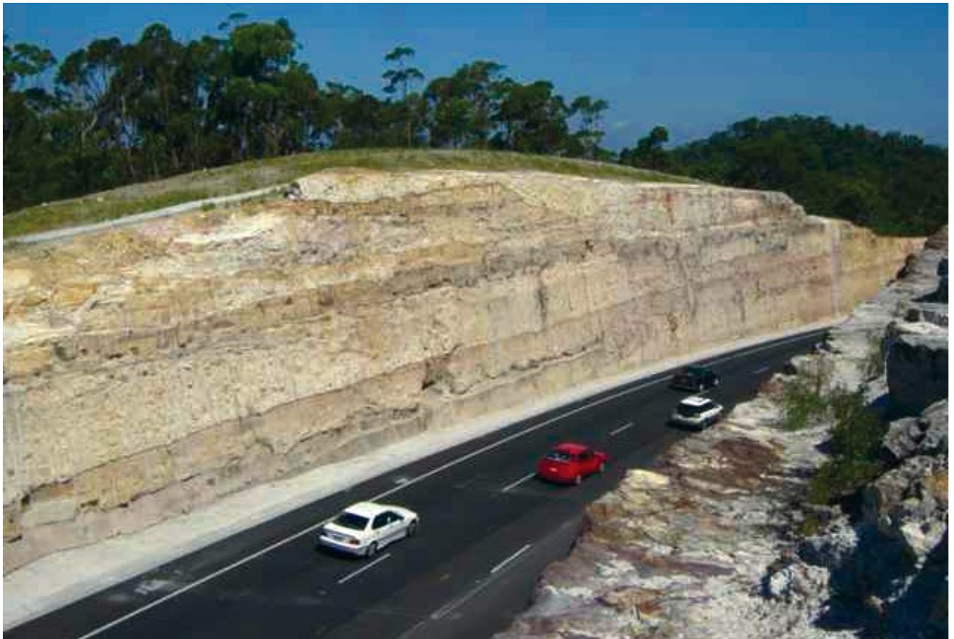
Shotcrete application carefully minimised on the M1 north of Sydney. Image: Spackman Mossop
