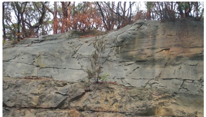
A rock type finish on the southern approaches to the Spit Bridge, Sydney is quite unobtrusive and effective.
