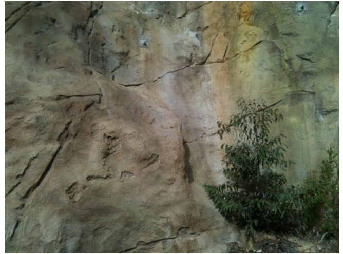
Rock sculpting and painting can help blend the shotcrete with the rock, but care must be taken that it does not appear artificial.
