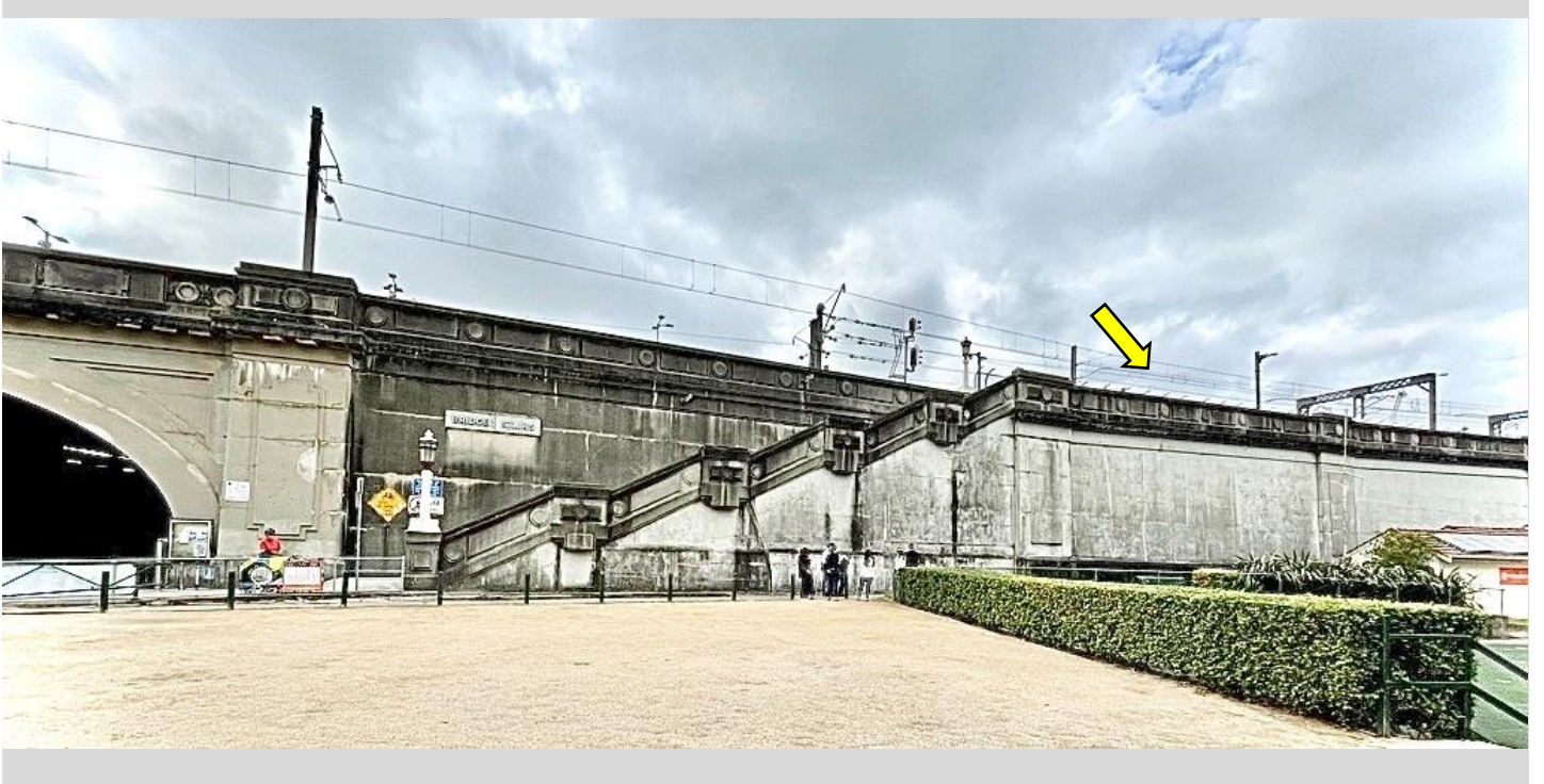
Photo: Burton Street tunnel and Sydney Harbour Bridge access stairs.
