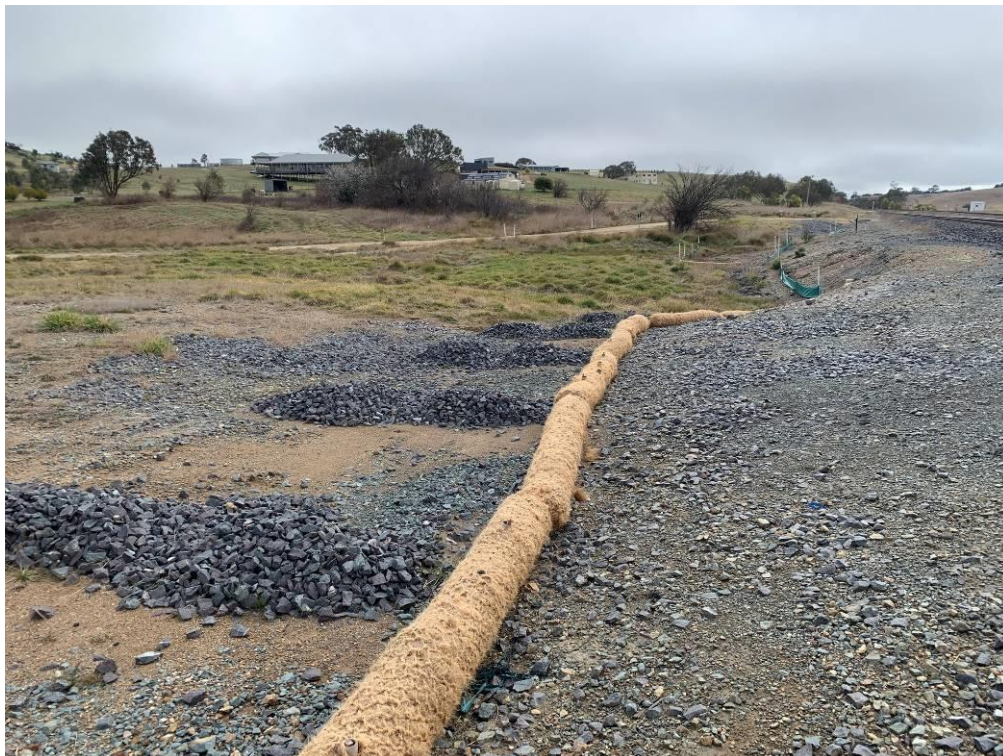
Photo 12: Rock checks running alongside former Woodlawn siding towards the middle culvert. Previous silt fencing with major damage replaced by Coir sediment control logs as recommended in previous inspections. No evidence of sediment build-up in rock armoury.
