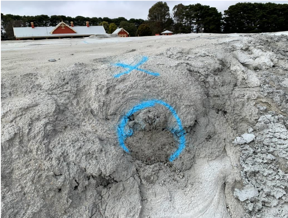
Photo 19: Exposed geofabric layer marker on main stockpile which was identified during the previous inspection (19/07/23), that has since been filled in with concrete.
