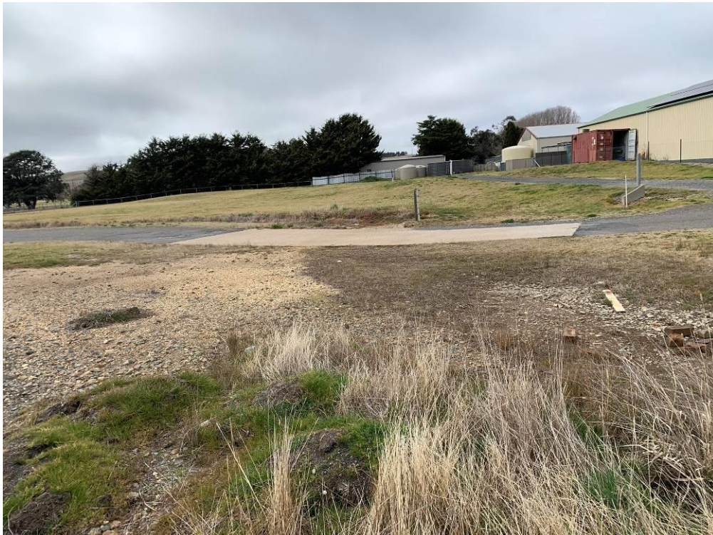
Photo 6: Causeway downgradient of middle culvert showing no evidence of current surface water moving off site. No visible sediment on road or vegetation nearby from sediment water was running off site in between inspections.
