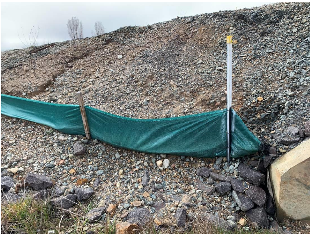
Photo 14: Upgradient of middle trainline culvert facing east. Silt fencing is clear with no sediment visible.
