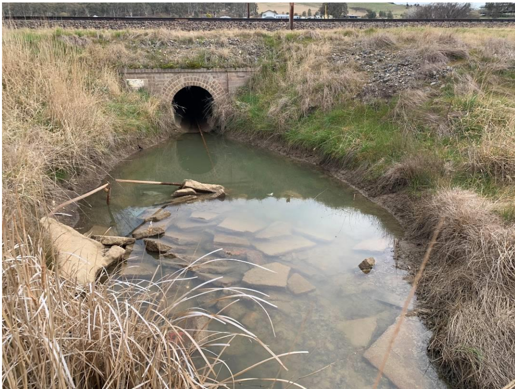
Photo 4: Downgradient of middle culvert showing mostly clear water on site. Majority of sediment has settled to the bottom of the water body. No surface water running off site at middle culvert.
