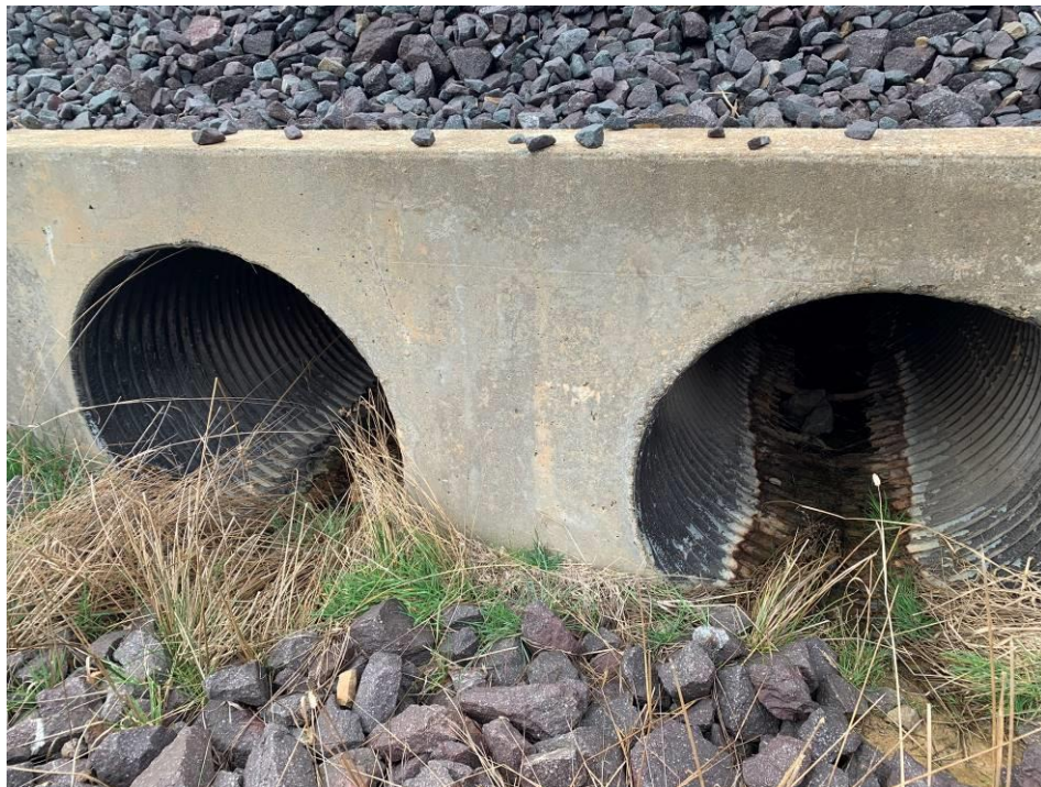
Photo 8: Upgradient of northernmost culvert showing evidence of no surface water surrounding.
