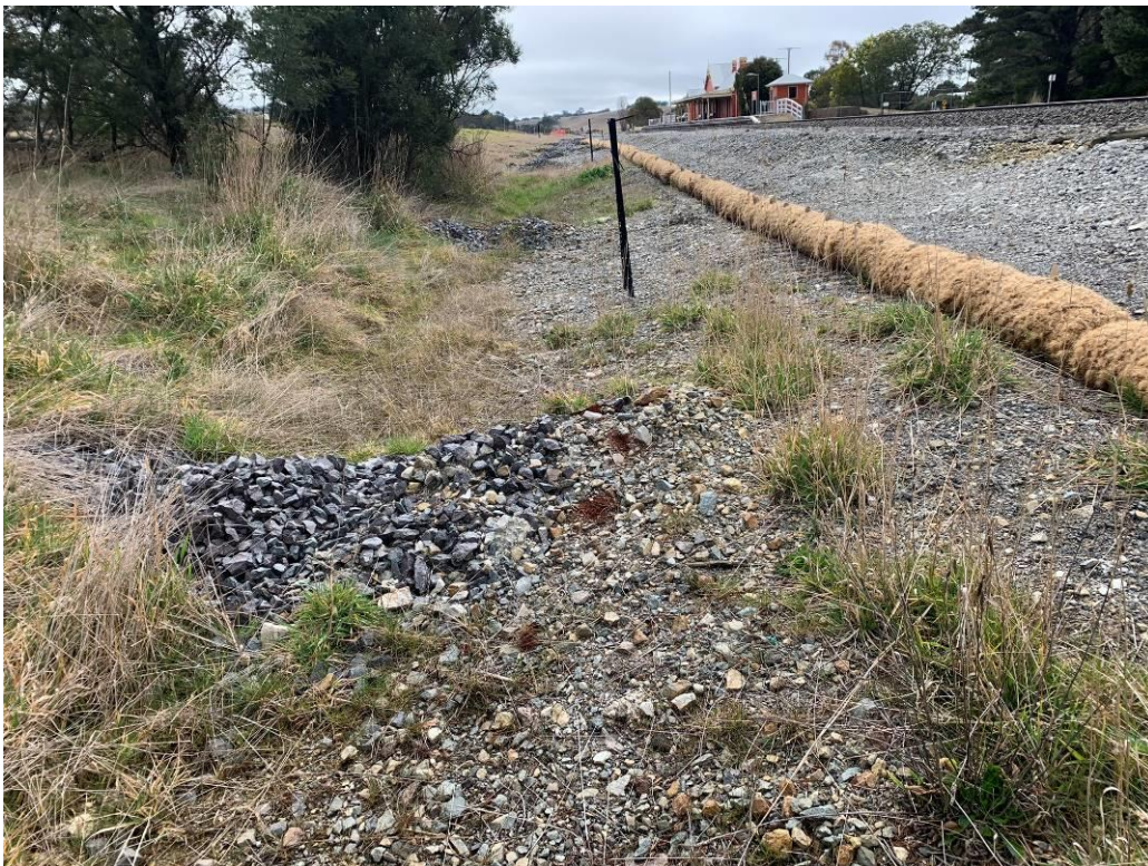
Photo 10: Upgradient of southernmost culvert showing previous silt fencing replaced by Coir sediment control logs, used as control measures for sediment control. Facing north-east.
