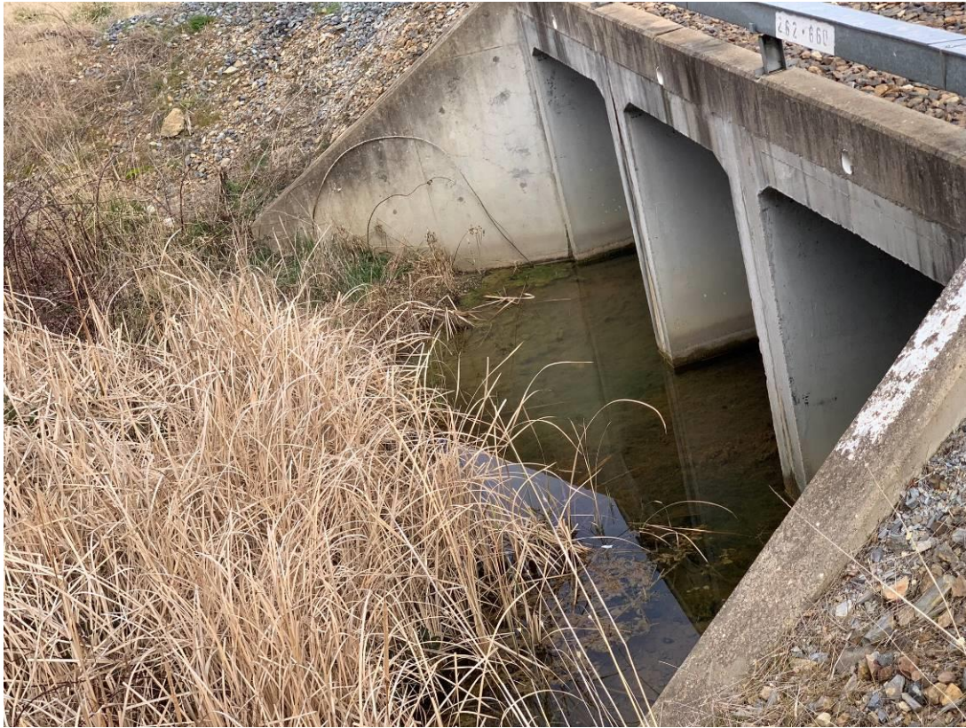
Photo 3: Southern most culvert downgradient of rail line, with slow moving surface water travelling off-site. Water is clear, low turbidity, minimal observable sediment, long grass and some algae present.
