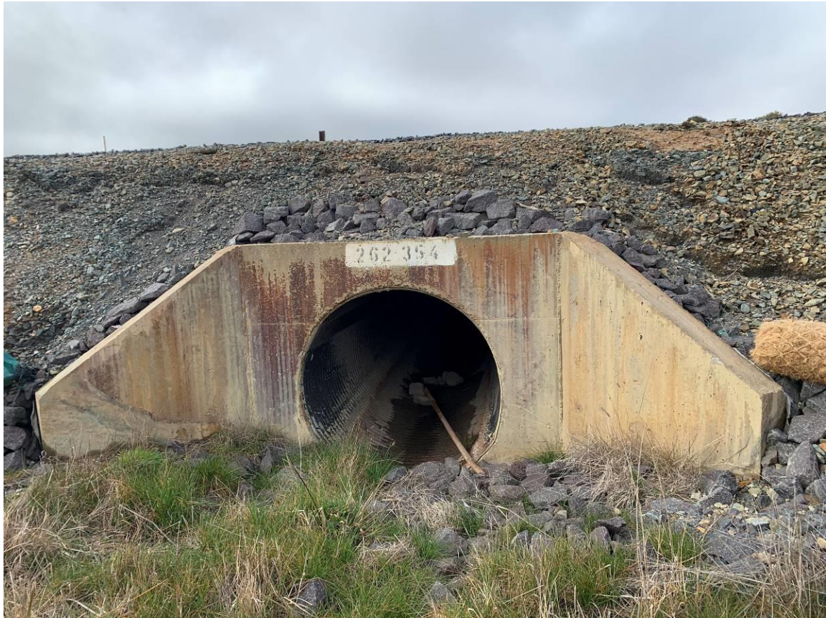
Photo 13: Middle culvert showing no flowing or pooled water. No evidence of sediment build-up in culvert.
