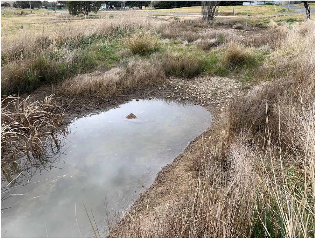
Photo 5: Downgradient of middle culvert. Dry beyond the pooled water and no evidence of current surface water run off on site.
