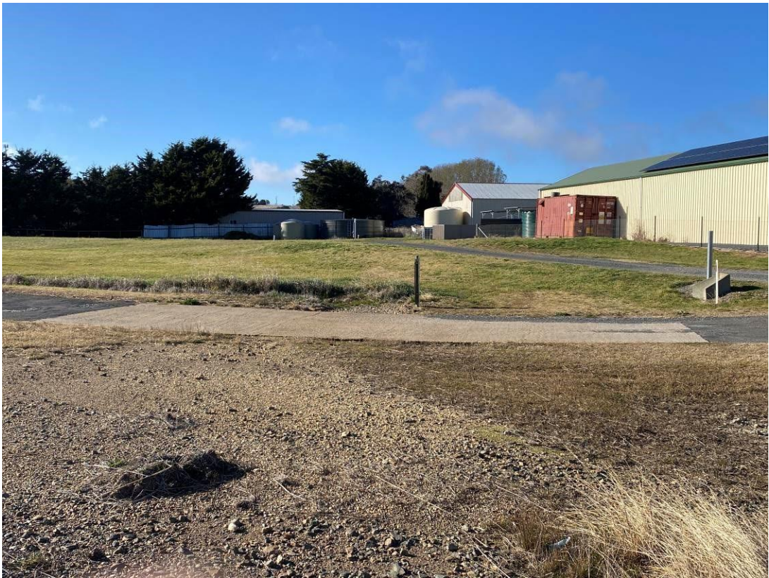
Photo 6: Causeway downgradient of middle culvert showing no evidence of current surface water run off on site. No visible sediment on road or vegetation nearby from sediment water was running off site in between inspections.
