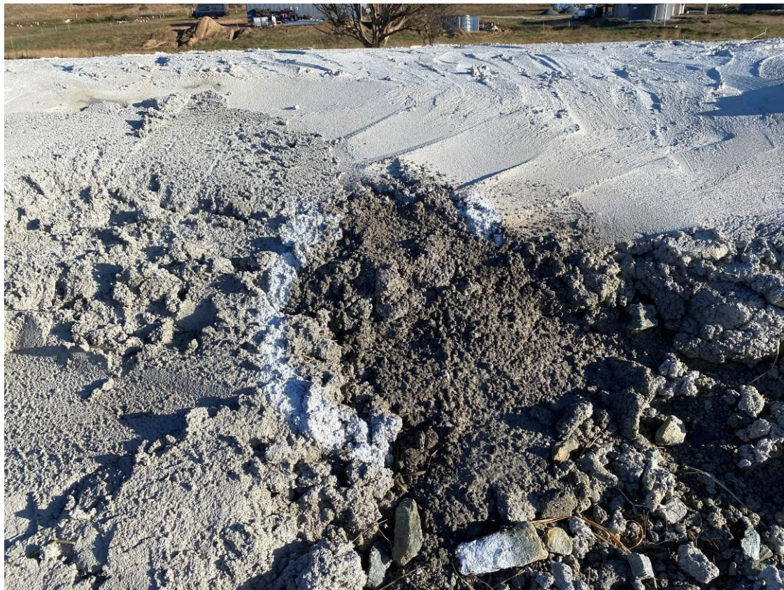
Photo 19: Geofabric marker layer visible in stockpile capping noted in previous inspection 20/04/23 had been patched as per recommendations.
