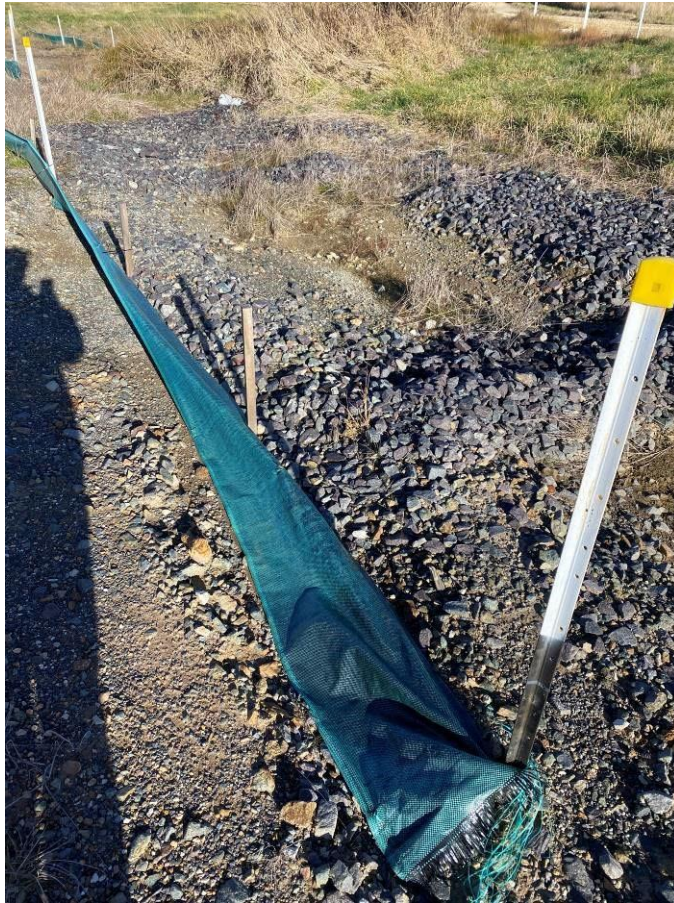
Photo 15: Silt fencing and rock armoury upgradient of trainline running from the middle to the north culvert. Silt fencing damaged and not attached to stakes.
