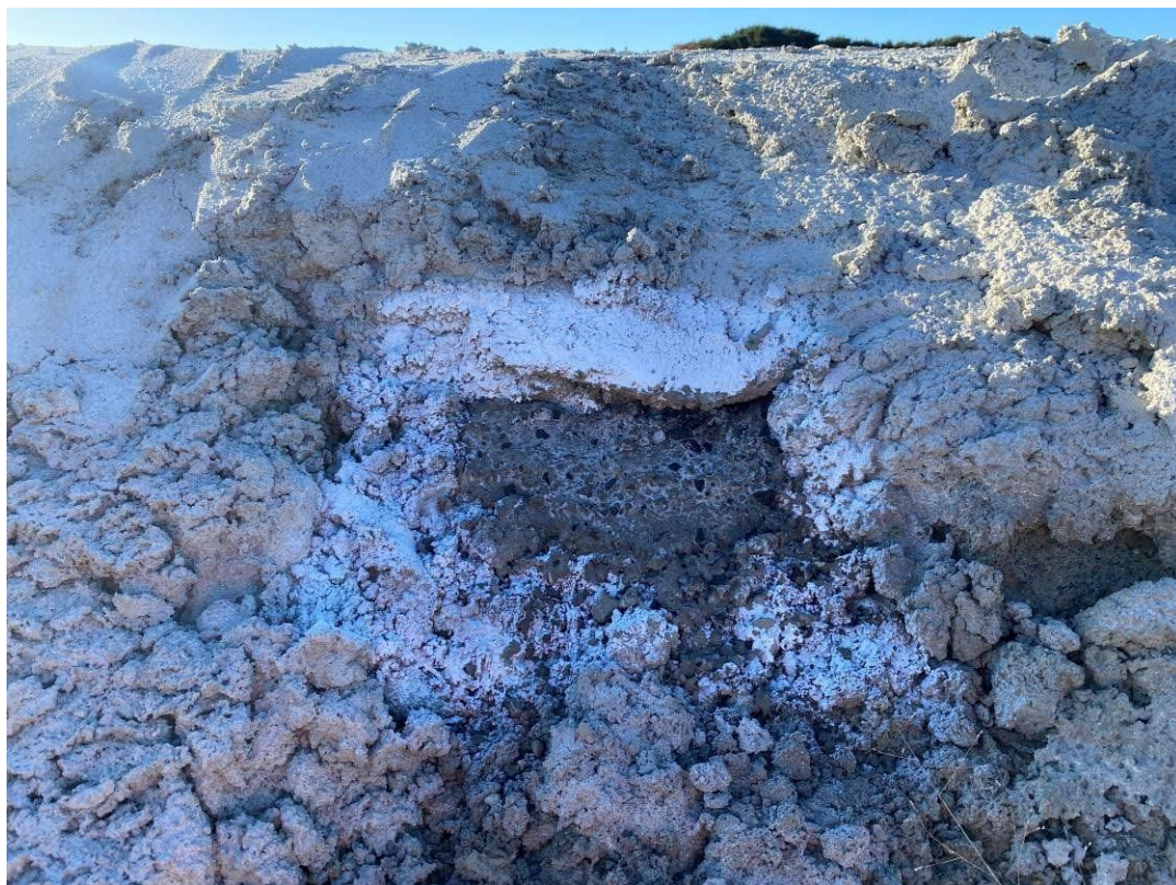
Photo 19: Geofabric marker layer visible in stockpile capping noted in previous inspection 20/04/23 had been patched as per recommendations.
