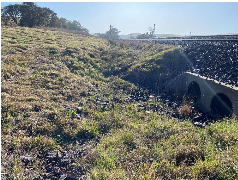
Photo 15: Silt fencing and rock armoury upgradient of trainline running from the middle to the north culvert. Silt fencing damaged and not attached to stakes.
