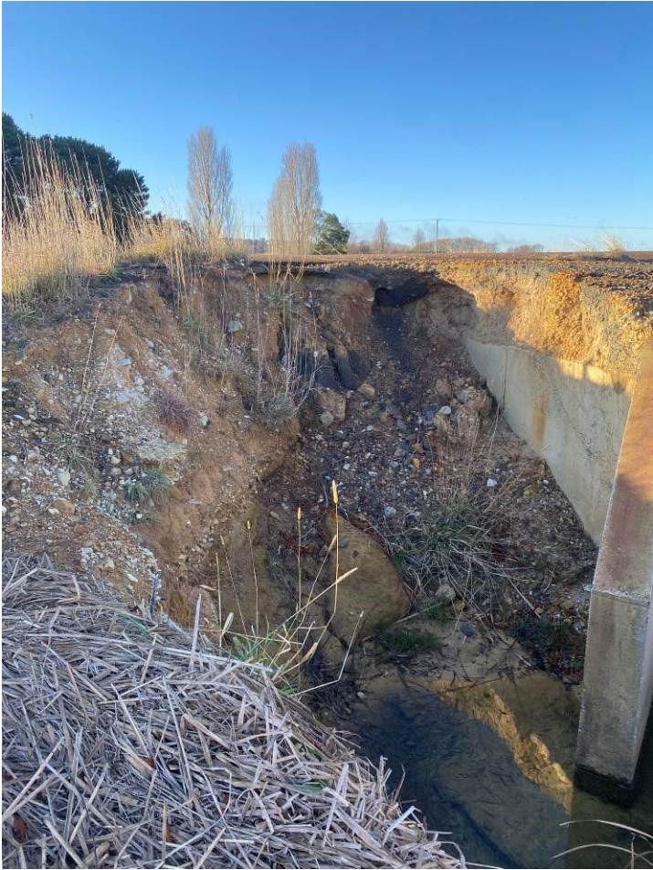
Photo 25. Notable erosion evident adjacent to the culvert further upgradient of the southernmost culvert. Surface water pooled near culvert and below erosion is clear with no visible signs of sediment. This erosion is not expected to impact surface water flowing off site.
