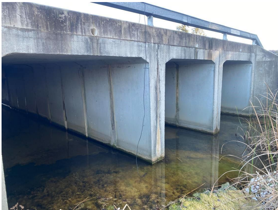
Photo 3: Southern most culvert downgradient of rail line, showing evidence of surface water run off on site. Water is clear, no turbidity, with no observable sediment, some algae present.
