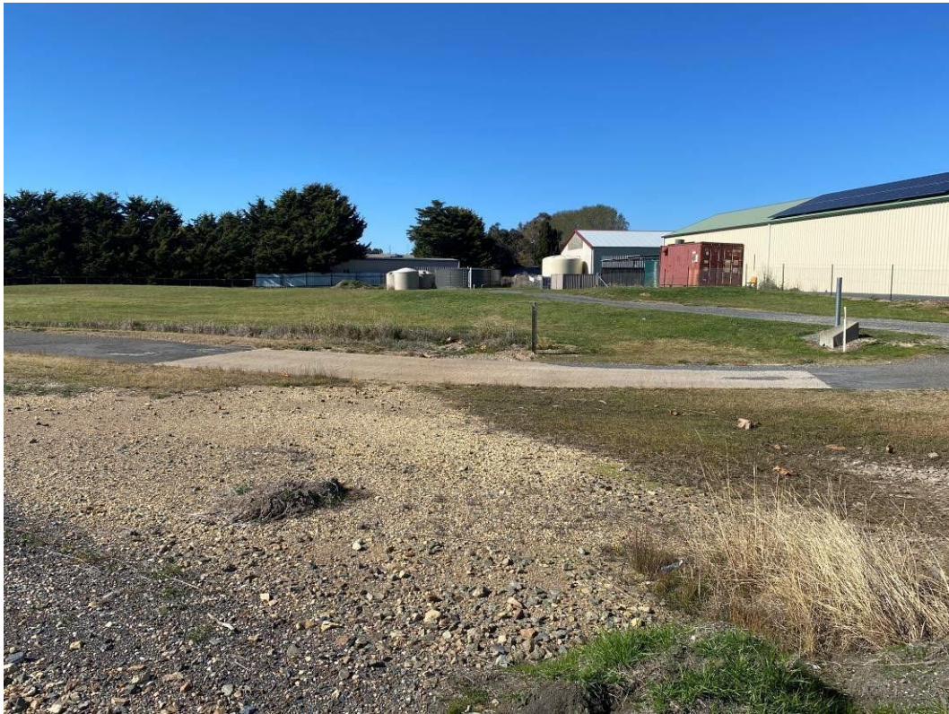
Photo 7: Causeway downgradient of middle culvert showing no evidence of current surface water run off on site. No visible sediment on road or vegetation nearby from sediment water was running off site in between inspections.
