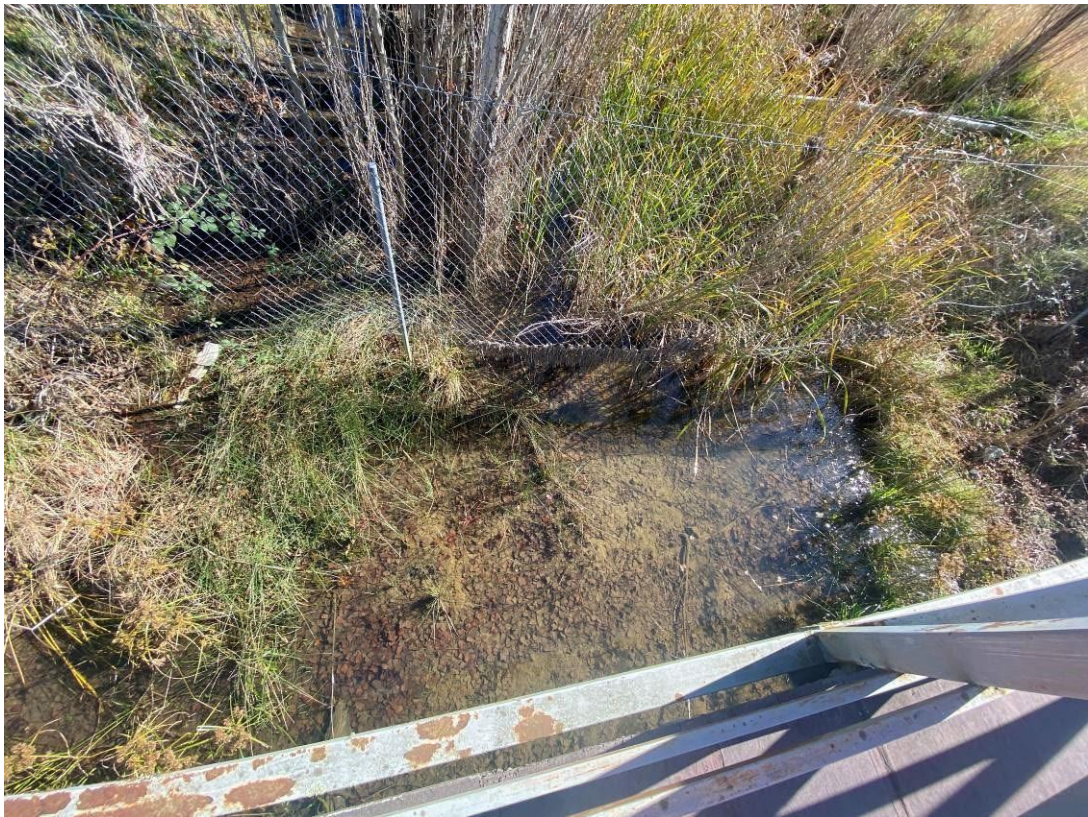
Photo 3: Southern most culvert discharge off site through culvert under Golburn street, showing evidence of surface water run off on site. Water is clear, no turbidity, with no observable sediment.
