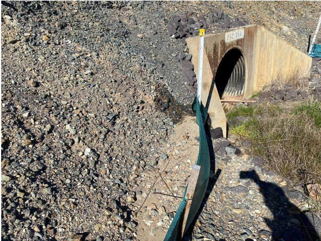
Photo 12: Upgradient of middle culvert showing signs of sediment in silt fencing on northern side. Silt fencing is full and sediment needs to be clear or fencing needs to be replaced before breakages.
