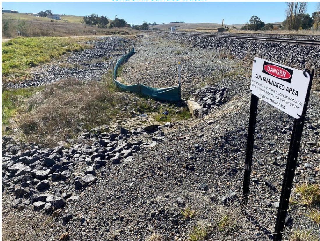
Photo 15: Upgradient of northernmost culvert. No evidence of surface water run off on site. No evidence of sediment buildup on rocks. Rock armory and natural vegetation allow for sediment control in surface water.
