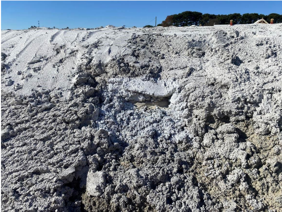
Photo 19. Geofabric marker layer visible in stockpile capping remained from previous inspection. Approximately 10cm x 2cm. UGL representative stated patching works will take place Friday 19 May 2023.
