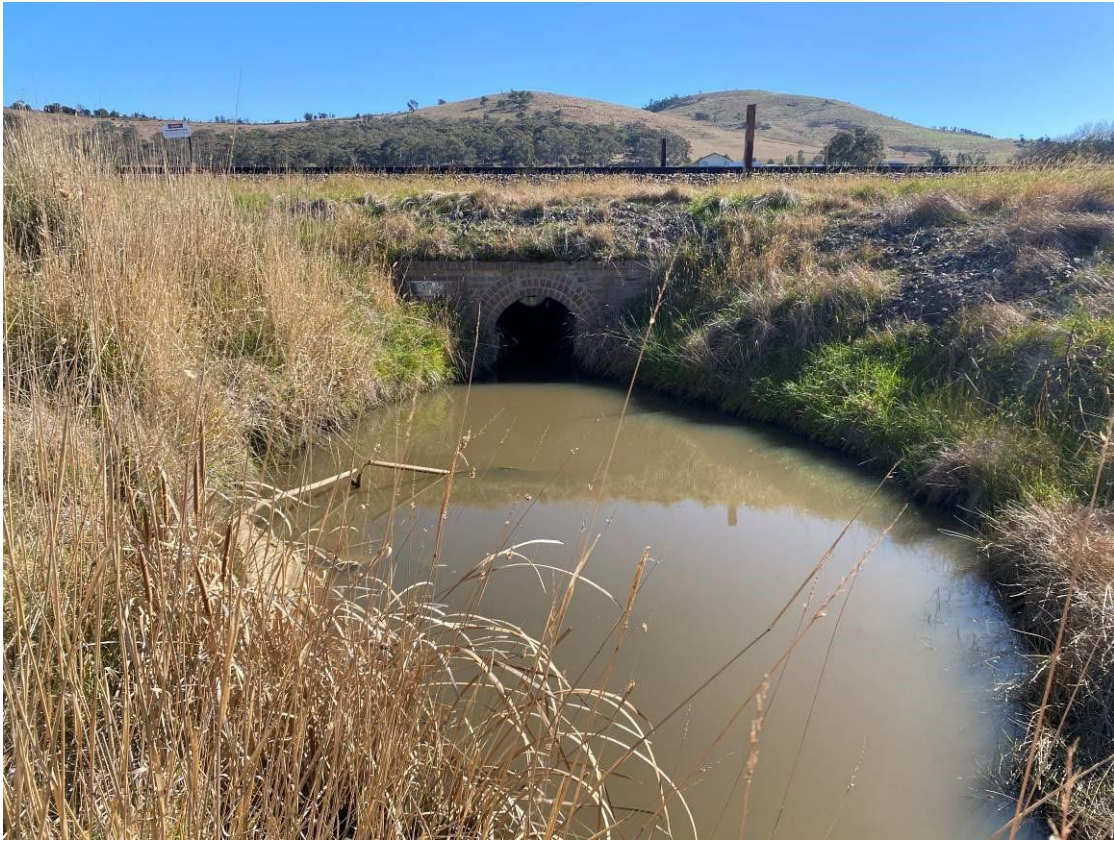
Photo 5: Downgradient of middle culvert showing pooled sediment laden water on site. Brown, moderate turbidity.
