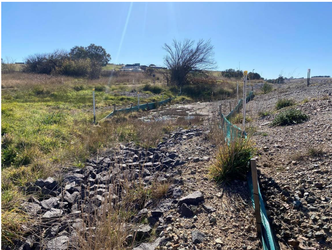
Photo 12: Upgradient of middle culvert showing signs of sediment in silt fencing on northern side. Silt fencing is full and sediment needs to be clear or fencing needs to be replaced before breakages.
