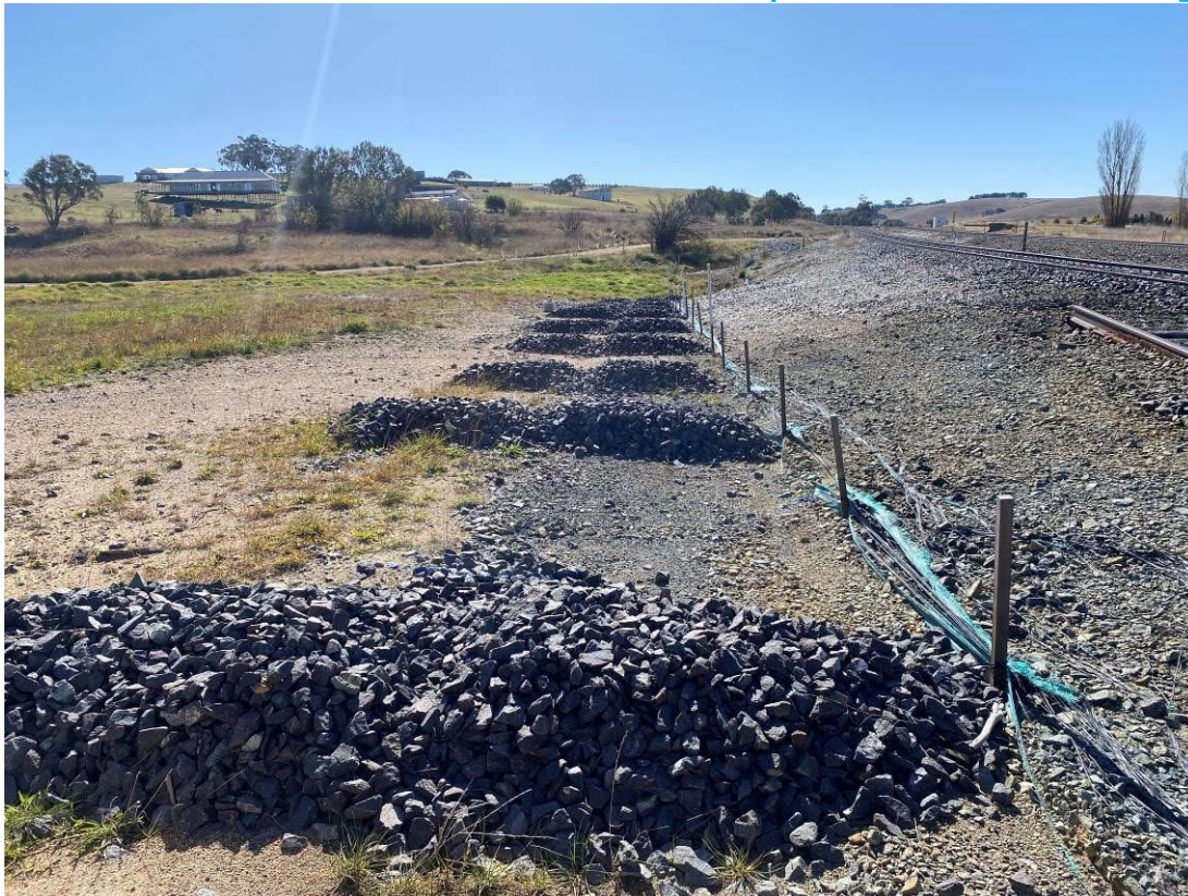
Photo 11: Rock checks and silt fences running alongside former Woodlawn siding towards the middle culvert. Major damage to silt fencing remaining on southern side. No evidence of sediment build-up in rock armoury.
