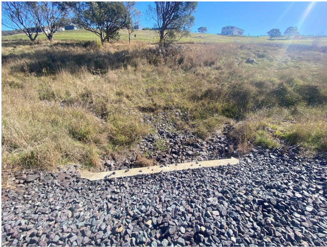
Photo 15: Upgradient of northernmost culvert. No evidence of surface water run off on site. No evidence of sediment buildup on rocks. Rock armory and natural vegetation allow for sediment control in surface water.
