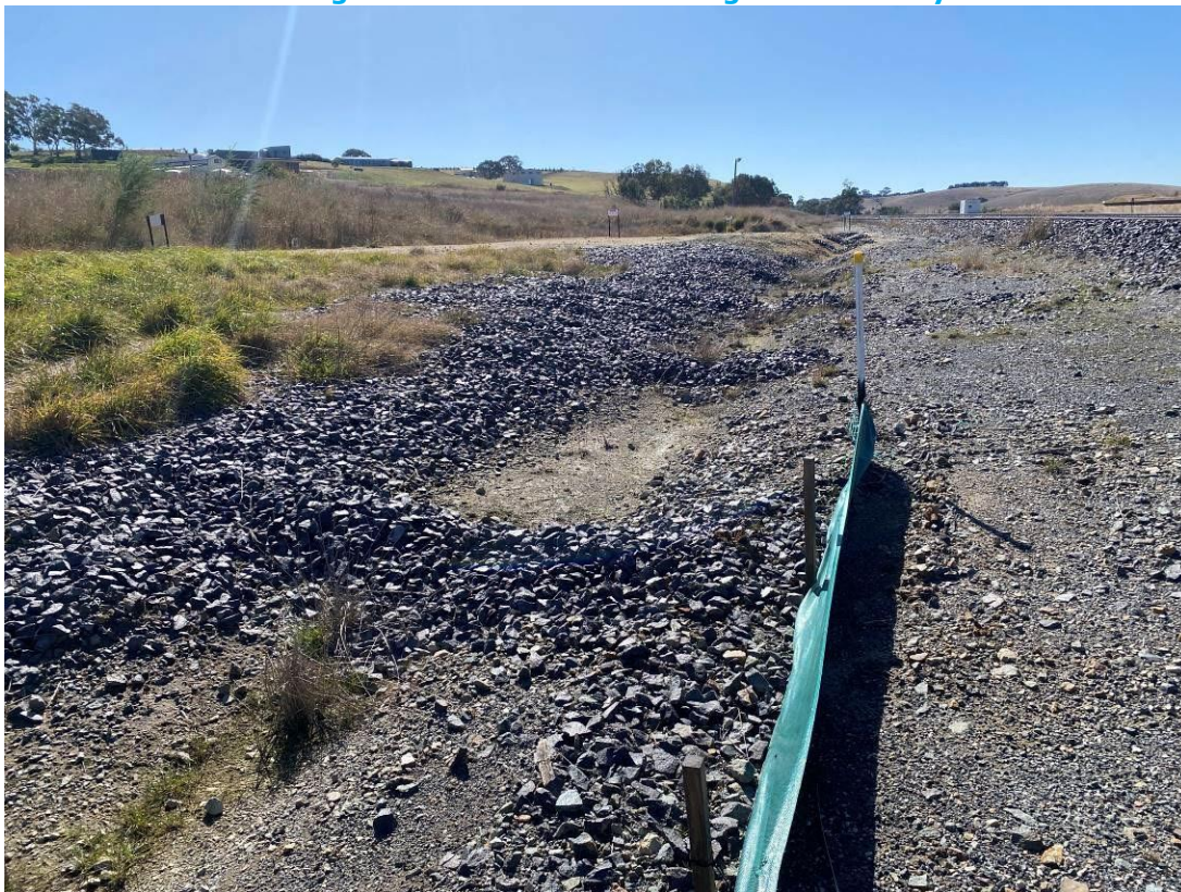
Photo 14: Silt fencing and rock armoury upgradient of trainline running from the middle to the north culvert. Some erosion evidence of soil and build-up of sediment on silt fencing and rock armoury.
