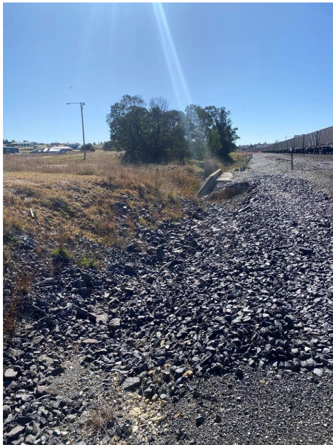
Photo 9: Upgradient of southernmost culvert showing silt fencing and rock armoury used as control measures for sediment control.
