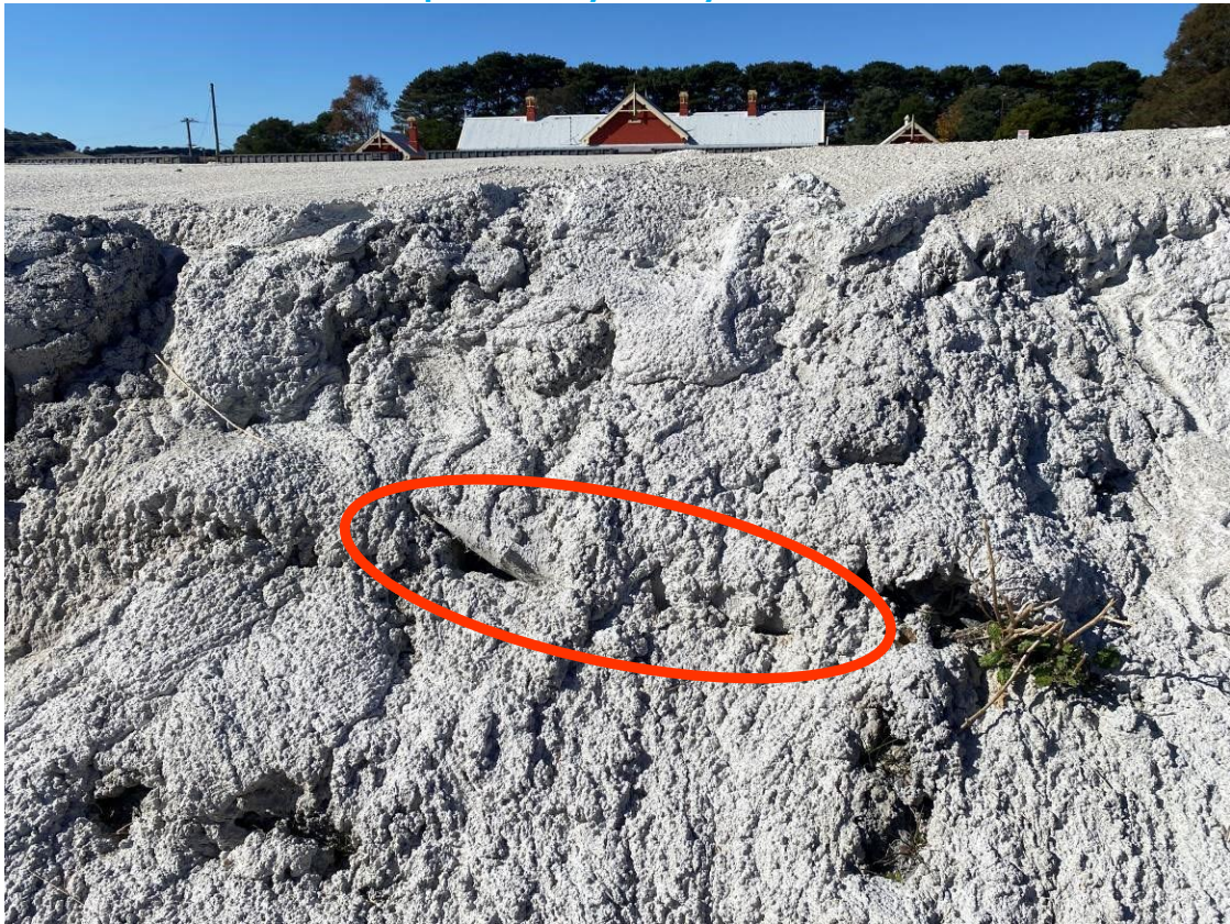
Photo 19. Geofabric marker layer visible in stockpile capping remained from previous inspection. Approximately 10cm x 2cm. UGL representative stated patching works will take place Friday 19 May 2023.
