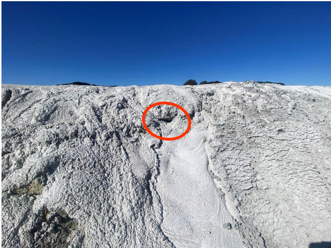
Photo 21. New location of geofabric marker layer visible in stockpile capping UGL on site representative was notified. Approximately 5cm x 3cm.
