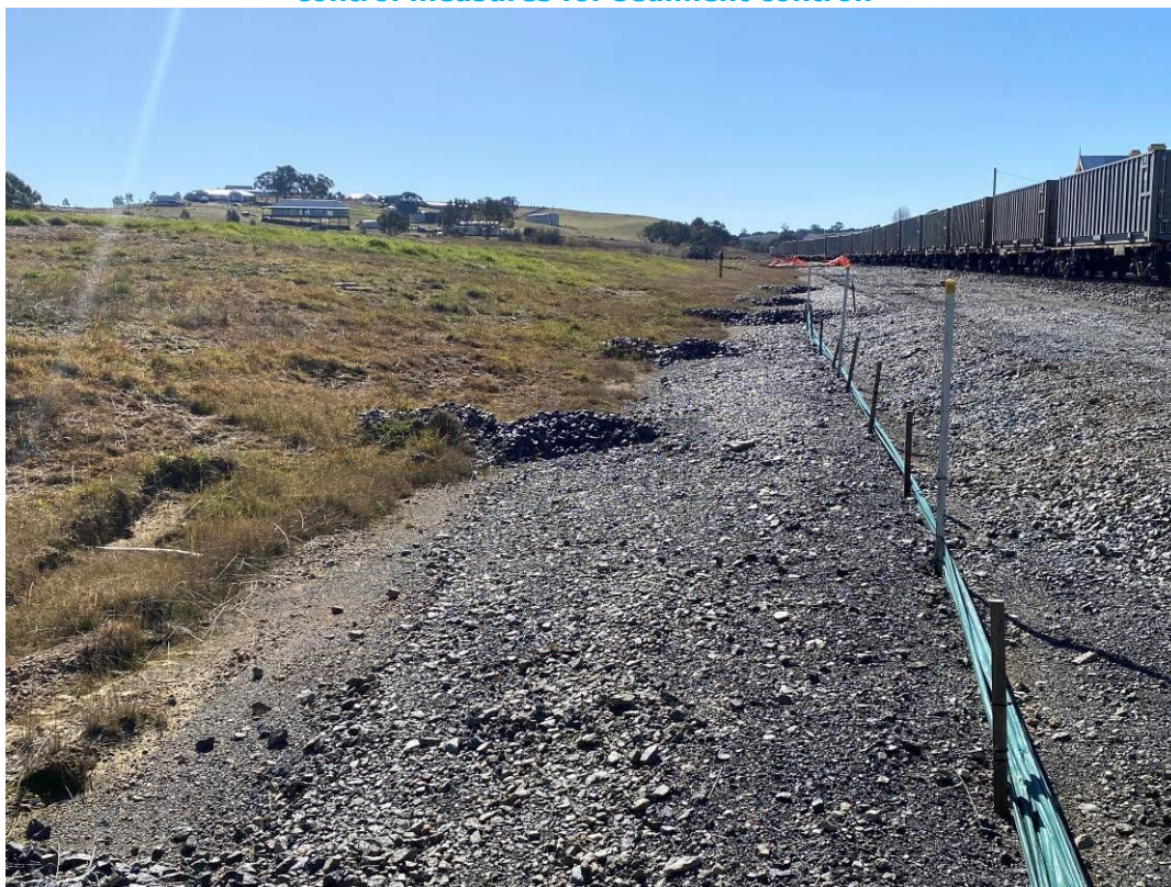
Photo 9: Upgradient of southernmost culvert showing silt fencing and rock armoury used as control measures for sediment control.
