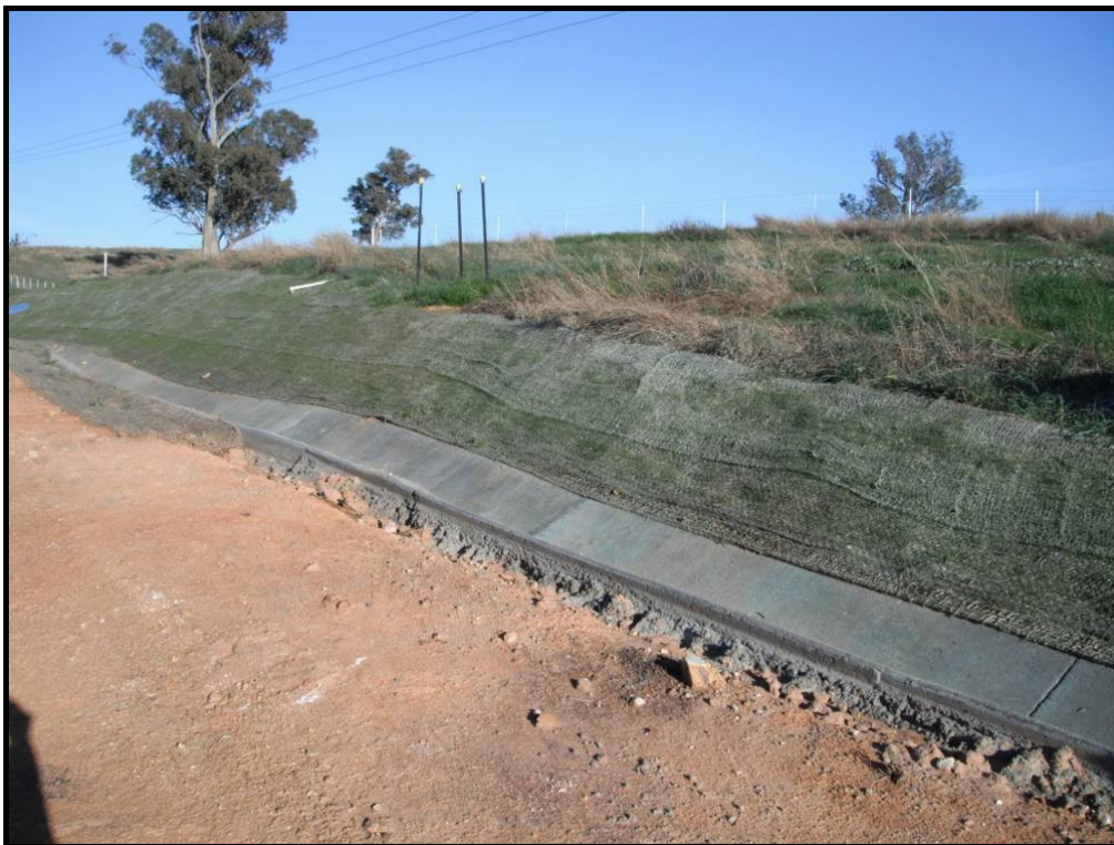
Plate 13 - Early installation and stabilisation of diversion drain for 'offsite' water.
