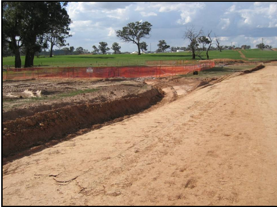
Plate 16 - Turn-out (mitre) drain to exit 'onsite' water to a sediment basin.
