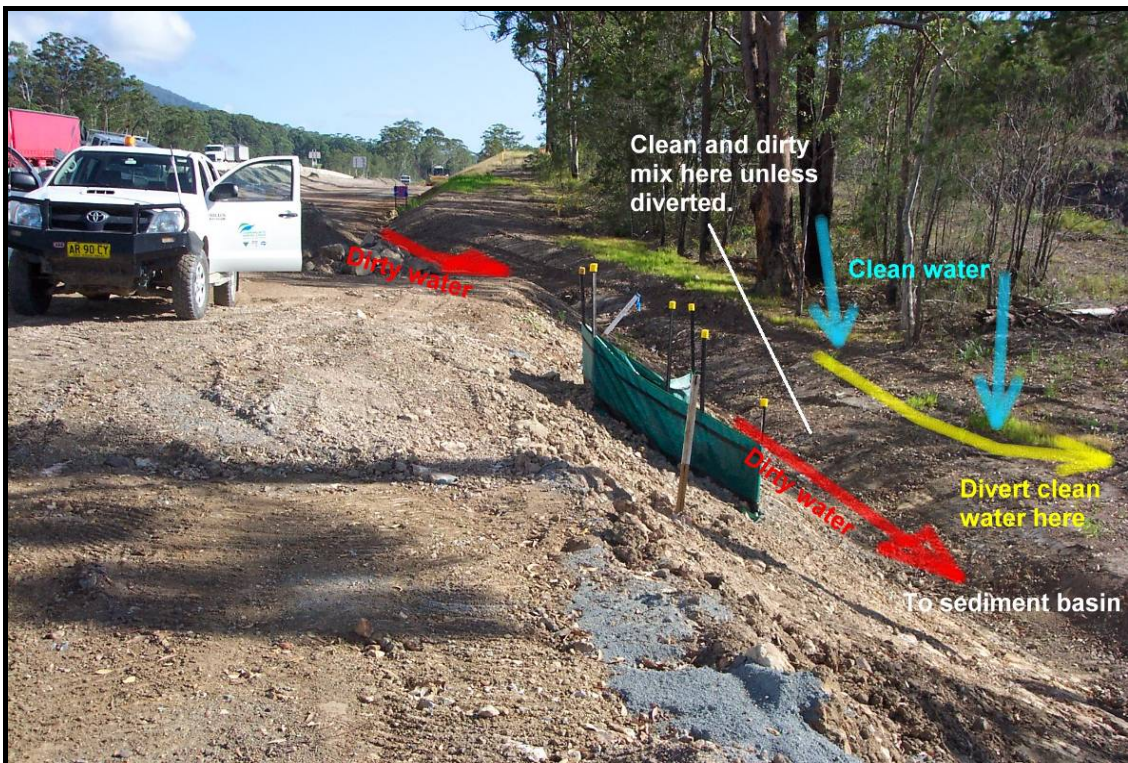
Plate 20 - Example showing offsite (clean) and onsite (dirty) water mixing at the cut/fill line. Offsite run-on should be temporarily diverted as shown using a berm, drain or sandbags so it doesn't flow to the sediment basin.
