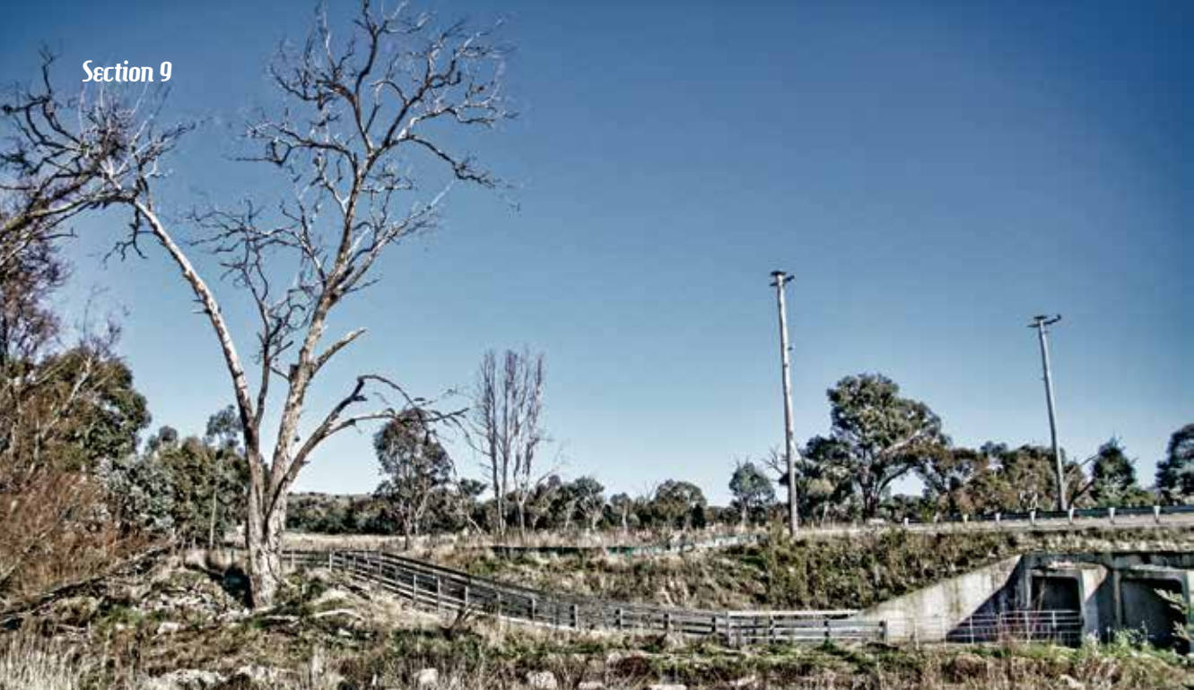
Stock underpass on Hume Highway, Kyeamba
