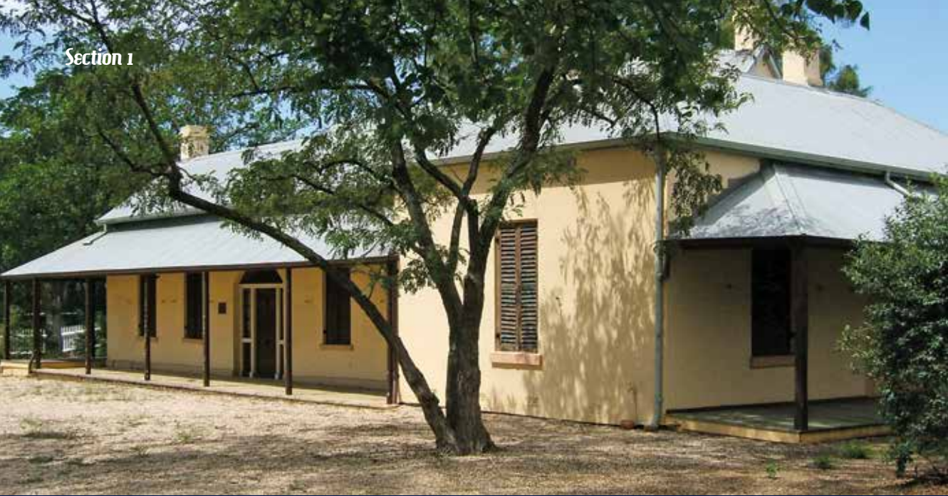
Collingwood House, built in 1810. It is the oldest house still standing in Liverpool
