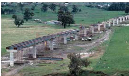
Sheahan Bridge under construction, September 1975
