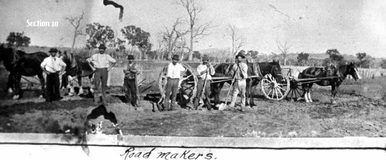
Road builders near Table Top. Photo: Howard Jones
