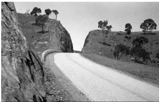
"The cut" on the completed Tumbalong to Tarcutta Deviation, 1941
