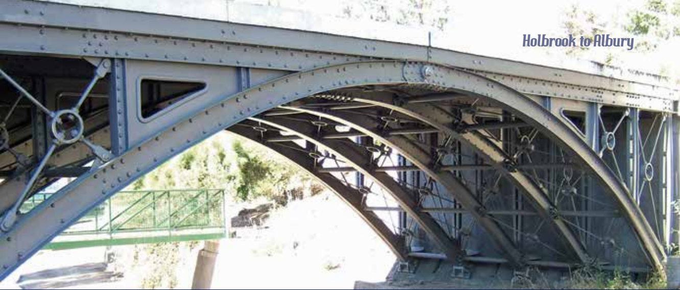
Smollett Street metal arch bridge, Albury
