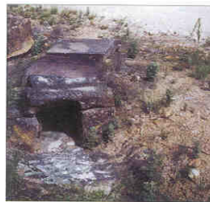
Drainage culvert under the road on Devines Hill
