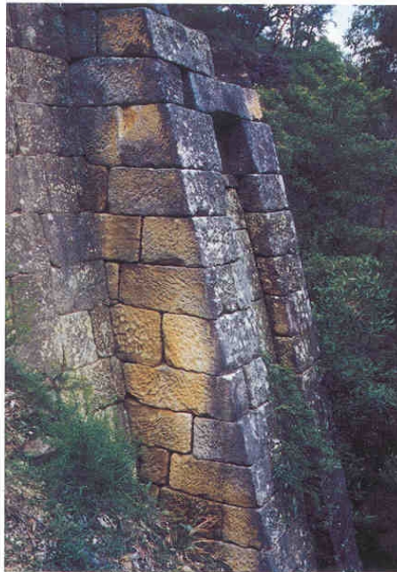
Stone buttress, built as a wall stabiliser and drainage outfall.
