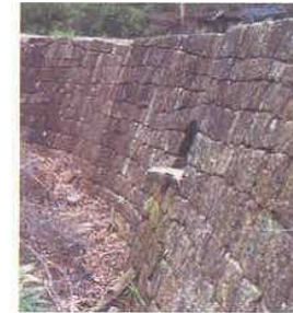
A stone retaining wall with an example of a drainage outlet
