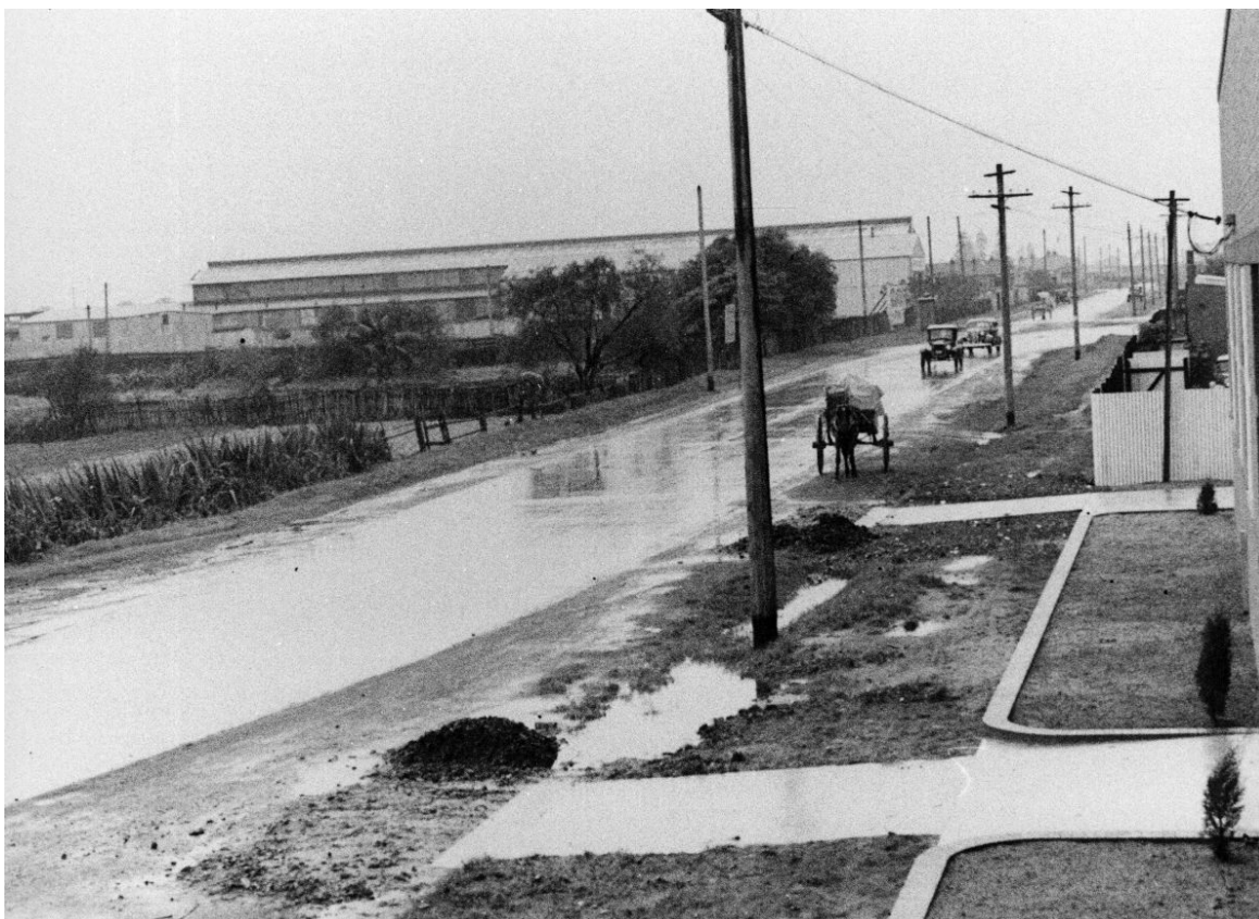
Figure 7 A single dray amongst the cars, with pavements wet with rain. Gardeners Road (MR 183) ready for widening. September 1938. Source: GPO1, 32486
