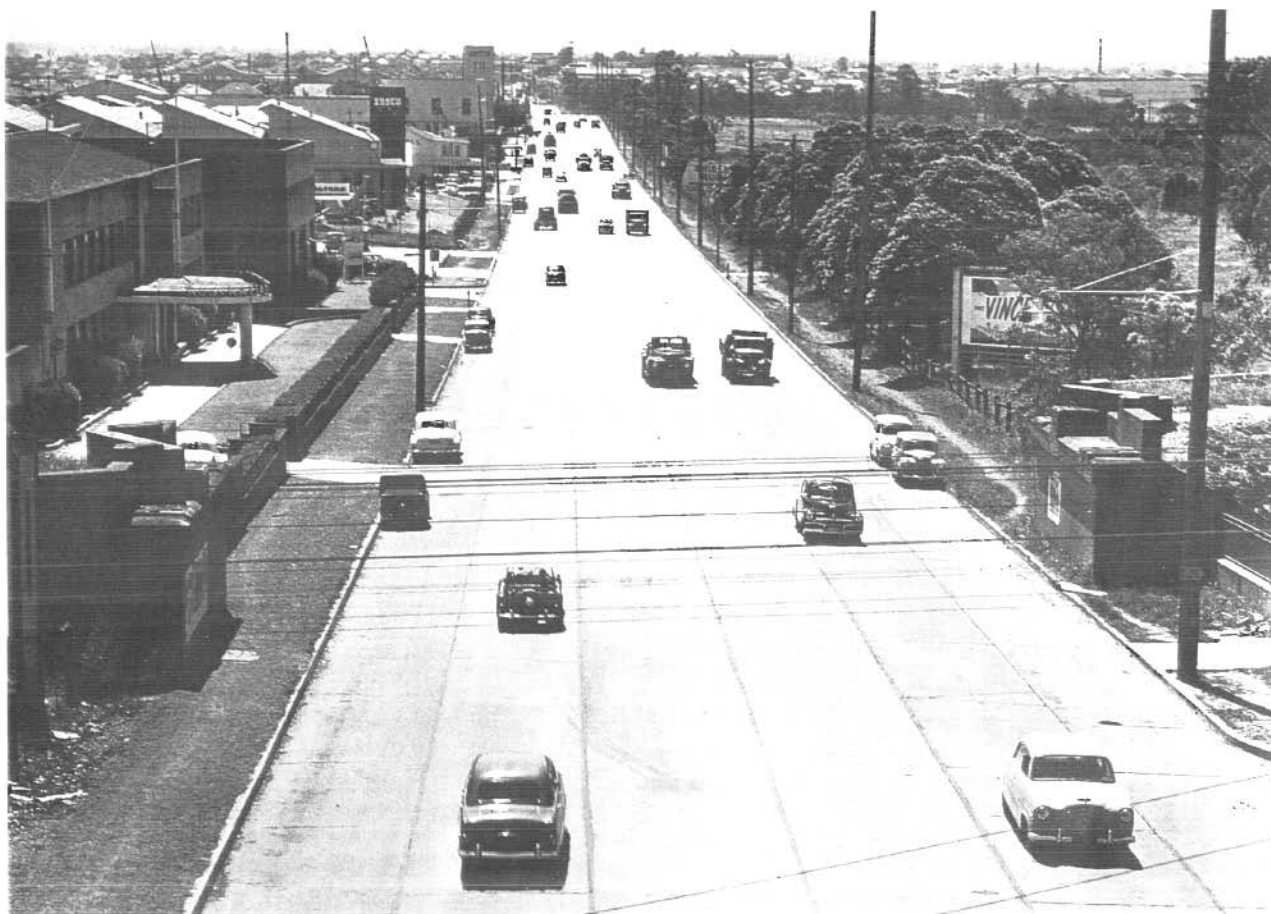
Parramatta Road, looking west at Flemington, Nov 1956 – note absence of painted centre line and lane lines
