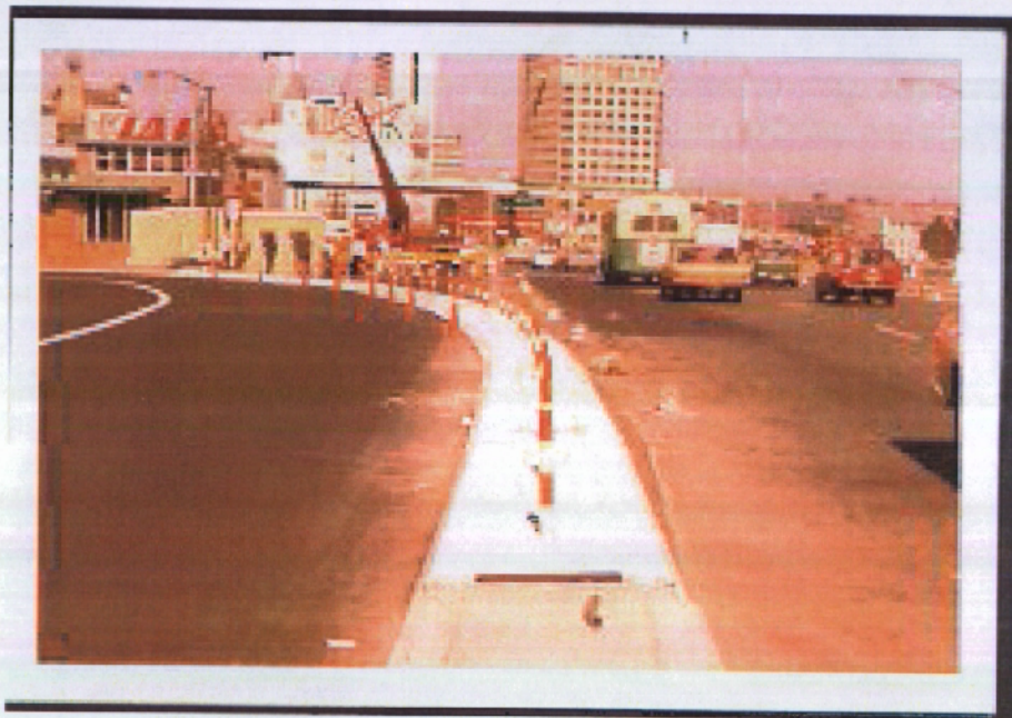
Moveable Median for Sydney Harbour Bridge (Photo: Jack Winning)
