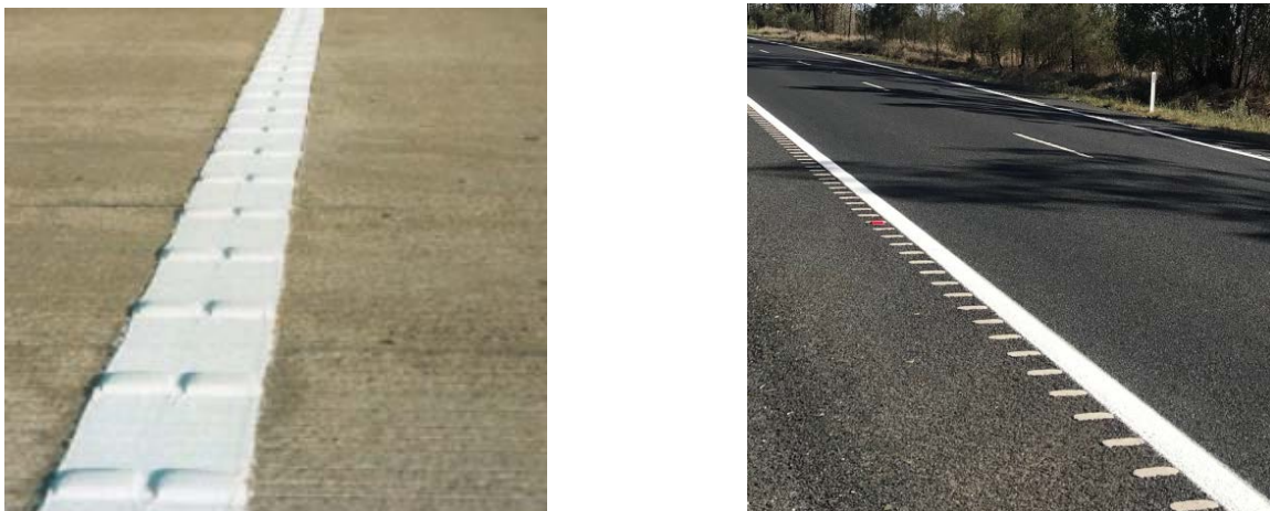
Figure 1: Examples of ATLM installation.
