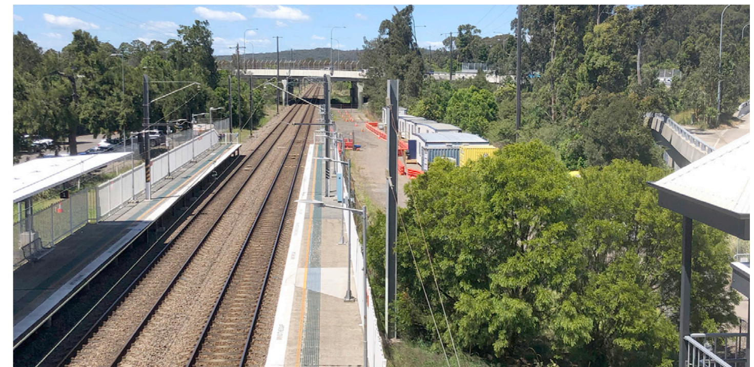
Preparing for the Tuggerah Station upgrade - site establishment underway
