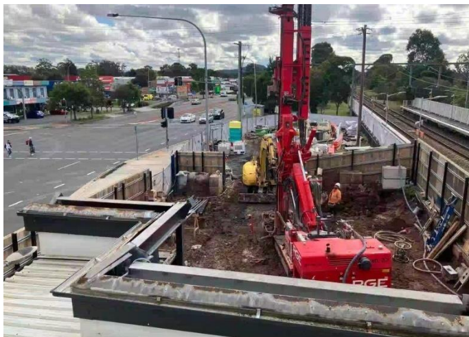
Progress of micropiling works next to platform 2.
