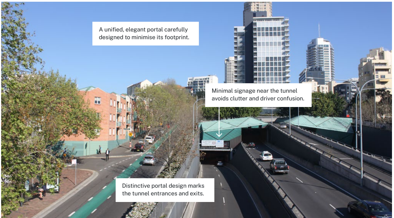
Cross City Tunnel, Sydney.
