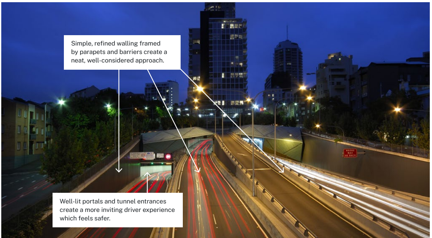
Cross City Tunnel, Sydney. (Urban design: Hassell. Photography: Rowan Turner).
