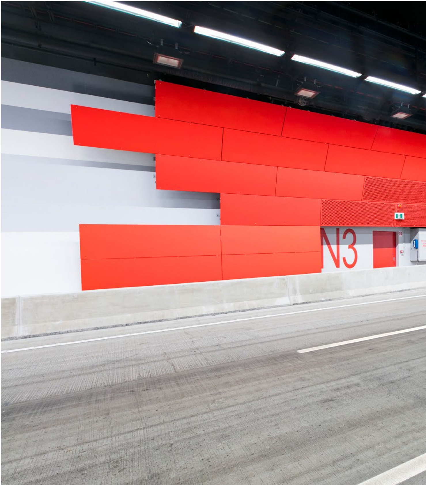
Boldly coloured panels highlight tunnel safety exit points, and the tones of grey on the walls depict the local field patterns. The whole effect provides variation and subtle stimulation to the driving experience. (St Helena Tunnel, Byron Bay NSW).
