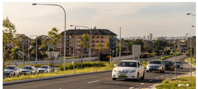
The entrance to Westconnex in Sydney at Haberfield, utilises neat panels with a strip lighting that can be modified in the control centre.
