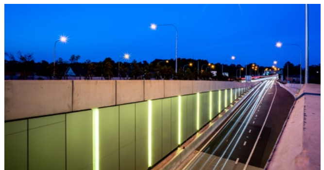
New entrance to the M4 East tunnel in Haberfield. A panelled approach with LED lighting creates a neat consistent, and distinctive finish across the tunnel system.
