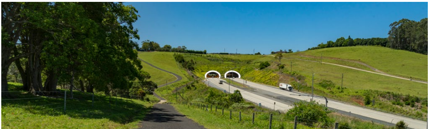
Wrapping the hillside around the portals at the Ewingsdale to Tintenbar tunnel on the Pacific Highway created a low impact design solution that respected the landform and landscape of the area.
