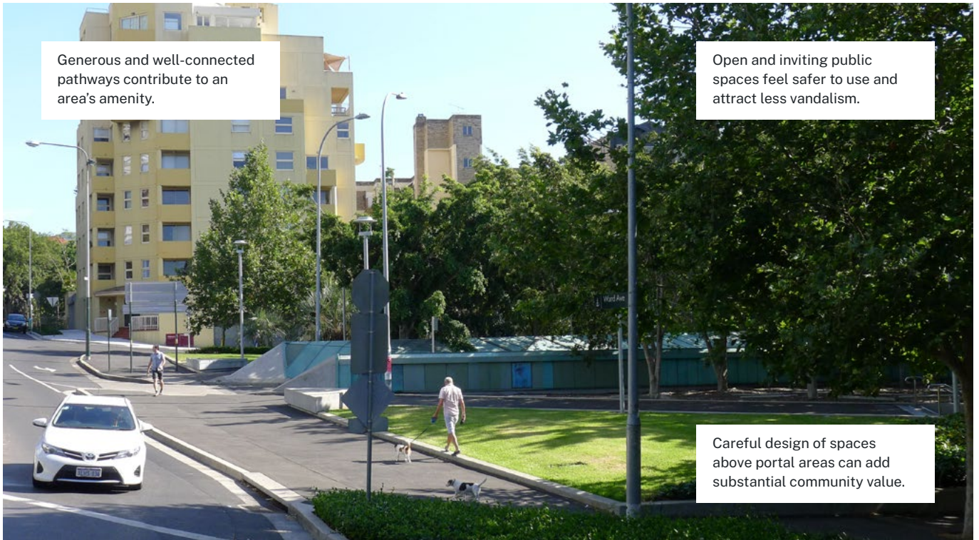
Cross City Tunnel, Ward Avenue Park, Sydney.
