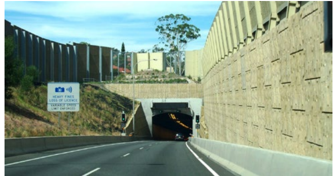
The M5 East tunnel approach and portal area in Sydney (including associated structures and elements) presents as a cluttered and uninviting experience for motorists.
