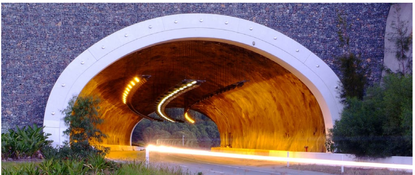
A generously proportioned, attractive portal greets motorists in the Cudgen Road tunnel. Journey safety is reinforced by the overhead lighting accentuating the curved alignment, and improving the visual experience of the tunnel. (Pacific Highway, Yelgun).
