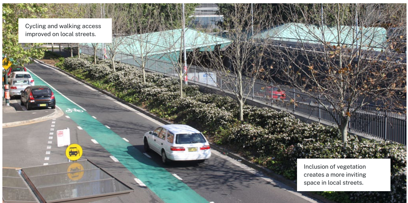
Cross City Tunnel, Sydney.
