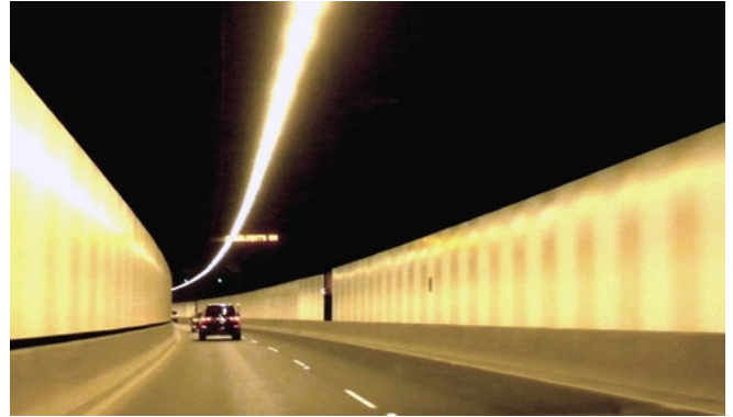
A simplified panel attached system in the Lane Cove Tunnel avoided unnecessary fixings and cover plates, which collect dirt and grime, making them easier to clean.
