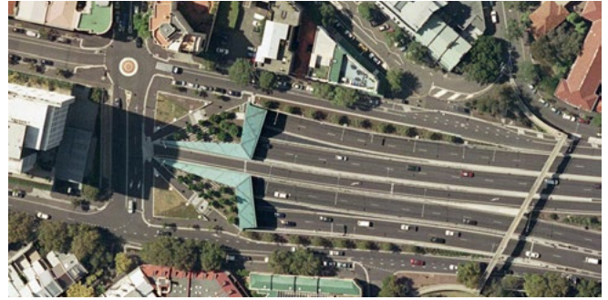
Despite limited space for the approaches and portals to the Cross City Tunnel in Sydney, the adjacent streets and public spaces include well-considered design details and local access.
