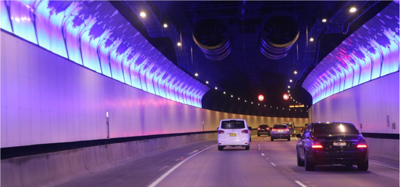
The 9km long Northconnex tunnel utilised a range of creative features to provide subterranean interest, visual comfort, support patronage and result in less vehicles on the surface in neighbourhoods.
