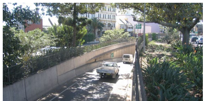
Careful design of this dive structure and portal to the Eastern Distributor tunnel (above two images) maintained essential landscape characteristics (including several large existing trees), as well as good local connectivity for motorists, pedestrians and cyclists.
