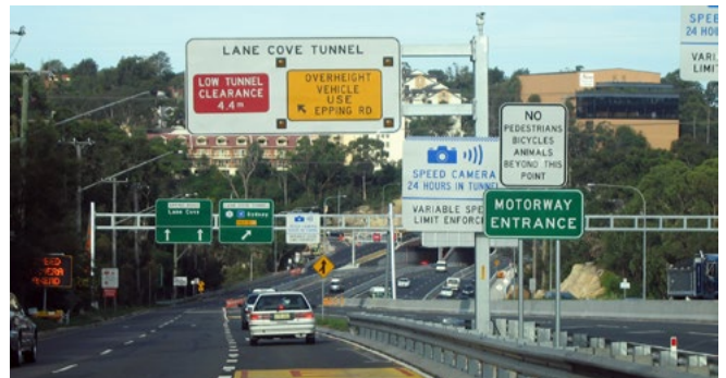
Too many signs on the approach to a tunnel can be confusing for drivers. The appearance of this approach to the Lane Cove Tunnel in Sydney is unsightly and obscures the effort undertaken in designing the portal.
