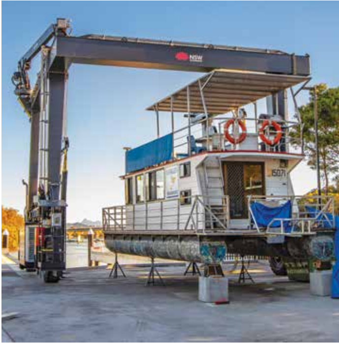
The new boat maintenance travel lift in action
