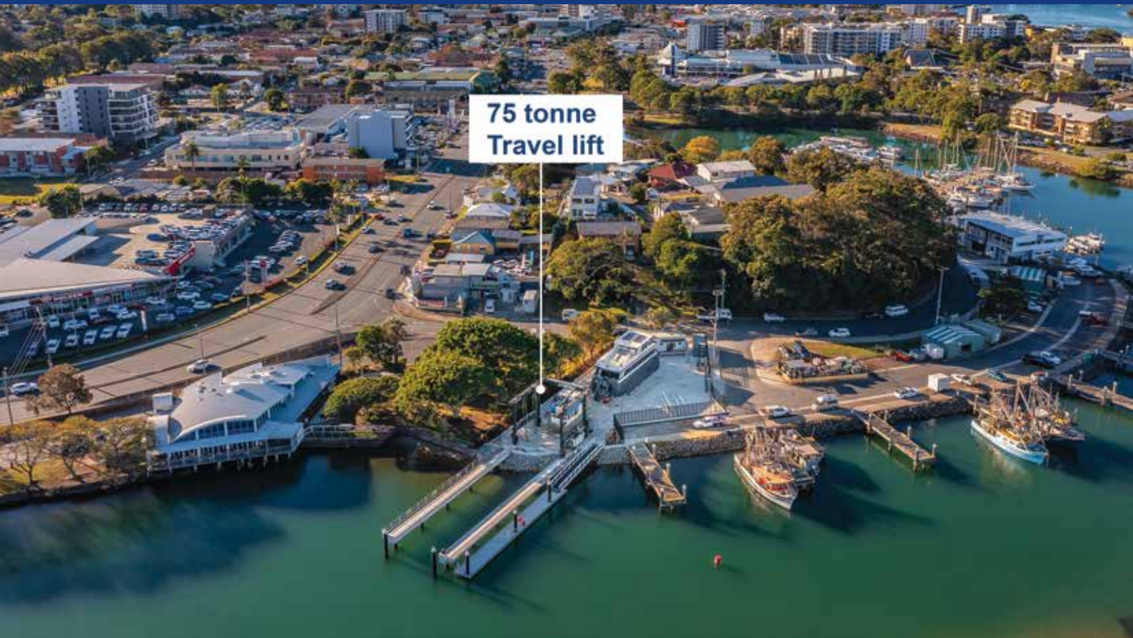
Aerial view of the current Tweed Head Boat Maintenance Facility
