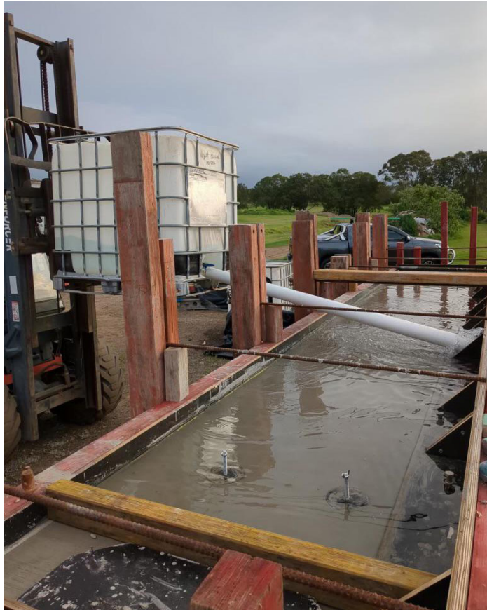
Offsite fabrication of the precast runway beams.
