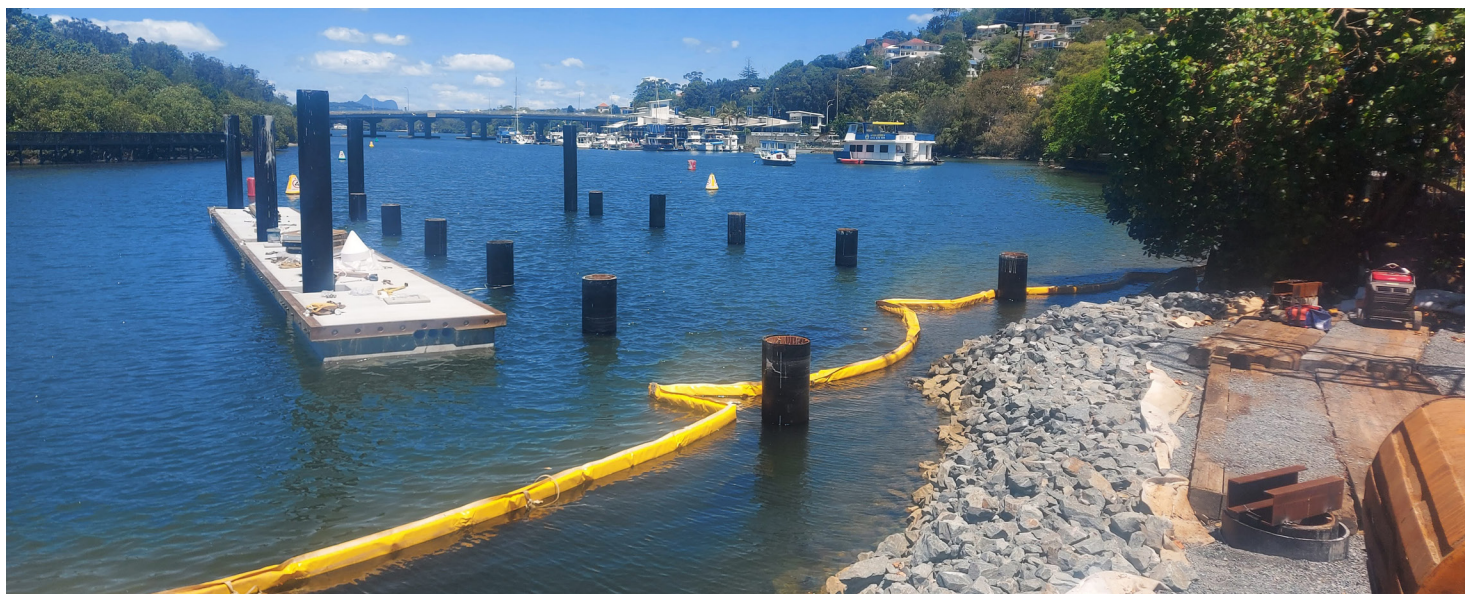
Installation of the steel piles.
