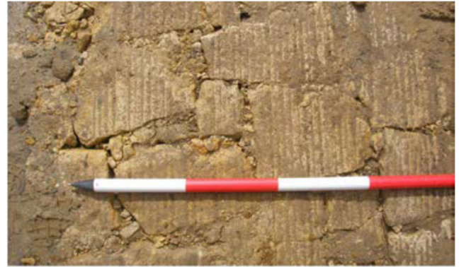
Figure 4: Close up detail of the sandstone surface showing material type, formation and construction detail. This is essential for establishing date of the feature.
