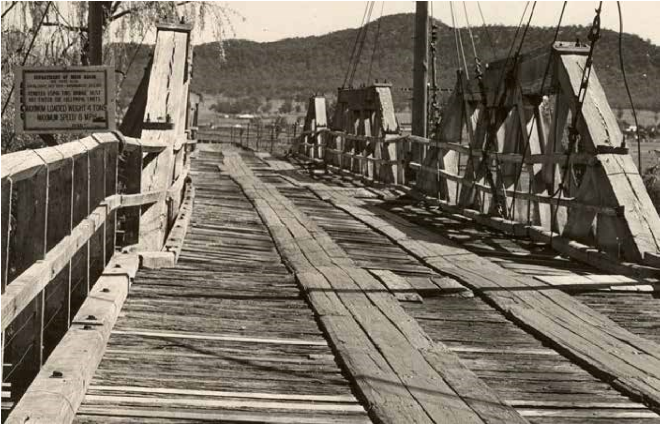
Figure 2-50: Typical Running Planks on Timber Bridge
