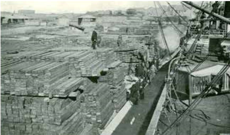
Figure 2-2: Australian hardwood sleepers and girders being loaded at Darling Harbour for South Africa in 1903
