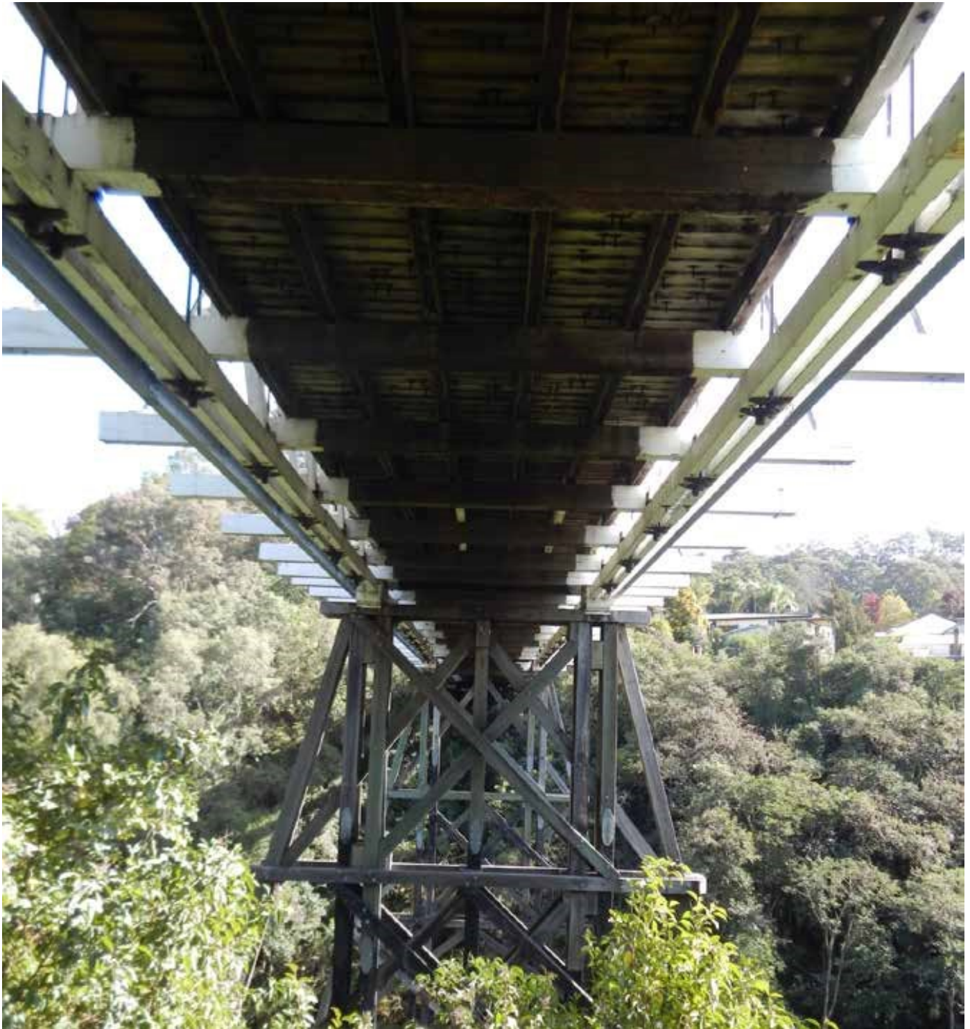
Figure 2-78: Photo of existing stringers and spaced transverse decking
