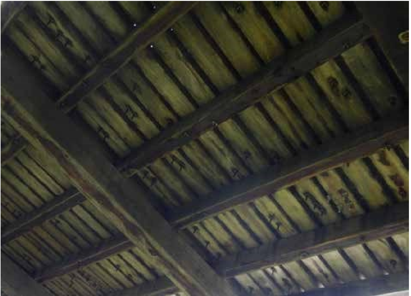
Figure 2-79: Bolted and spaced decking
