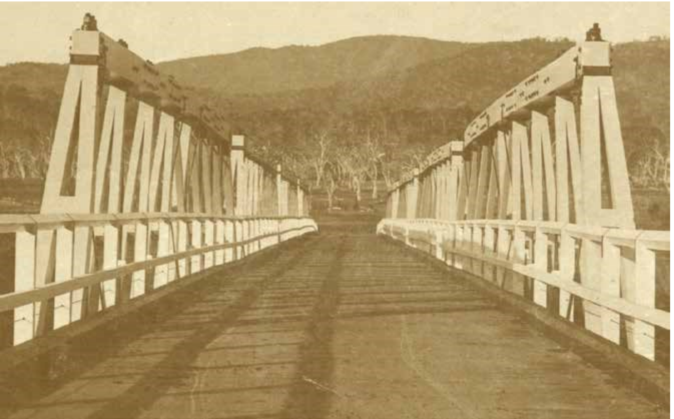
Figure 2-17: Original timber deck on Tharwa Bridge, undated
