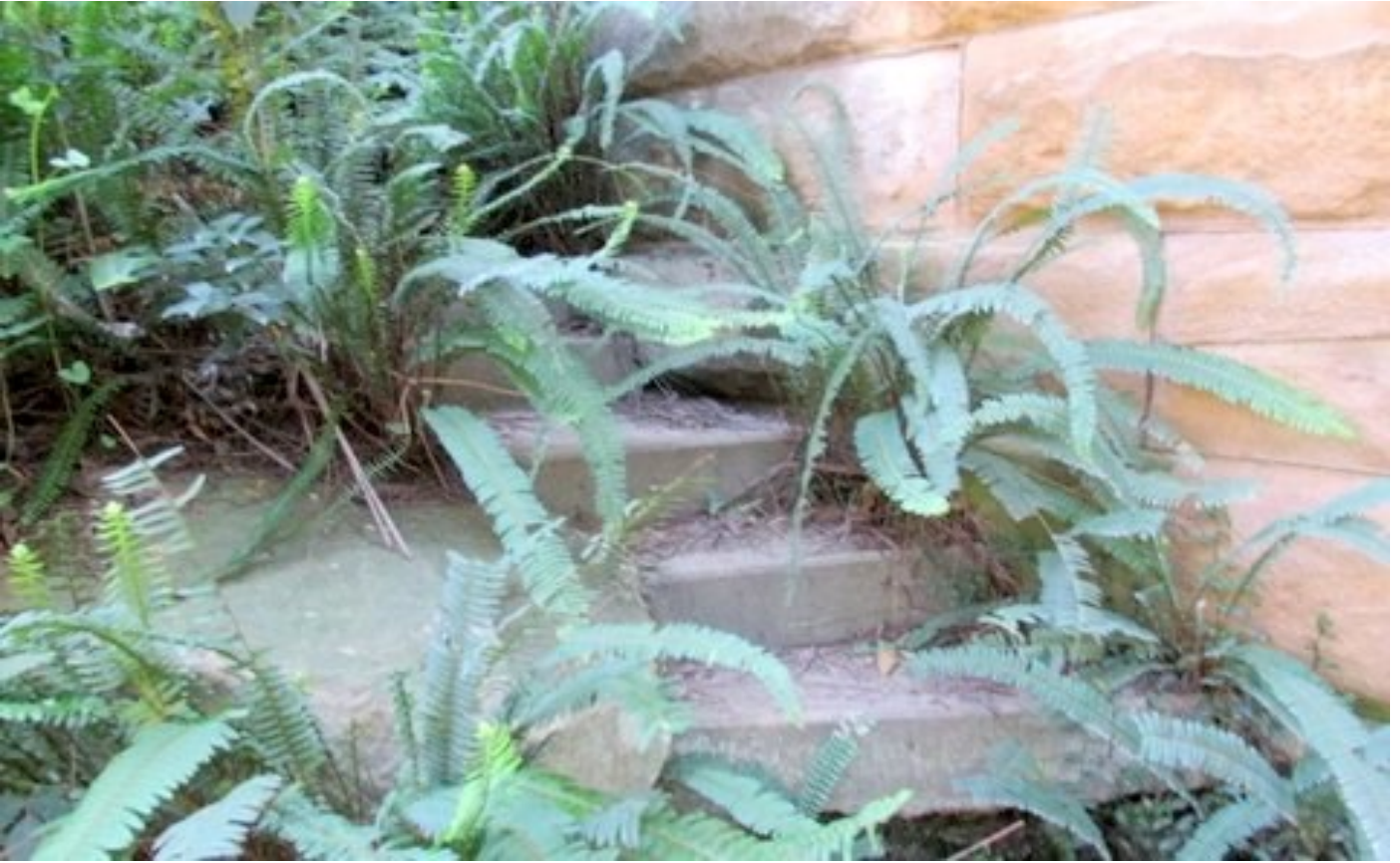
Figure 2-28: Flight of steep steps down viaduct wall 85
