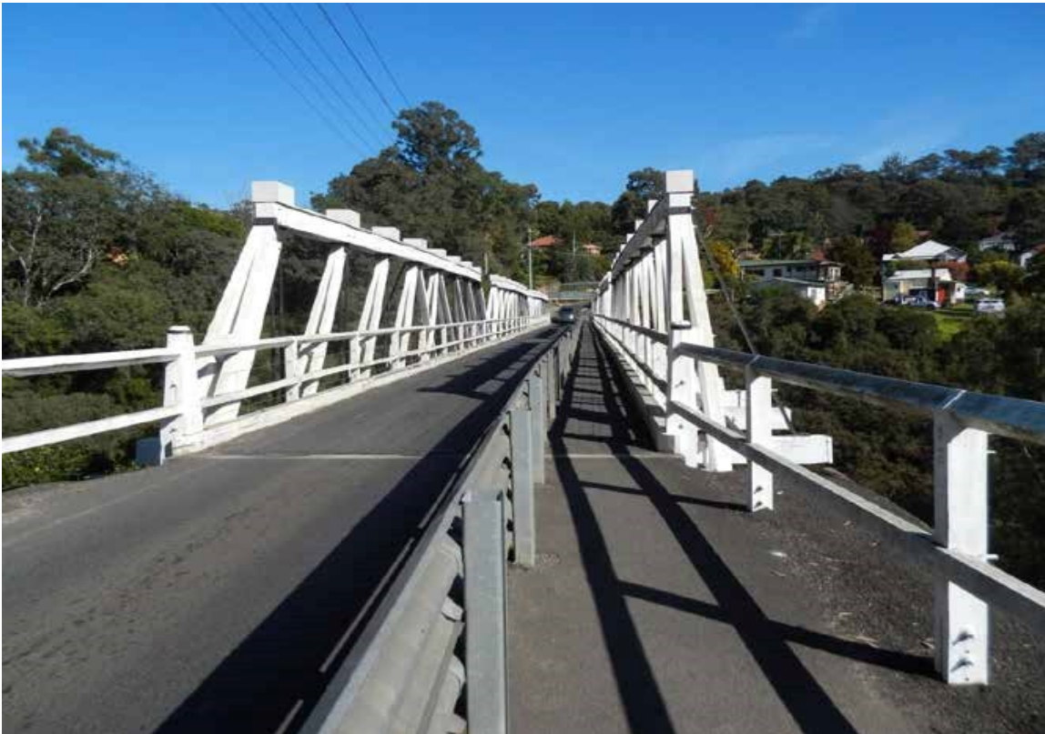
Figure 1-4: Victoria Bridge in its setting from close up, facing west
