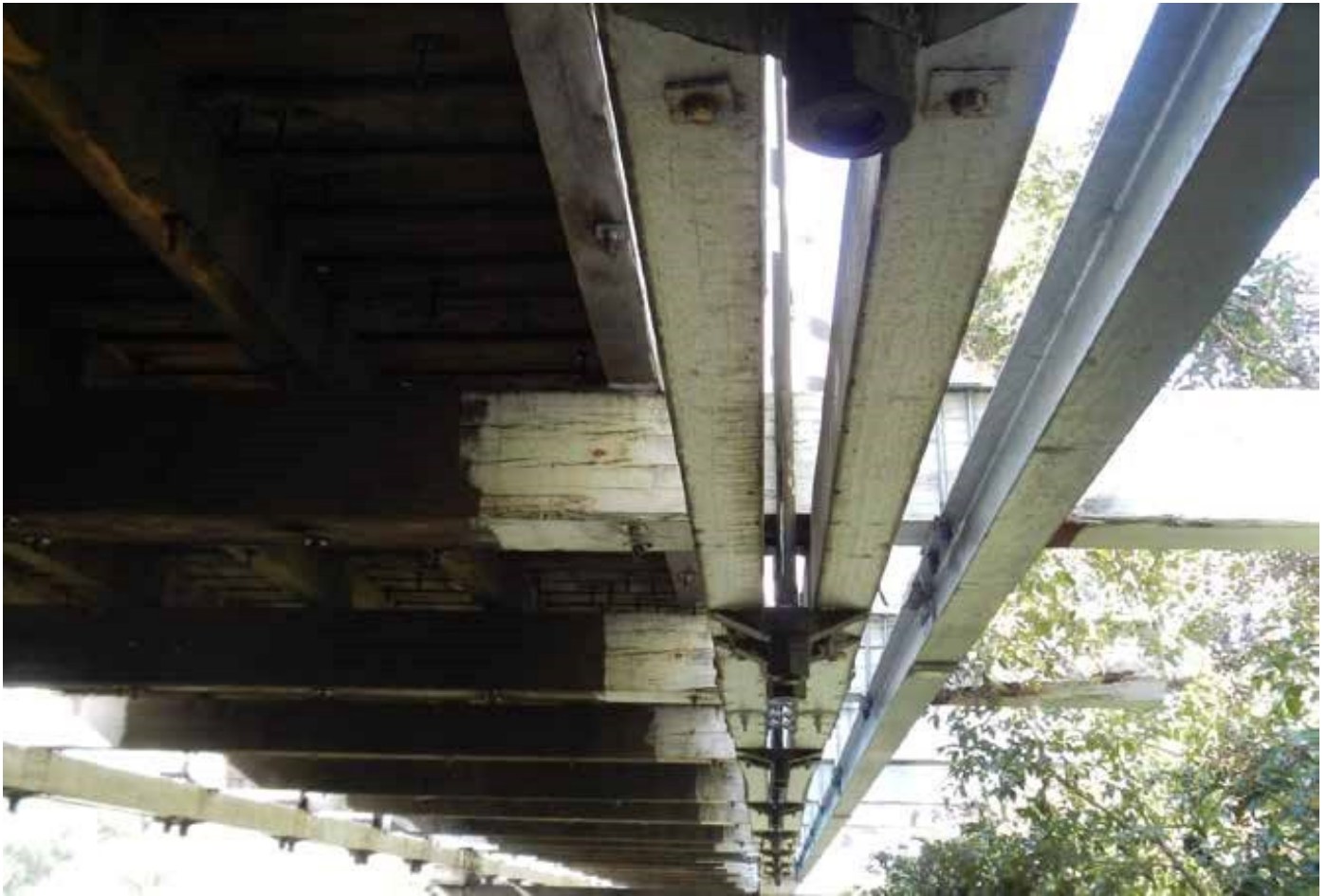
Figure 2-60: Photograph of timber bottom chord taken from under bridge
