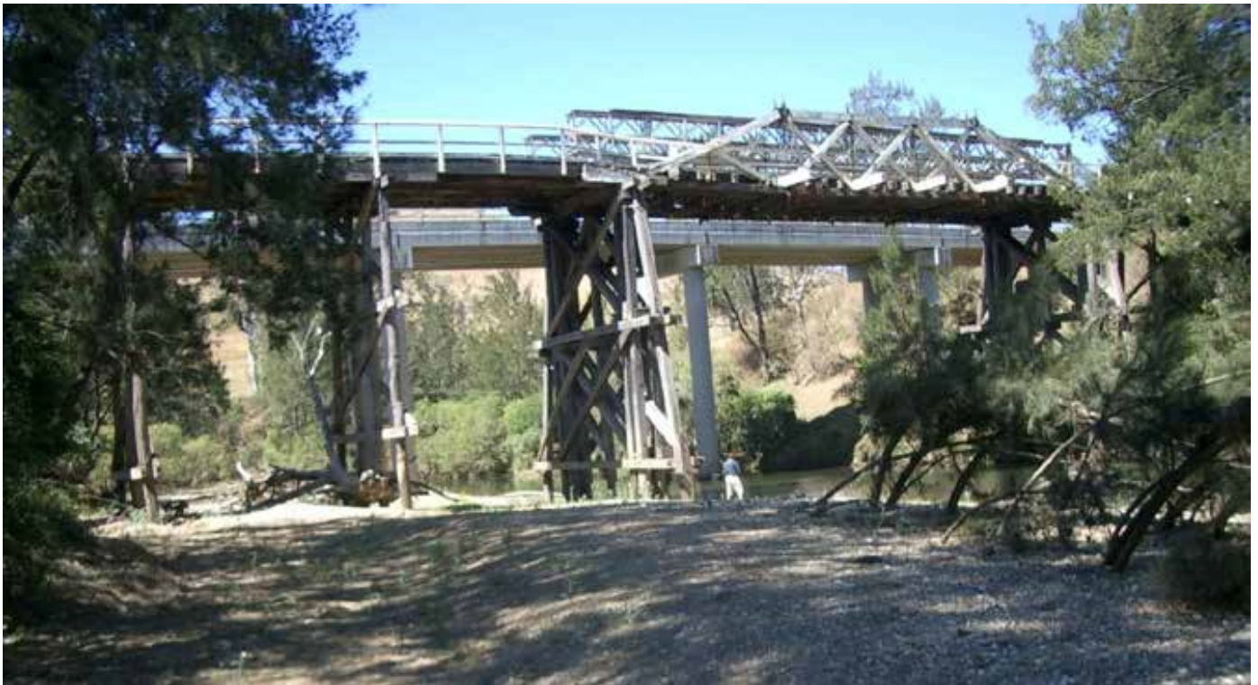
Figure 5-2: Five Day Creek Bridge (since demolished) with concrete bridge
