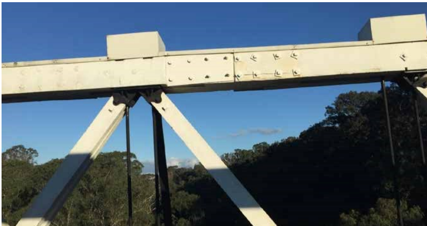
Figure 2-57: Additional splice at D-E in Span 2 Downstream
