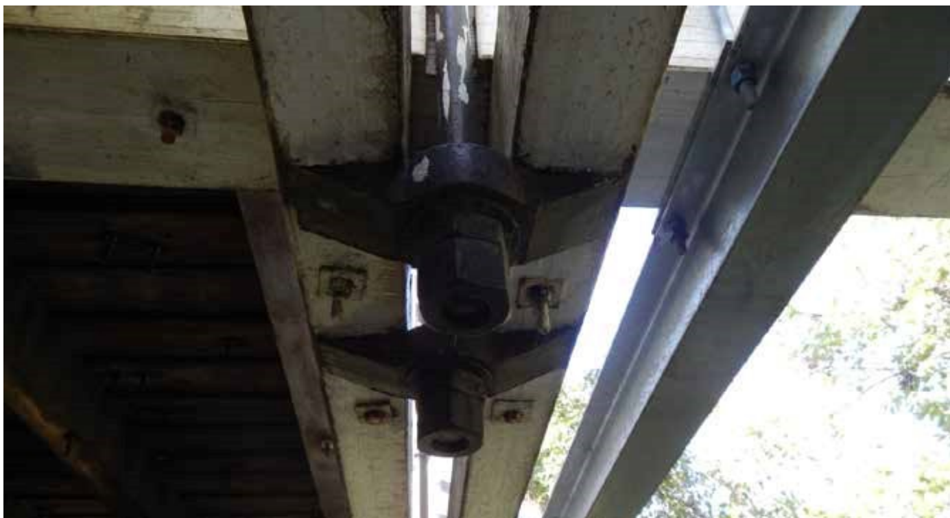
Figure 2-65: Photograph of thin nuts and main nuts only partially threaded
