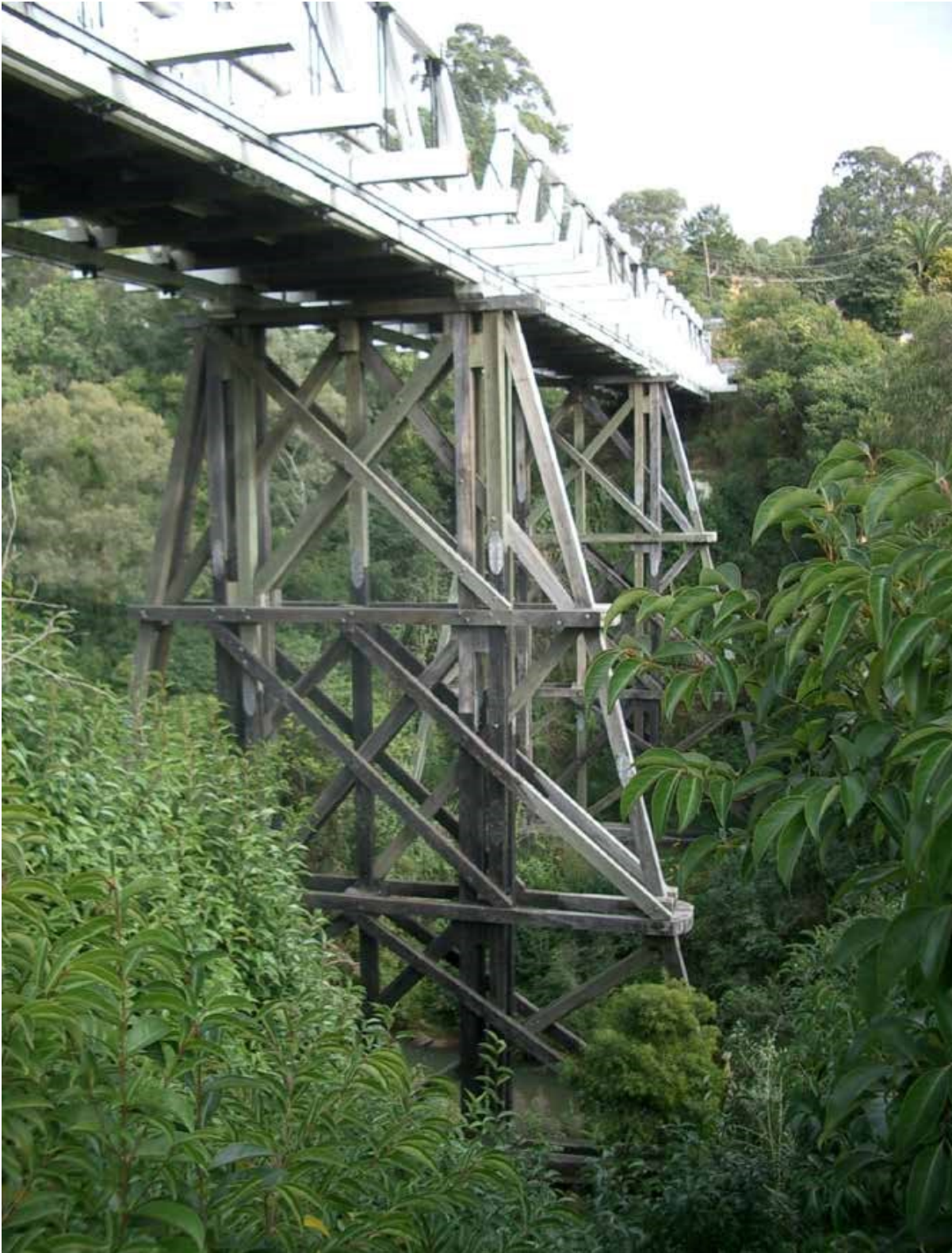
Figure 2-86: Timber double trestle piers at Victoria Bridge
