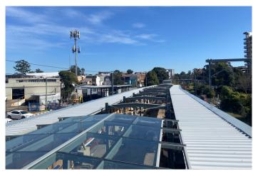
Above: View of the new canopy sections during installation. The roof design includes glass panels to provide natural light for commuters.
