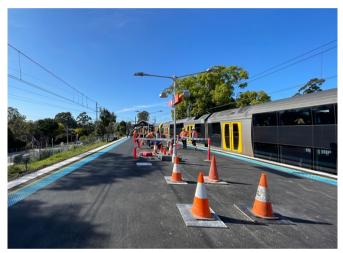
Above: New asphalt surface on platform with yellow and blue tactile ground surface indicators.
