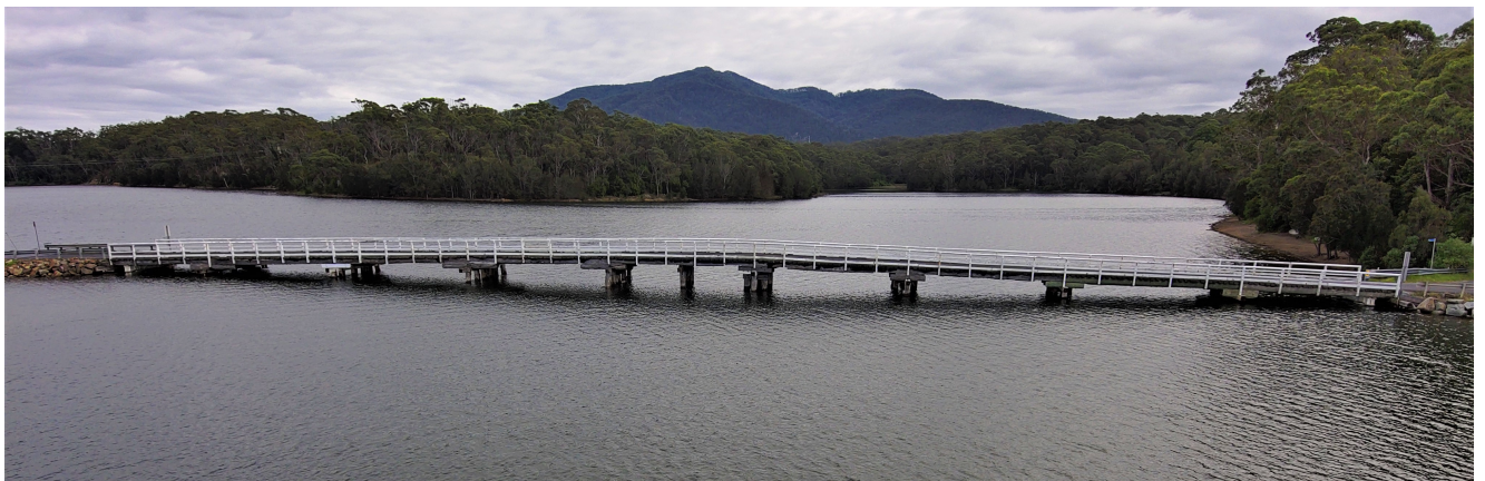
Looking west towards Wallaga Lake Bridge. Picture taken April 2023.
