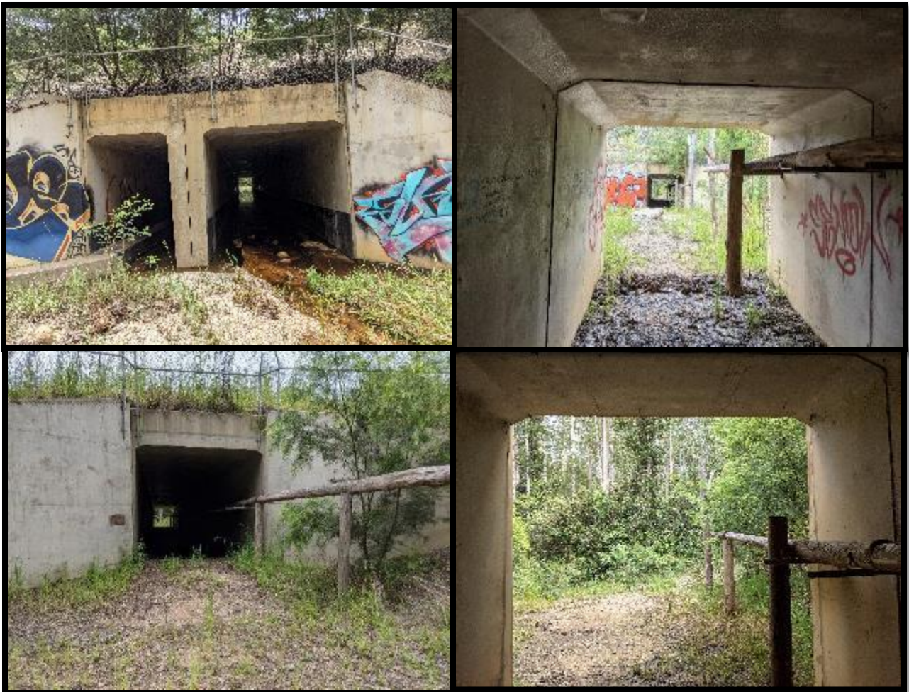
Plate 1. Dual box culverts with designated wet passage at site 5 (top left). Split median box culverts at site 9 and 10 (top right). Fauna furniture entering (bottom left) and exiting site 8 (bottom right).
