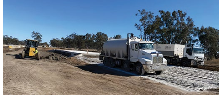
Moree Plains Shire Council carrying out roadworks
