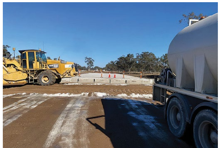
Moree Plains Shire Council carrying out roadworks
