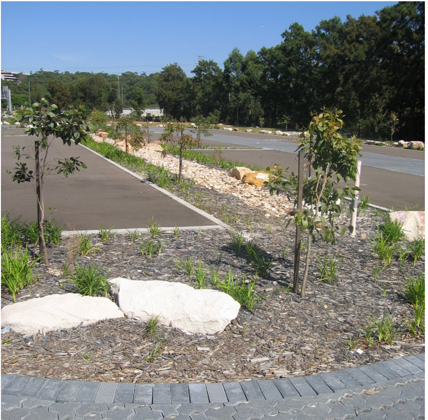
Figure 14. Permeable pavement in car park constructed as part of the Lane Cove Tunnel project
