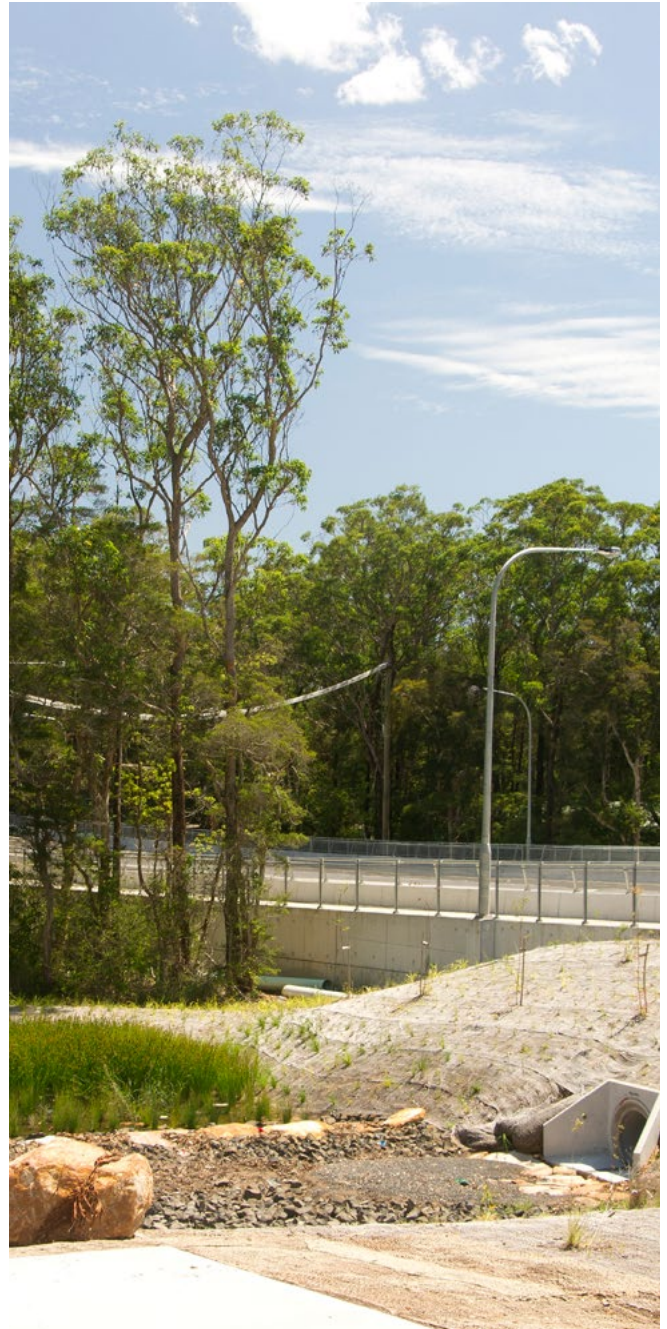
Figure 15. Bioretention basin with sediment entrapment zone on the Central Coast Highway, Wamberal
