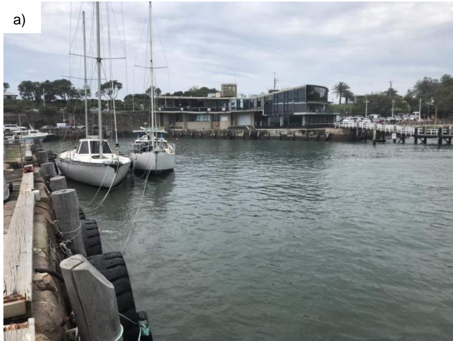
Plate 2: a) Marine extent of the study area, consisting of steep sandstone seawall, wooden piles and large rubber tyres used as fenders.
