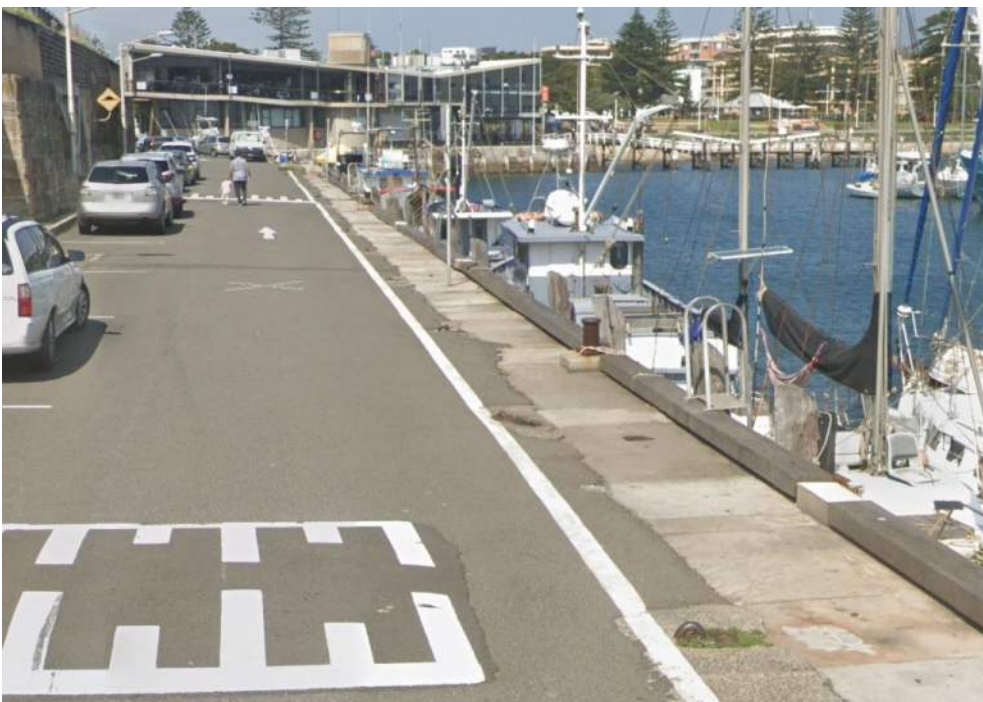
Figure 1-11 Existing Path Condition around Belmore Basin
