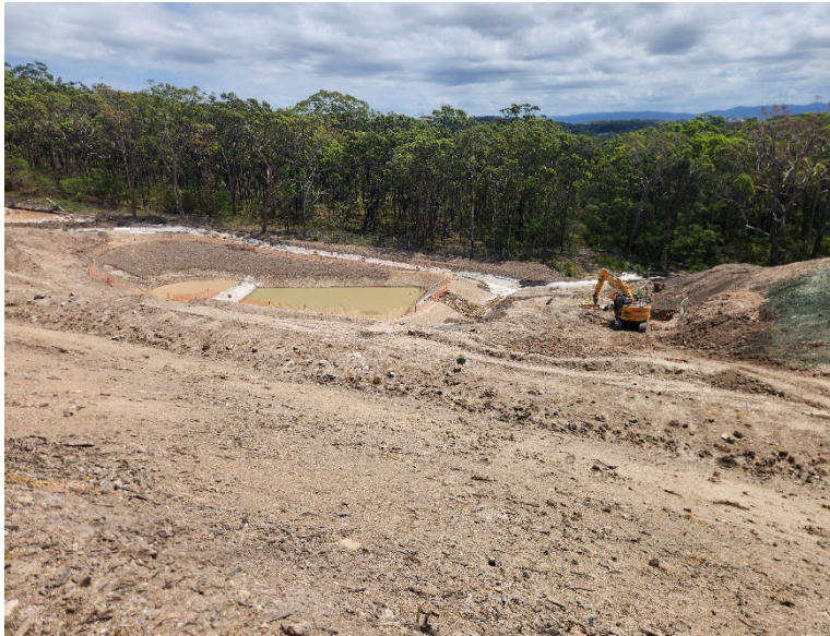
Image 5: Midway through main line, view looking west. ErSed controls in this area have been reinstated.
