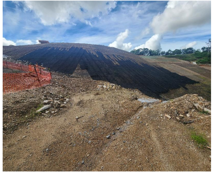
Image 6: Southern Interchange permanent landscaping works.
