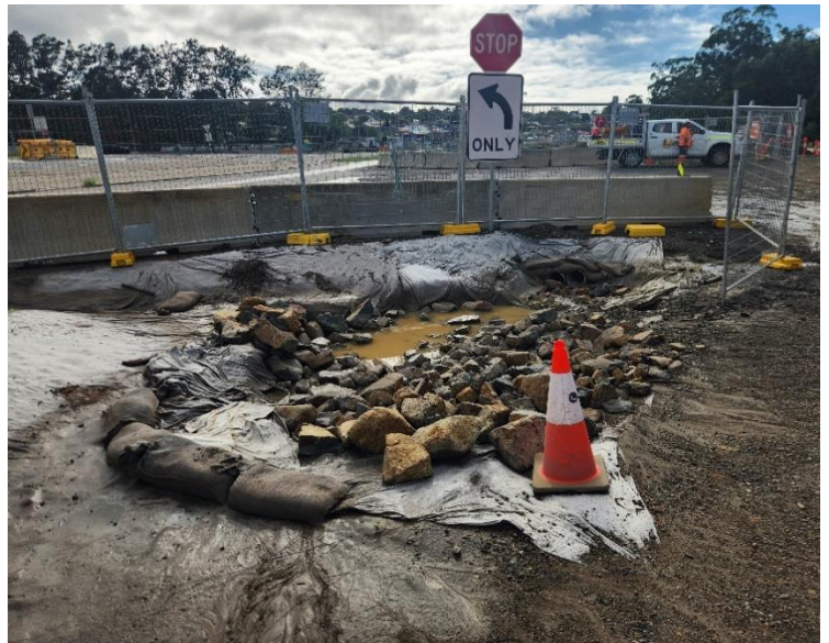
Image 2: Northern Interchange, view of the entry to the compound and site.
