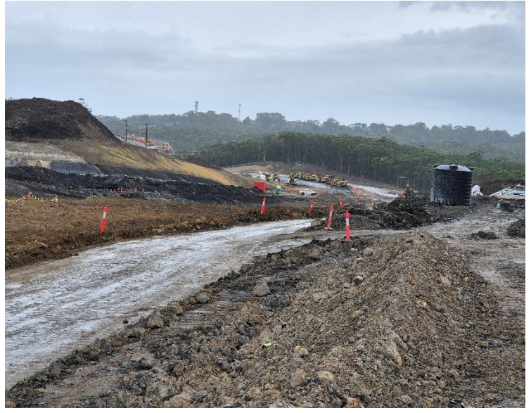
Image 4: Mainline looking South with JHH interchange on the left.
