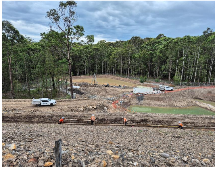
Image 2: Mainline storage basin (background) and sediment basin (foreground). The sediment basin has recently been cleaned out and returned to capacity.
