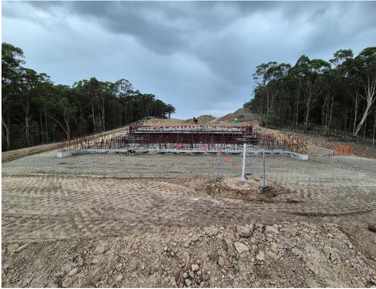
Image 3: Mainline at Fauna underpass. View looking South.
