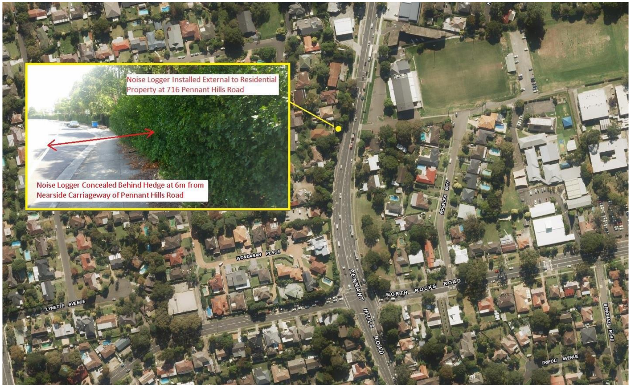
Figure 6-1 Noise monitoring location outside 716 Pennant Hills Road, Carlingford
