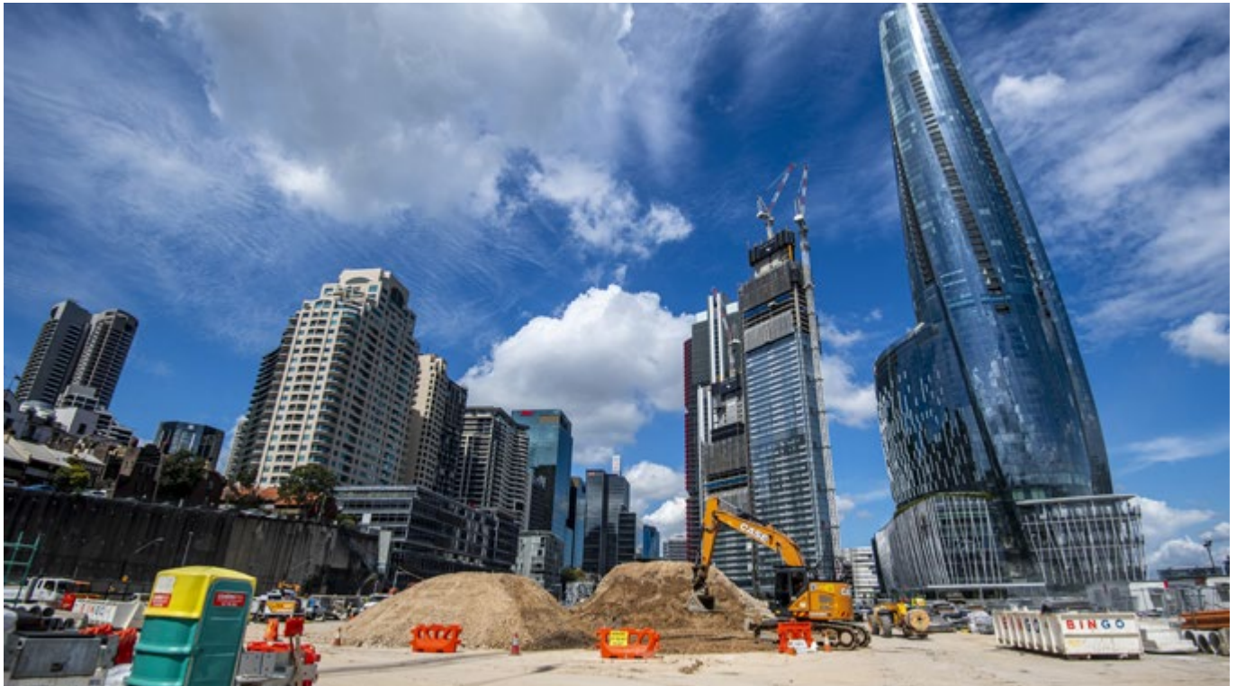
Image: Spoil from other sites being delivered to the Barangaroo site to be used for the new Hickson Road construction.
