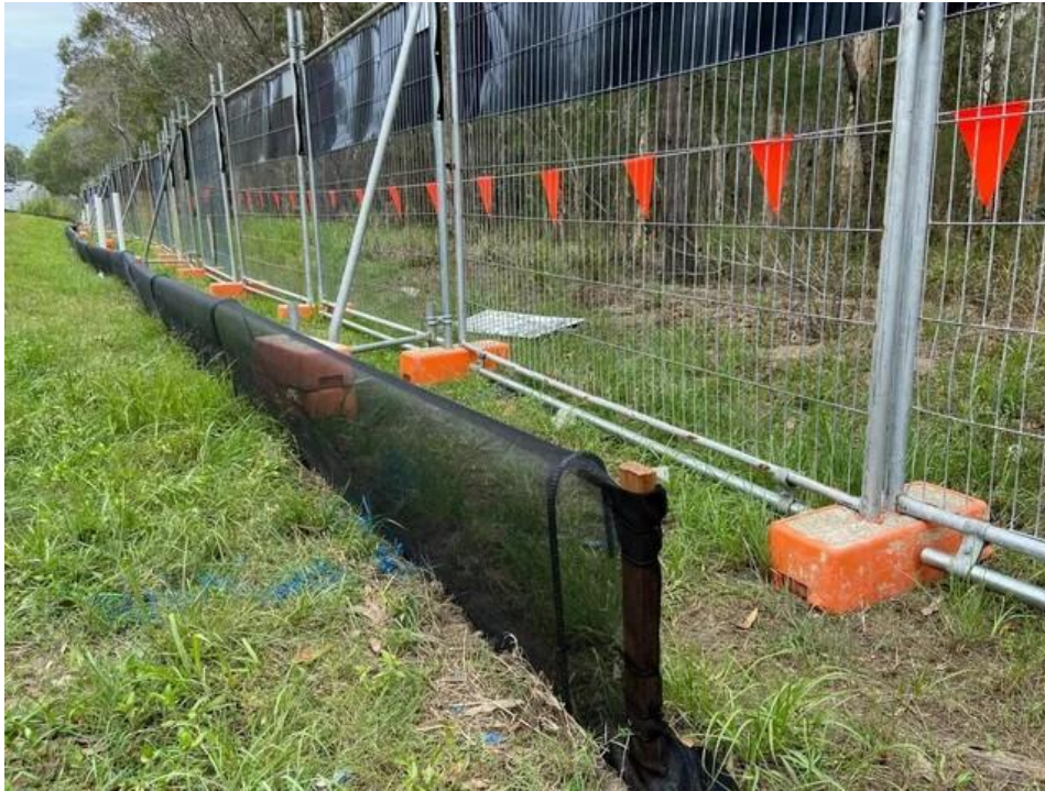
Figure 4-10 Temporary fauna exclusion fencing. 28
