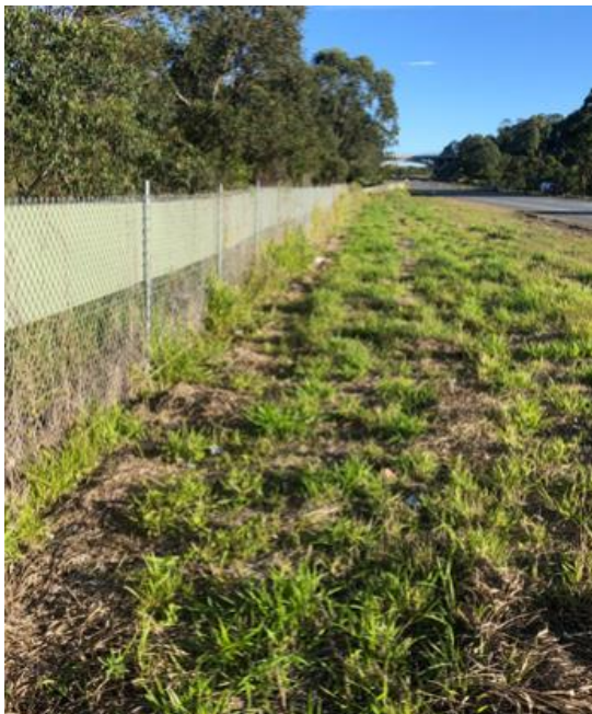
Figure 4-9 Koala Exclusion Fencing on section of the Pacific Highway upgrade, NSW. 27
