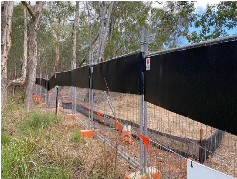
Figure 4-11 Temporary fauna exclusion fencing. 29
