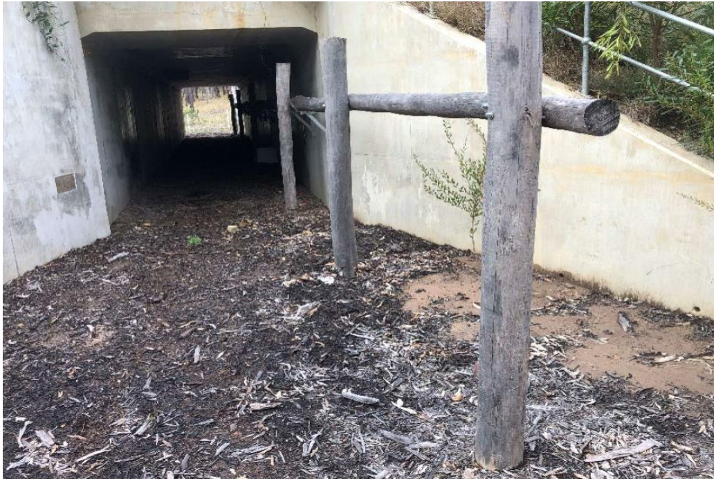
Figure 4-1 Example of a 2.4 metres x 2.4 metres Reinforced Concrete Box Culvert (RCBC). 17
