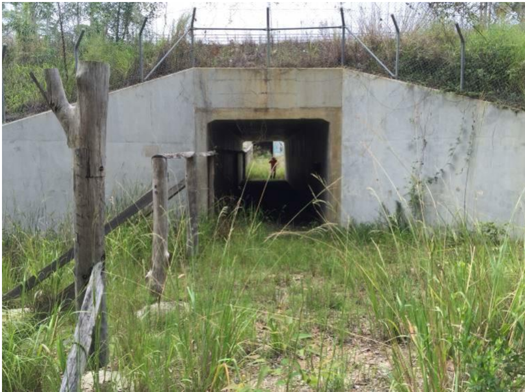
Figure 4-7 Example of fauna furniture and refuge pole used in the Pacific Highway Upgrade. 23
