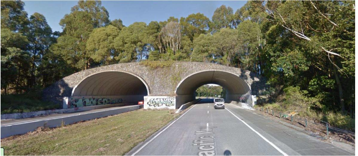
Figure 3-4 Fauna overpass (comprising two concrete arches) across the Pacific Highway, Yelgun to Chinderah, NSW. 11
