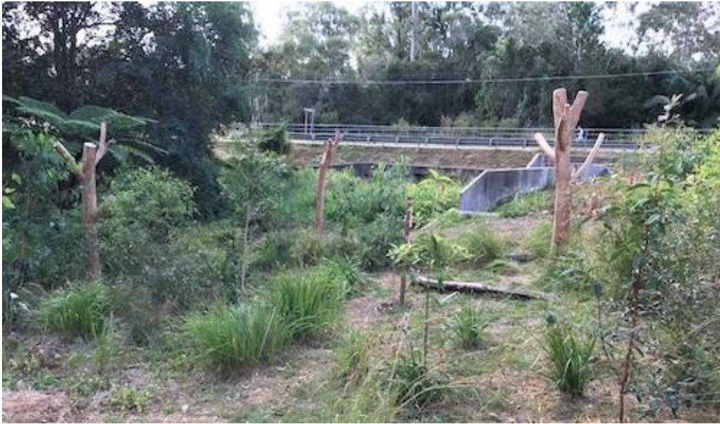
Figure 4-8 Example of refuge poles used at Pine Mountain Rd on Salvin Creek (Brisbane City Council). 24
