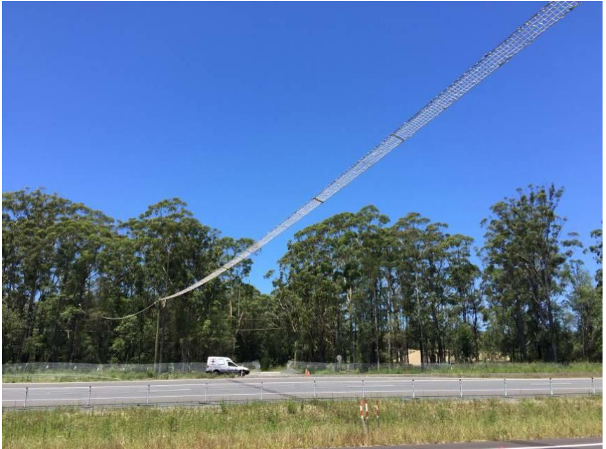
Figure 3-8 Example of aerial rope crossing across the Pacific Highway Upgrade. 13
