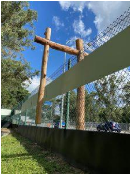
Figure 4-13 Example of escape poles install by Brisbane City Council. 31
