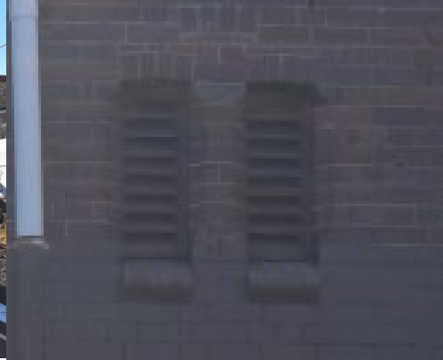
Figure 32. Close up of brick capping, downpipe and windows featuring timber louvre vents on the west elevation.
