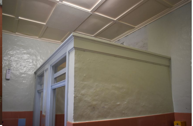
Figure 48. Internal view of the male toilet facing east. Mismatched wall tiles are evident.
