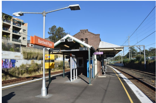
Figure 34. View of east elevation concealed by a modern gable roof awning.
