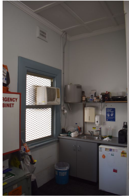
Figure 44. Close up of aluminium framed window within timber frame on the south elevation. An air conditioning unit has been inserted within.
