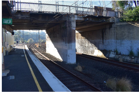
Figure 58. View of the southern end of the overbridge, featuring original brick piers with later white paint.
