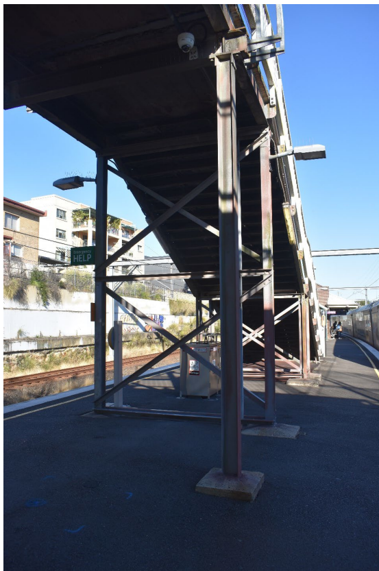
Figure 56. Entry staircase featuring the original steel superstructure
