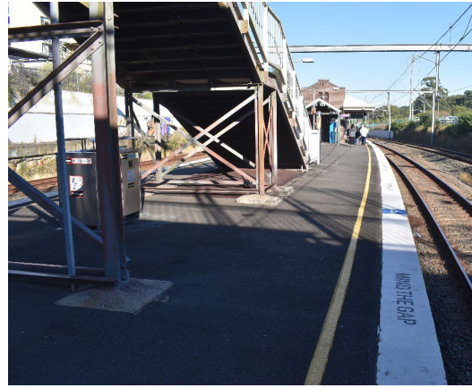
Figure 55. Entry staircase featuring the original steel superstructure.
