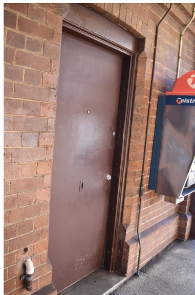
Figure 36. Close up of modern timber flush door and adjacent wall mounted telephone booth on the south façade.
