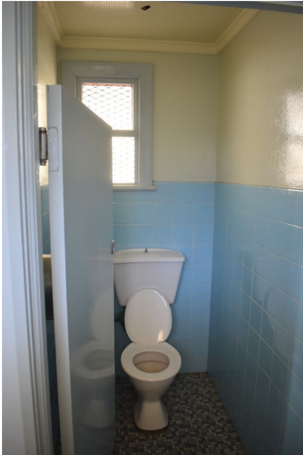
Figure 53. Female toilet cubicle. Wall tiles run just above window sill height.
