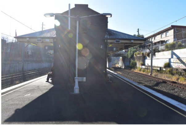
Figure 31. View of west elevation. Brick parapet wall featuring face bricks partially painted mission brown approximately to the top of the awnings on either side. A flush door is located in the centre with two windows above.
