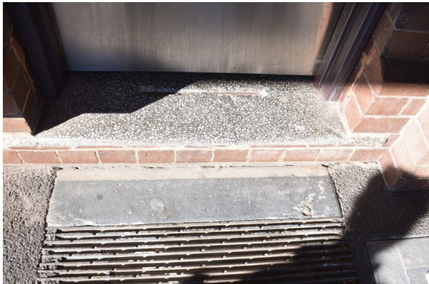
Figure 39. Close up of terrazzo step threshold to the female toilets and boot scraper grill.
