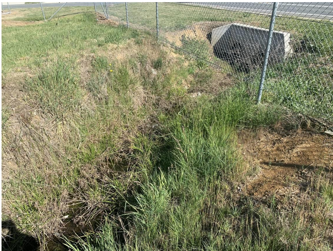
Photo 16: Downgradient of the fourth culvert encountered, coming from the South of the site, near to Malbon Street railroad crossing. Water slowly discharging through site. Low turbidity.
