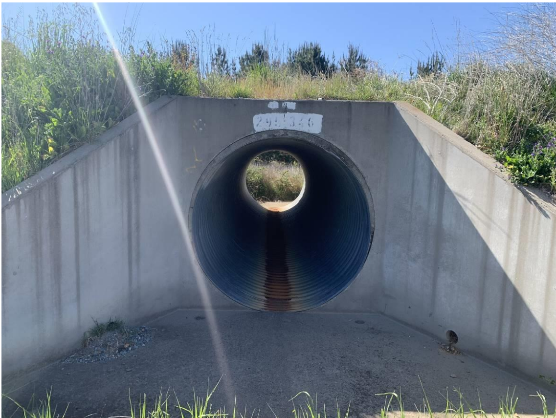
Photo 12: Downgradient of the first culvert encountered, coming from the South of the site. Dry, no surface water present with no visible sediment inside culvert or surrounding area.
