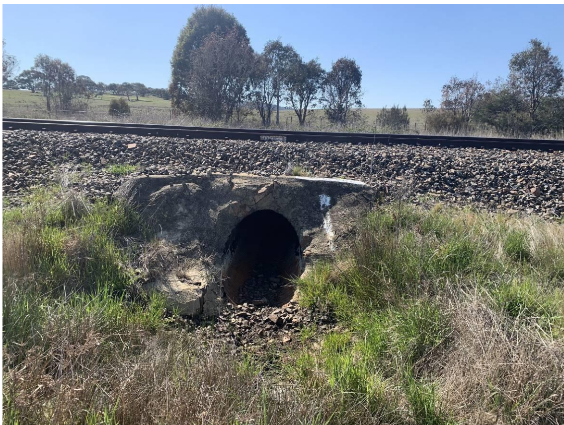
Photo 14: Downgradient of the third culvert encountered, coming from the South of the site. Dry, no surface water present, with no visible sediment inside culvert or surrounding area.
