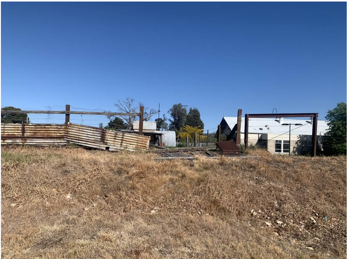
Photo 2: Collapsed fencing adjacent to rail tracks and north of Bungendore station on the side closest to Majara Street. Condition appears unchanged since last site inspection (17/07/23).
