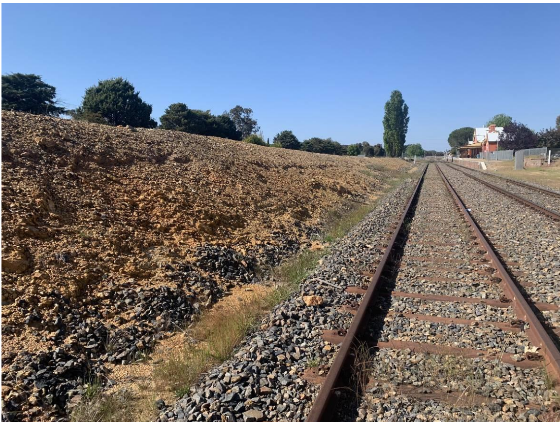
Photo 8: Evidence of erosion upgradient of train line facing south-east towards Powell Street and opposite the Station Master Cottage. Bungendore Railway station to the right.
