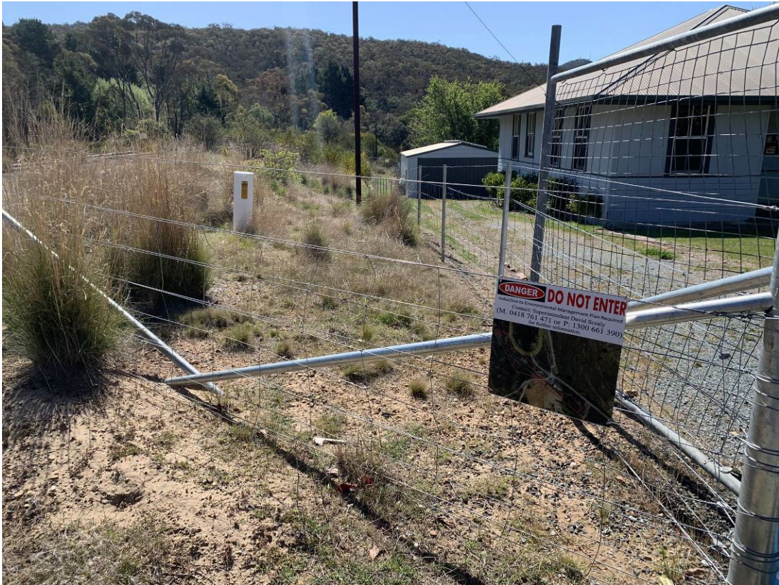
Photo 9: Exclusion zone signage placed at north-East boundary of the site with appropriate fencing.
