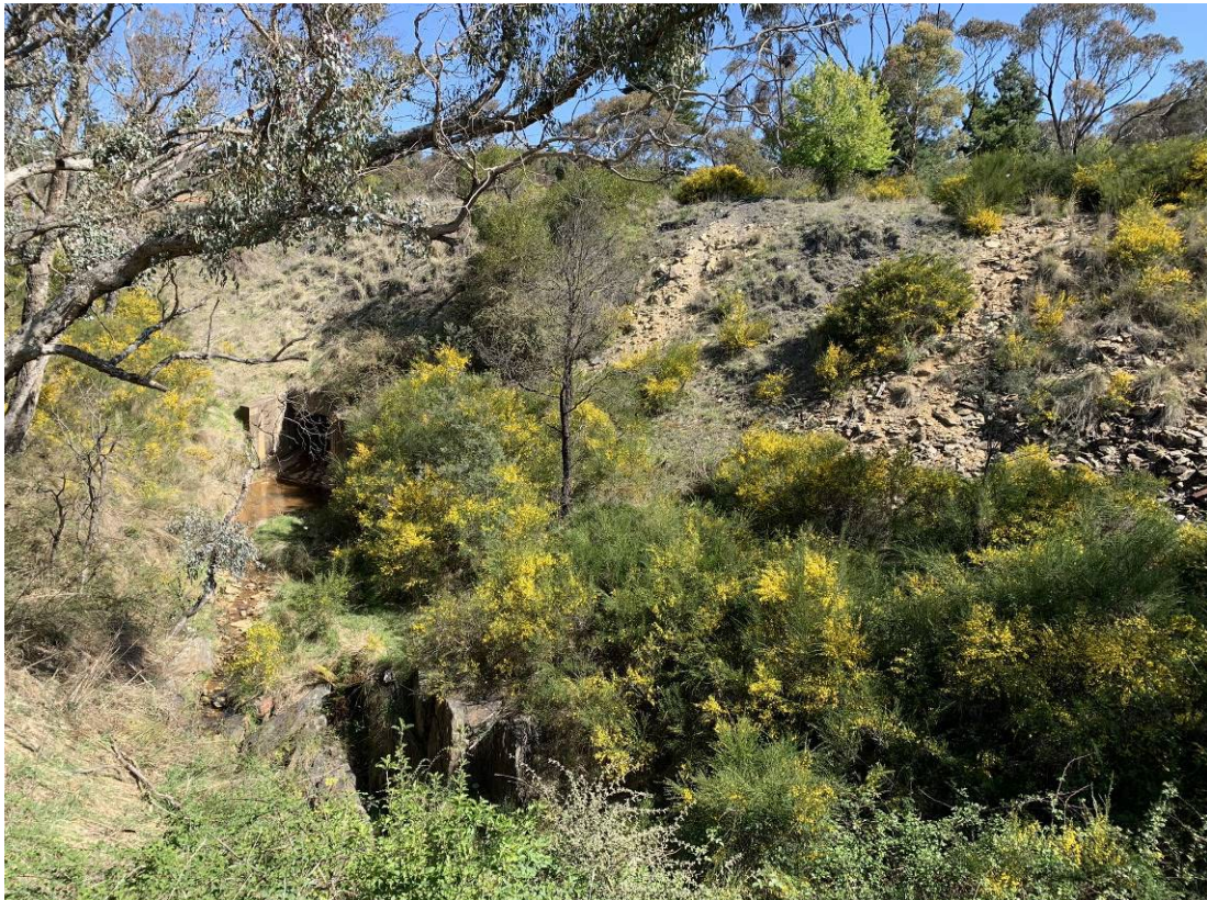
Photo 6: Photo taken from the Miners Road and Captains Flat Road intersection showing the southern boundary of site. Copper Creek culvert visible. No evidence of current onsite surface water runoff into Coppers Creek. Facing South-West.
