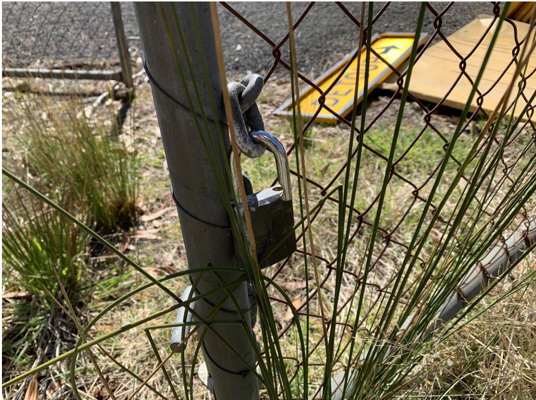
Photo 14: An unlocked and open gate between the site and State Emergency Service (SES) Facility. An unlocked padlock is visible. The opened gate is located on the south-east boundary of the SES facility.
