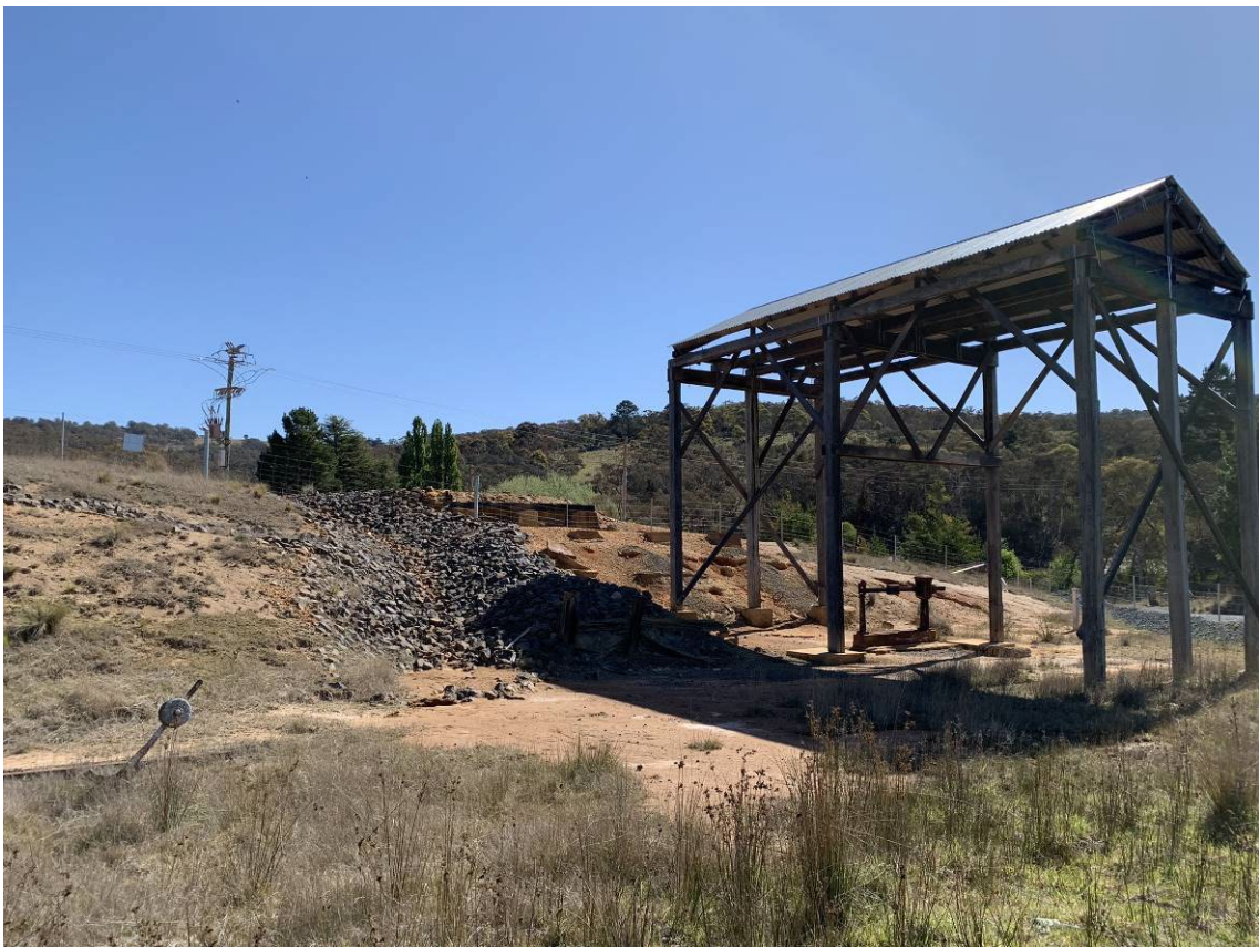
Photo 2: Former Loadout Facility and Weigh Bridge. No airborne dust was visible on site. Facing South-West
