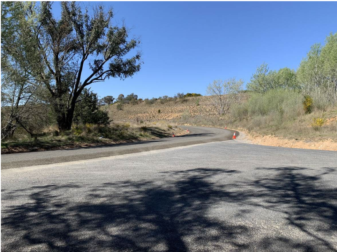
Photo 16: Captains Flat Road and Copper Creek Road intersection. Significant road upgrades and resurfacing have occurred on Captains Flat Road.
