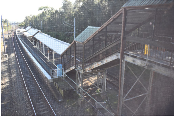
Figure 66. View facing west from the overbridge towards the station. The various canopies connect to run the length the platform from the stairway structure to the platform building.
