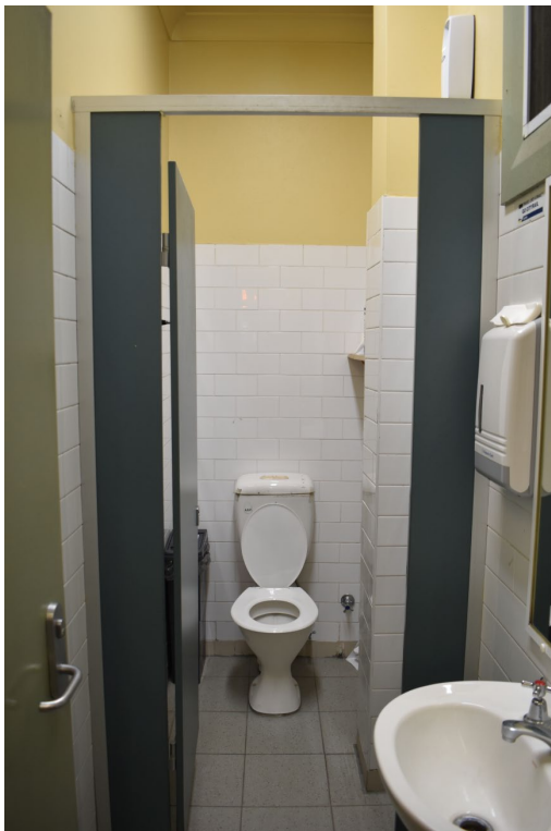
Figure 50. Staff toilet, facing west. A metal frame and timber partition has been inserted for the toilet.
