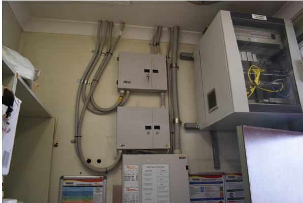
Figure 52. Storeroom. Plant is shown to protrude from the internal wall above the store entry partially concealing the transom window. Exposed pipework is shown to the left connecting to the ceiling.
