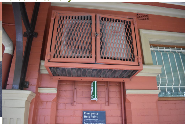
Figure 43. North elevation. Air conditioning unit protruding from the exterior wall concealed within metal hutches.
