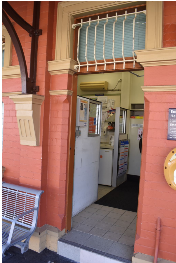
Figure 39. South elevation. Close up of entry to storeroom. Grilles have been installed in front of window openings.
