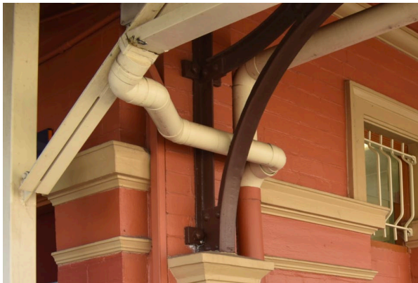
Figure 44. Close up of southwest corner. Standard double bowed steel brackets supporting the canopies have been painted mission brown. Downpipes run across the canopies and are fixed to the north and south elevations.
