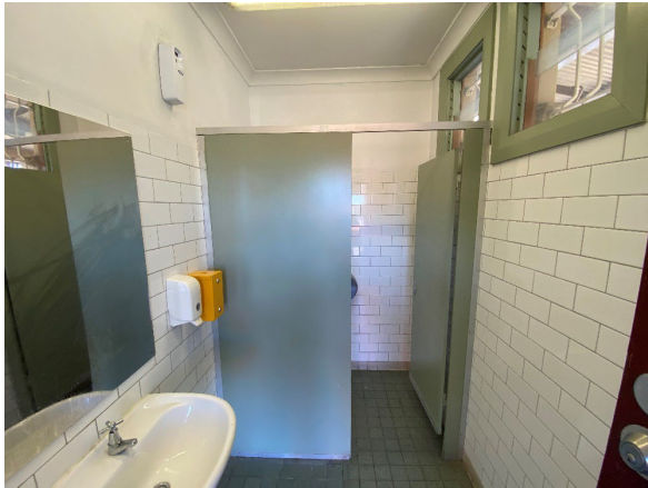
Figure 55. Unisex WC, facing east. Internal walls feature subway tiles to approximately 2m in height. Floor is tiled. A thin metal frame and timber partition has been inserted for the toilet.
