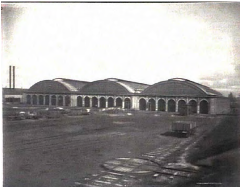
Plate 3.1: The engine running sheds located to the east of the subject site. These sheds were later demolished and replaced by the EMC. (FuturePast, 2015: 15)
