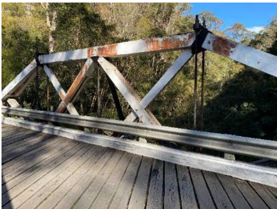
Figure 4-17: View of timber principals and timber trusses, facing south east
