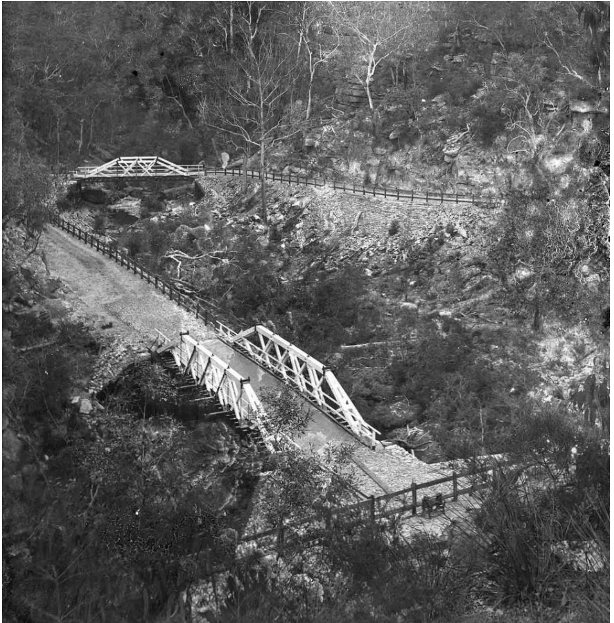
Figure 6-2 Two McDonald Truss bridges at Galston Gorge provided examples of the longest and shortest of the standard McDonald Truss designs, the former Berowra Creek Bridge at 27.4 metres (bottom) and the remaining Galston Timber Bridge (Tunks Creek Bridge) at 19.8m.
