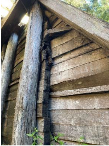
Figure 4-25: Example of timber displacement where previously replaced in wings of North Abutment (B)
