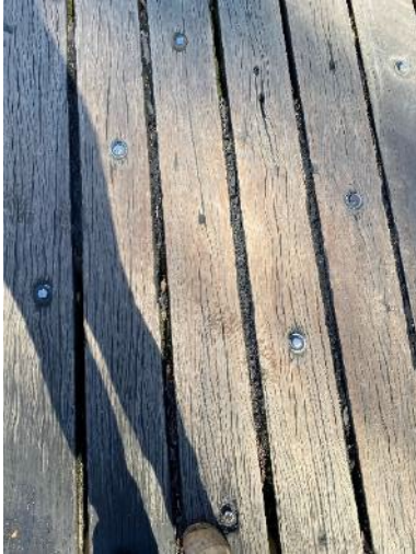
Figure 4-15: Another view of the transverse timber decking including spacing
