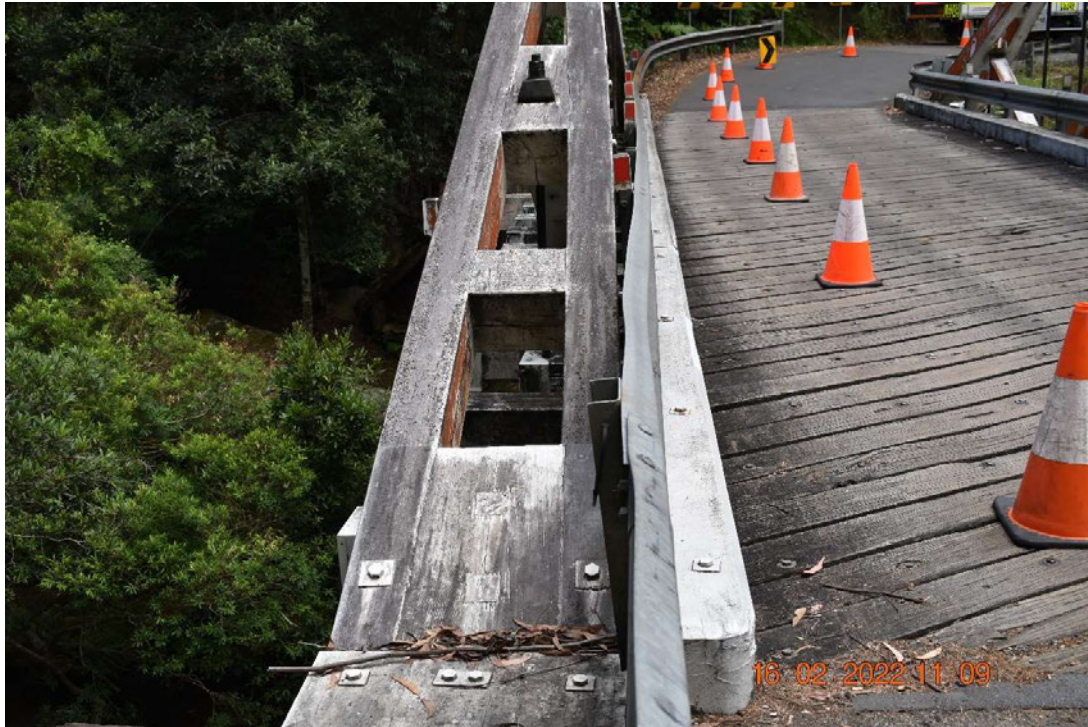
Picture 26 Mould on white painted timbers
