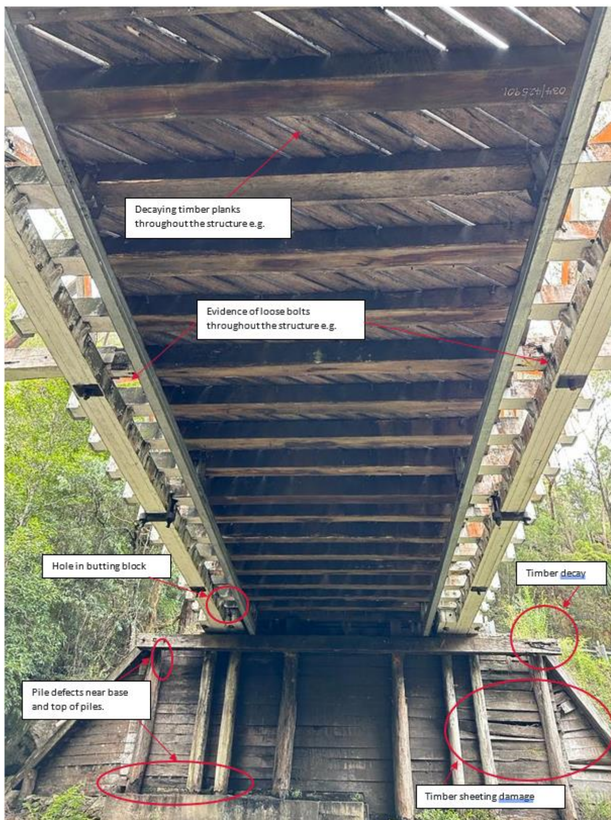
Examples of key defects to be repaired or elements replaced
