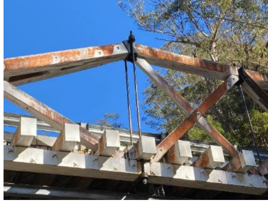
Figure 4-8: View of the principal timbers and trusses, and steel tie rods, facing south west
