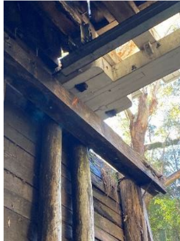
Figure 4-20 View of butting timber block to be replace, on western side of bridge attached to North Abutment (B)
