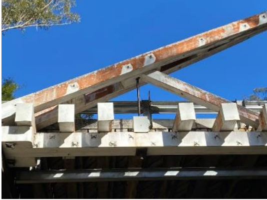
Figure 4-9: View of the principal timbers and trusses, and steel tie rods, facing south west
