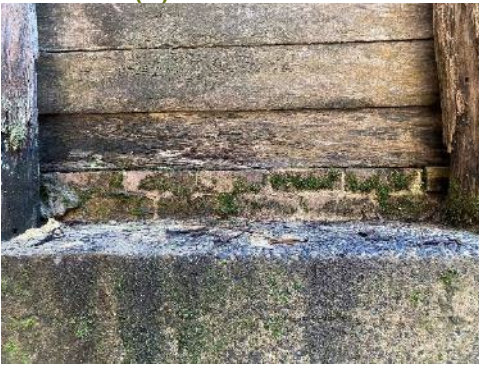
Figure 4-27: Example of concrete casing below piles with brick retaining under the timber sheeting of North Abutment (B)
