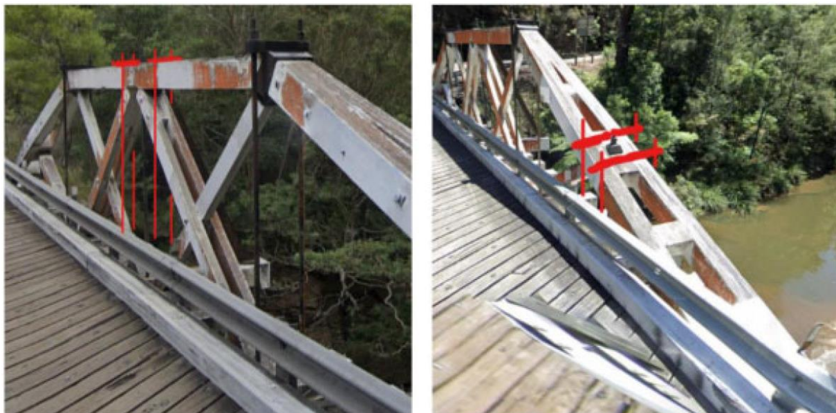
Figure 3-9 Temporary hanger bracket locations (Source: Contractor Works Methodology (August 2024))
