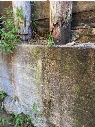
Figure 4-29: Example view of concrete casing experiencing cracking directly beneath each pile
