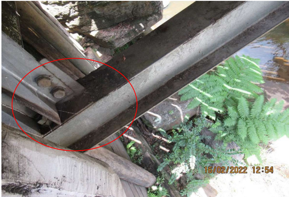
Picture 29 General corrosion on I beams and bolts
