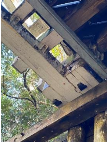
Figure 4-19: View of butting timber block to be repaired, on eastern side of bridge attached to North Abutment (B)
