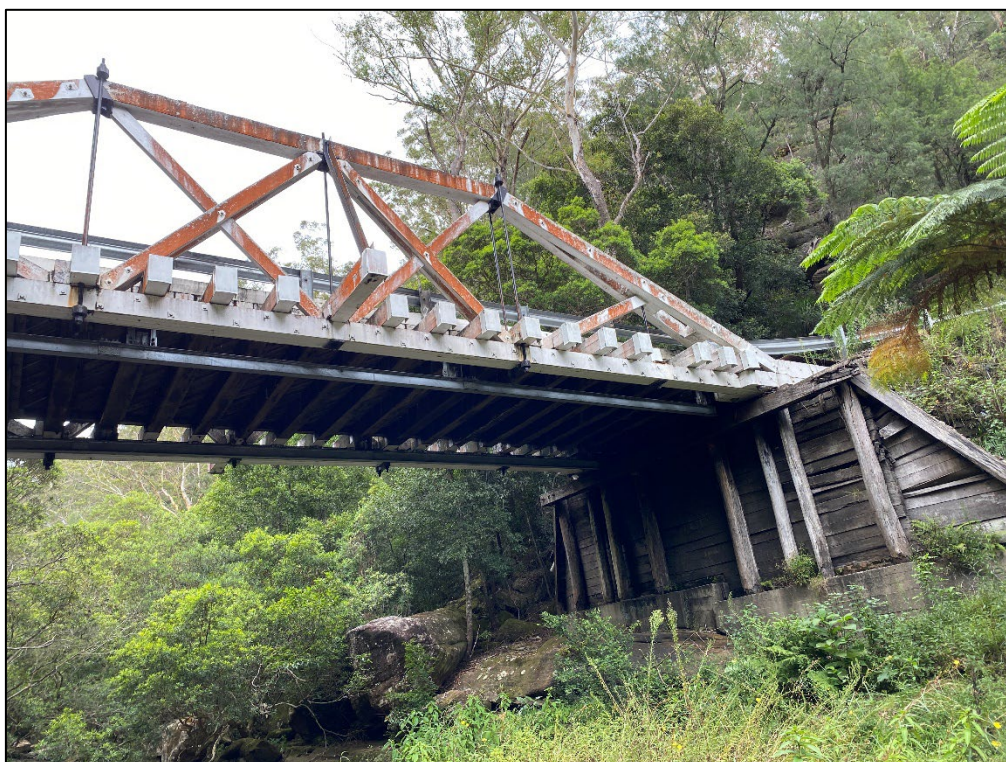
Plate 2: Structure of the northern abutment and bridge underside.
