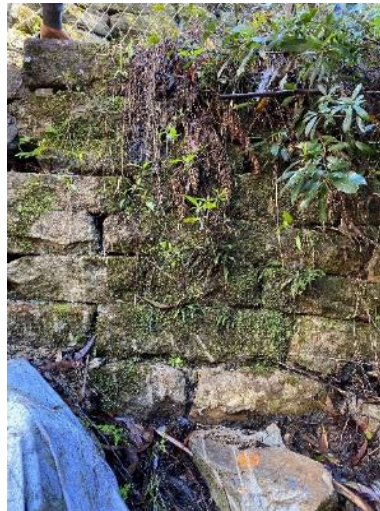
Figure 4-30: Example view of dry stone walls on either side of the abutments of the bridge
