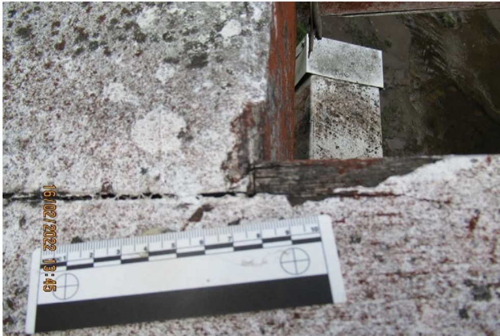
Picture 37 Paint Delamination
