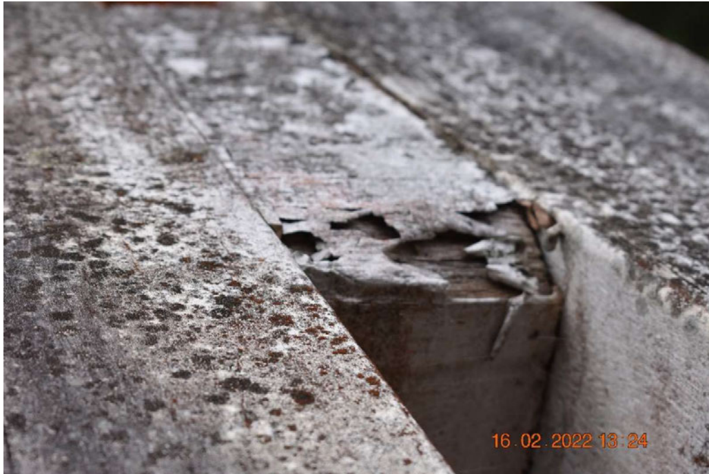
Picture 30 – Timber Rot and Paint delamination
