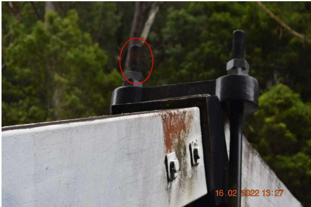
Picture 36 Corrosion on black metal pole
