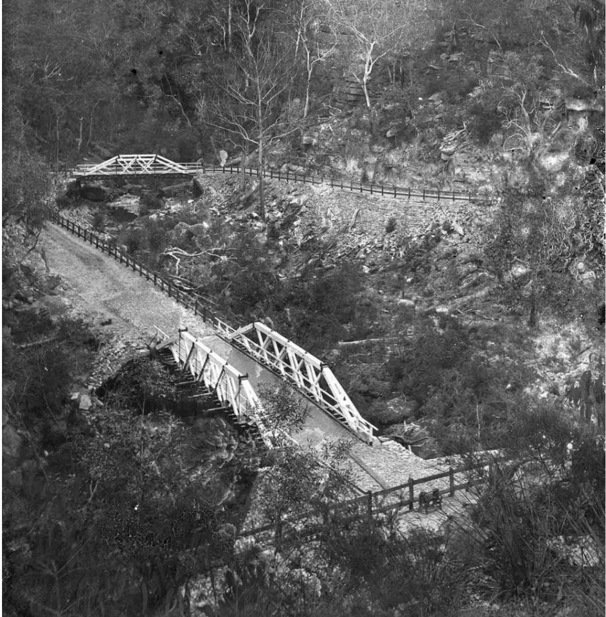
Figure 3-5: Two McDonald Truss bridges at Galston Gorge provided examples of the longest and shortest of the standard McDonald Truss designs, the former Berowra Creek Bridge at 90 feet (bottom) and the remaining Galston Timber Bridge (Tunks Creek Bridge) at 65 feet (27.4 m and 19.8m). (Source: WF Hall photo, Australian National Maritime Museum. Retrieved from: Timber Truss Book)
