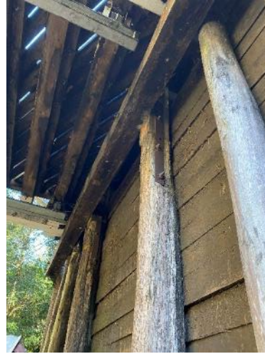
Figure 4-26: Closer view of spliced piles, top section of two piles in foreground of North Abutment (B)
