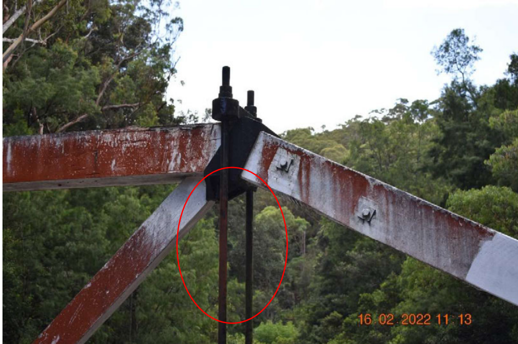
Picture 35 Corrosion on black metal poles
