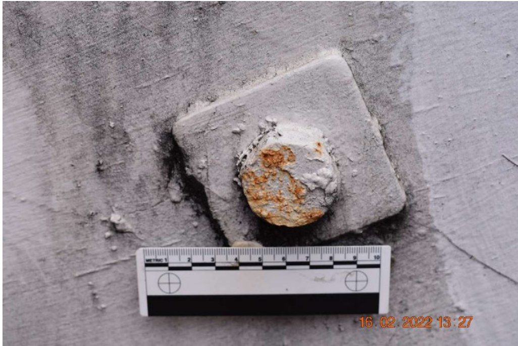
Picture 27 General corrosion on bolt
