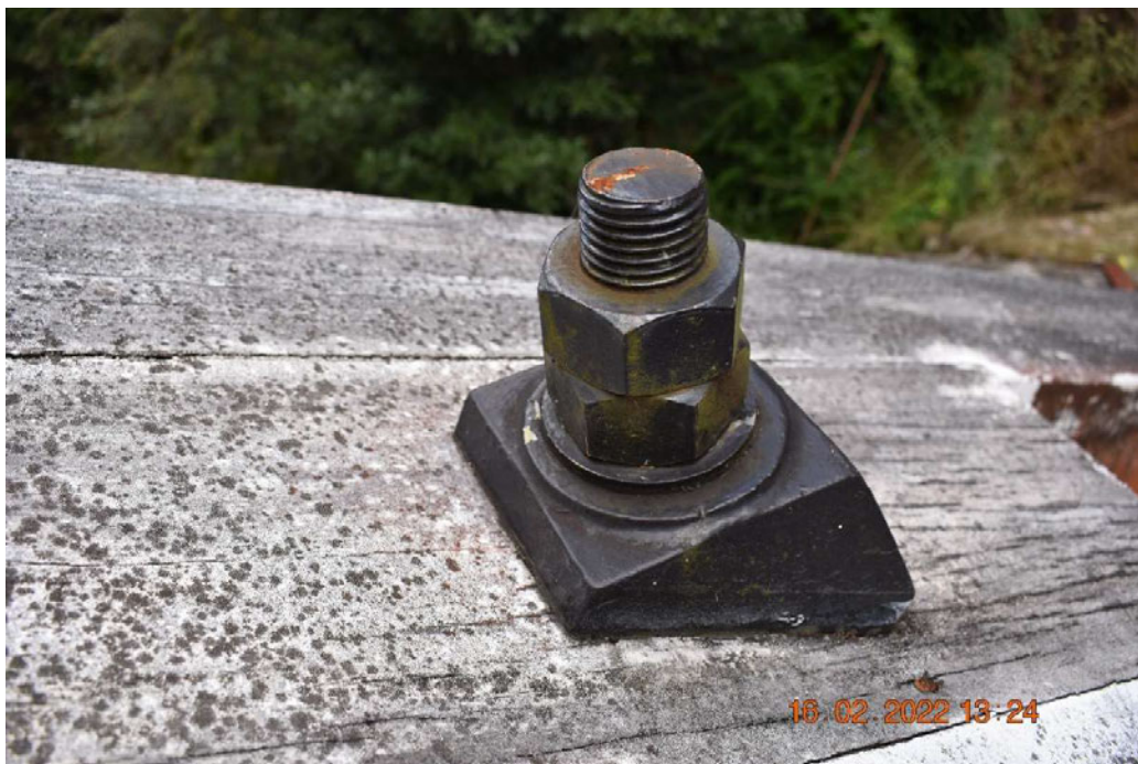
Picture 28 General corrosion on bolt
