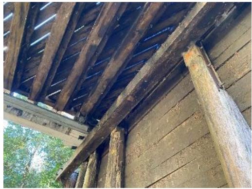
Figure 4-24: Example of spliced piles, top section of two piles in foreground of North Abutment (B)
