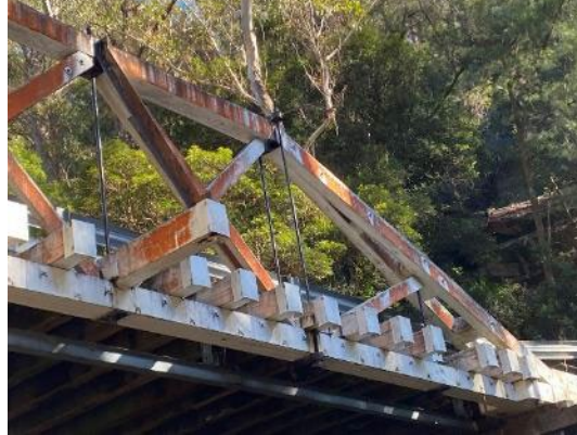
Figure 4-10: View of the principal timbers and trusses, and steel tie rods, facing south west
