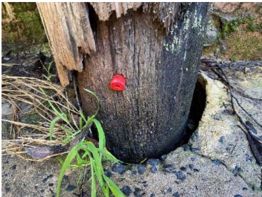
Figure 4-23: Example of pile encased in concrete, experiencing timber rot
