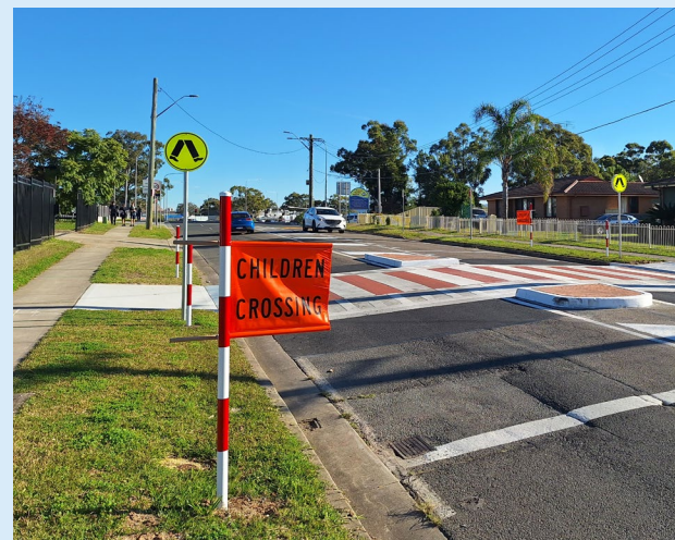
Raised crossing on Bringelly Road. Delivered by Penrith City Council and co-funded by Get NSW Active. Image courtesy of Penrith City Council.
