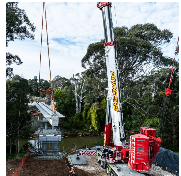
Lifting in one of six 46-tonne girders into place at Constitution Hill for the T-way cycleway Realignment project. When completed, the 75-metre bridge will provide a safe link for pedestrians and bike riders. Delivered by City of Parramatta Council and co-funded by Get NSW Active. Image courtesy of Abergeldie Complex Infrastructure.
