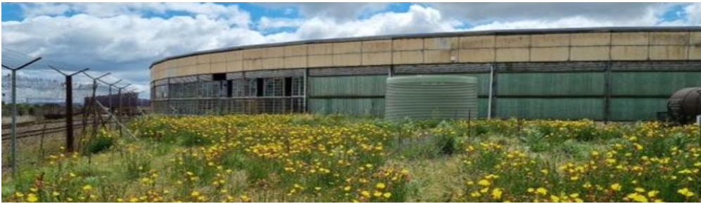
Roundhouse looking north.
