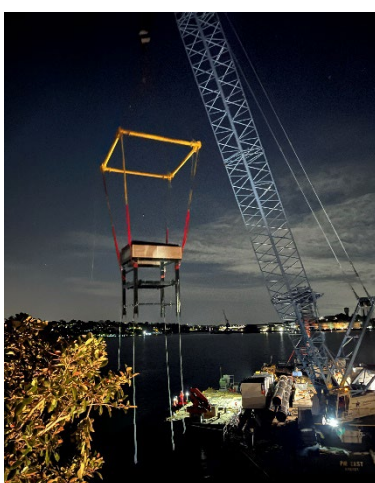
View of the lift shaft being installed at night
