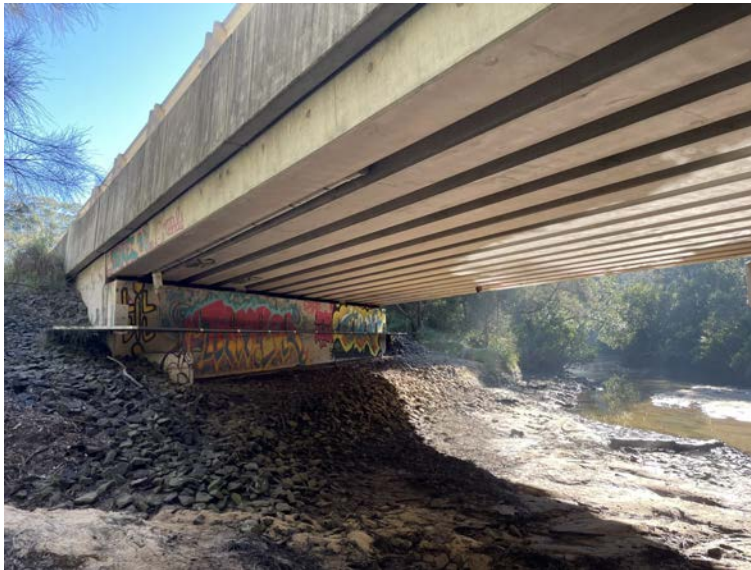
Figure 3-8: Raised ledge installed at northern abutment of Deadmans Creek bridge. Ground treatments would be applied to each end of this ledge to improve fauna access across the riprap
