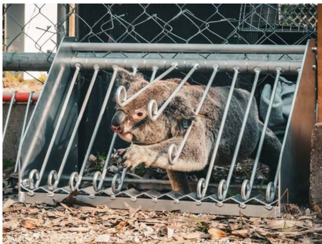
Figure 3-11: Example of one-way koala escape hatch
