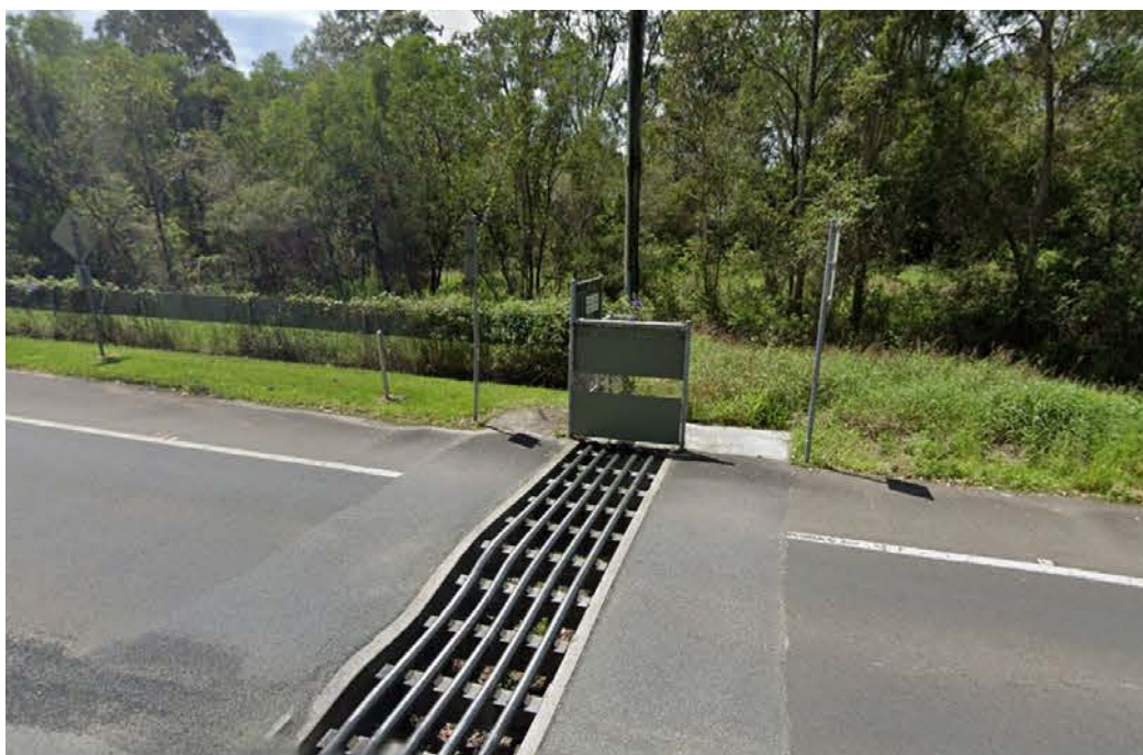
Figure 3-6: Koala grid installed on Gulgan Road, Brunswick Heads, with koala fencing alongside the road
