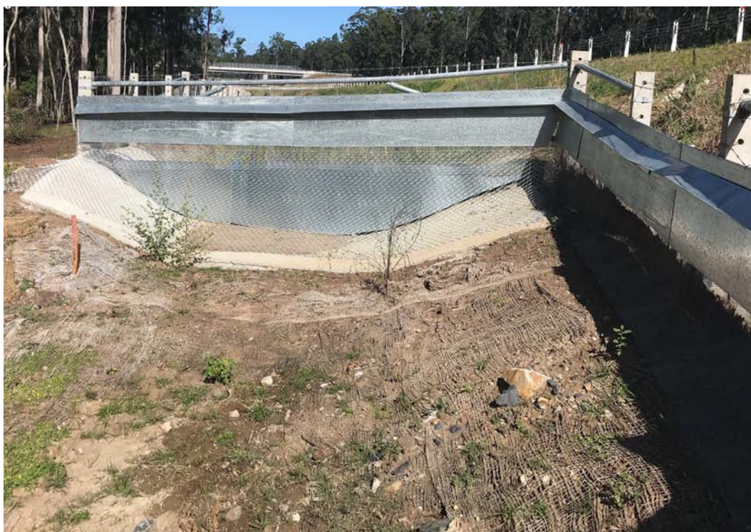
Figure 3-3: Example drainage flap where koala fence traverses a drainage swale
