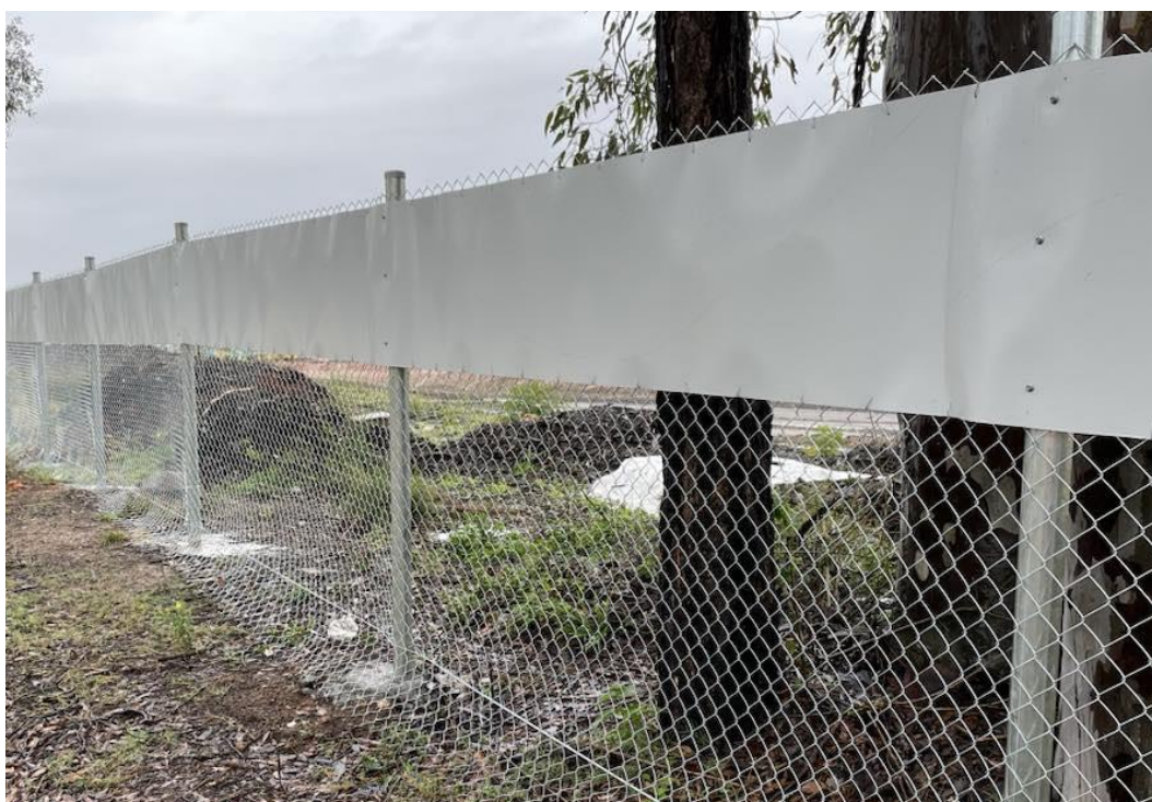
Figure 3-4: Example of koala fencing installed alongside the M1 to Raymond Terrace project in the Hunter Region
