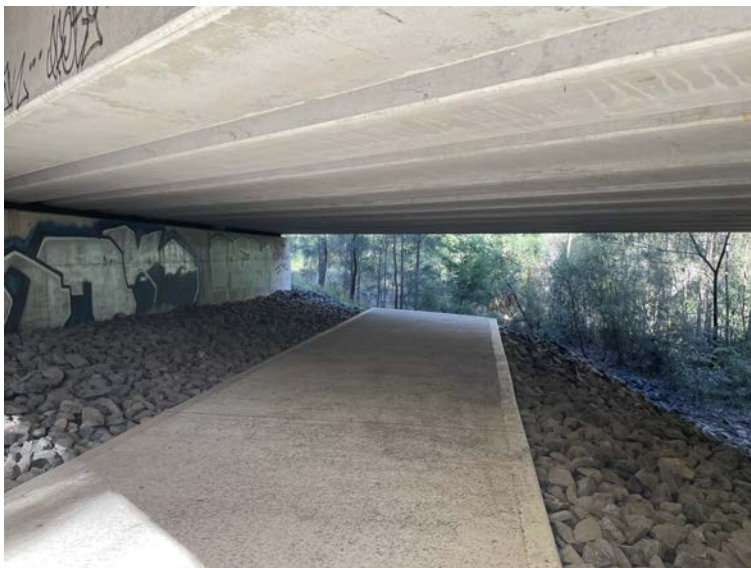
Figure 3-9: Concrete pathway installed at the southern bridge abutment
