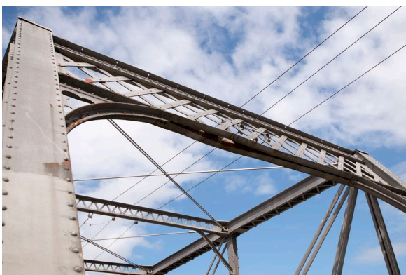
Image: End truss lattices
