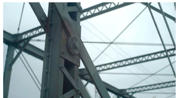
Images: rosette style diagonal bracing washers
