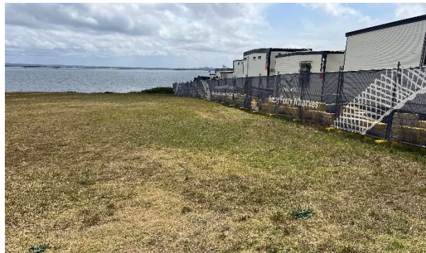
Photo LP6: La Perouse Site compound – Fence line located by survey within the Project Boundary. Shallow soil upon rock shelf has been undisturbed due to proximity to AHIMS Site# 45-6-0651 (Site 4 - La Perouse).
