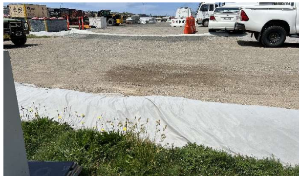
Photo LP7a and LP7b: La Perouse site compound – Entire site compound lined with geofabric and road base to prevent disturbance of AHIMS Site# 45-6-0650 (Site 3 - La Perouse). No dig order is in place.
