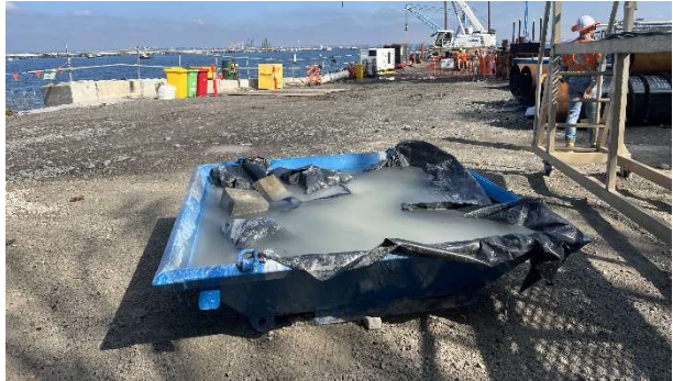
Photo K7: Kurnell construction site. Containment of concrete agitator washout waste.
