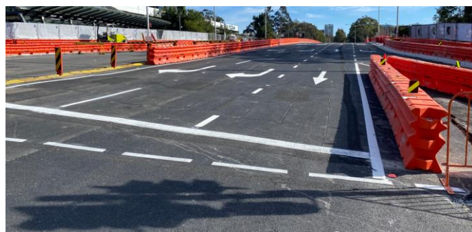
Completed temporary line marking along Waterloo Road
