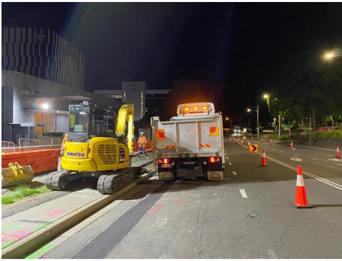
Footpath preparation works along Waterloo Road
