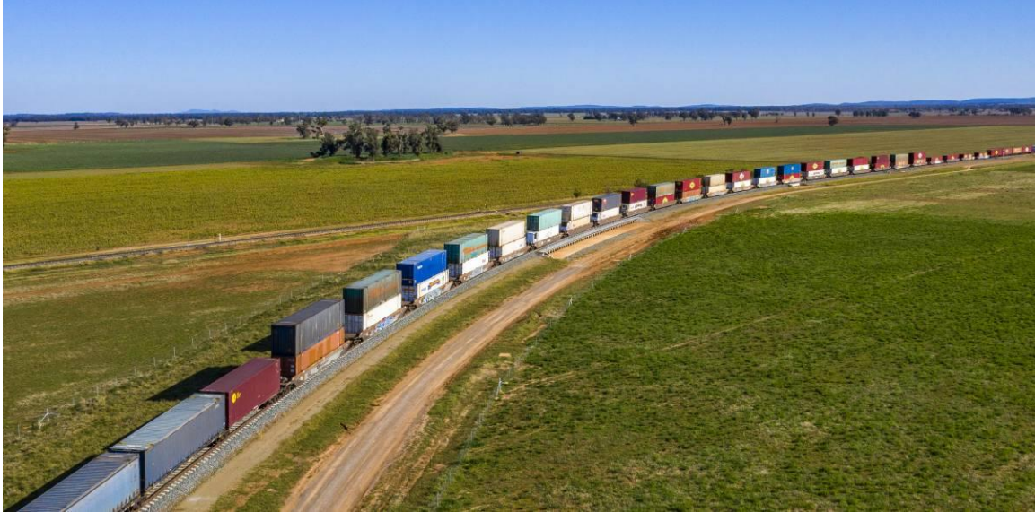
Figure 19: A double-stacked freight train at on the upgraded Inland Rail line at Parkes. Picture: ARTC
