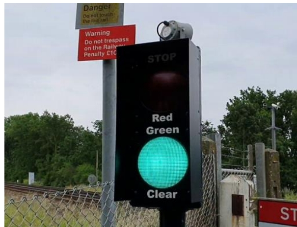
Figure 12: Typical Vamos level crossing signalling components for a private level crossing.
