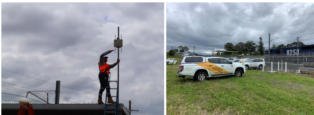
Figure 11: The DSRC Roadside Unit being installed at Unanderra Level Crossing.
